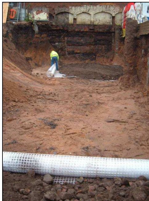
Plate 15: General working shot in north-east corner facing north
