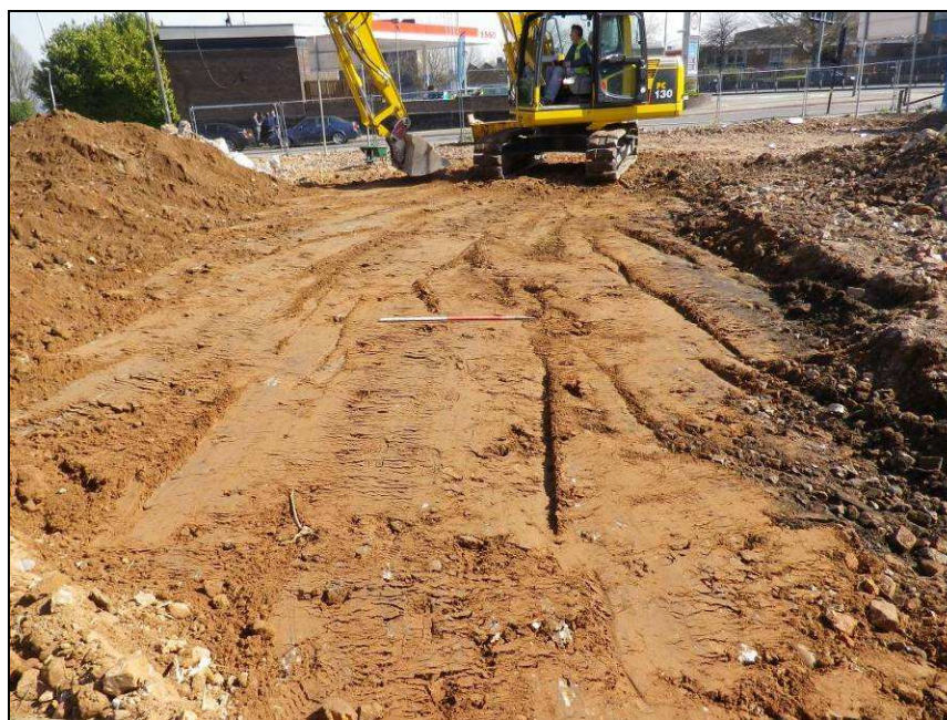
Plate 2: East facing photo of site being stripped of (1000) to reveal (1002)
