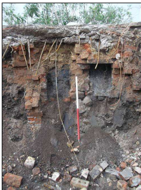
Plate 10: Shot of furnace {1018} and burnt material (1023) next to west wall in north-west corner
