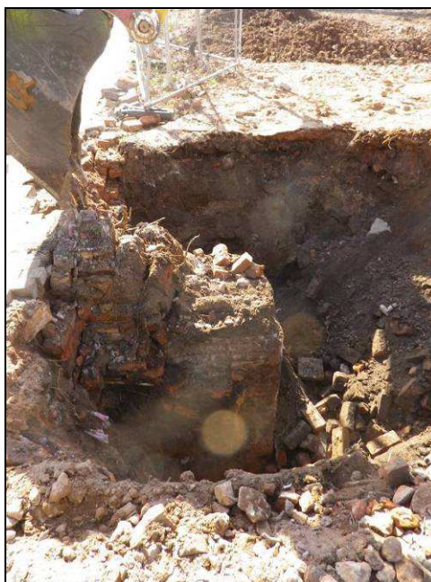
Plate 1: South facing photo of Stanchion 2 {1001} being excavated
