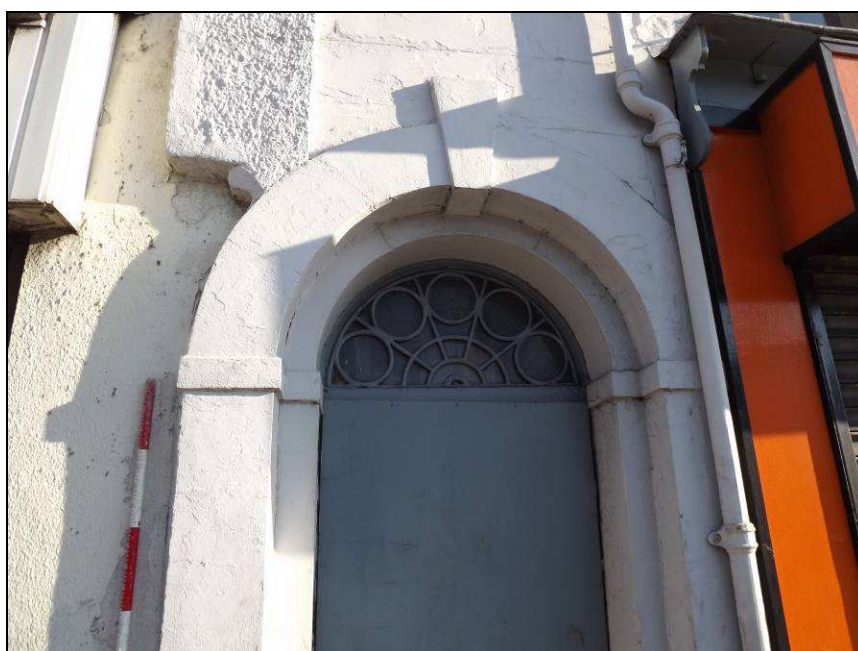
Plate 62: Detail of arched head and decorative fanlight window, 155 Botchergate
