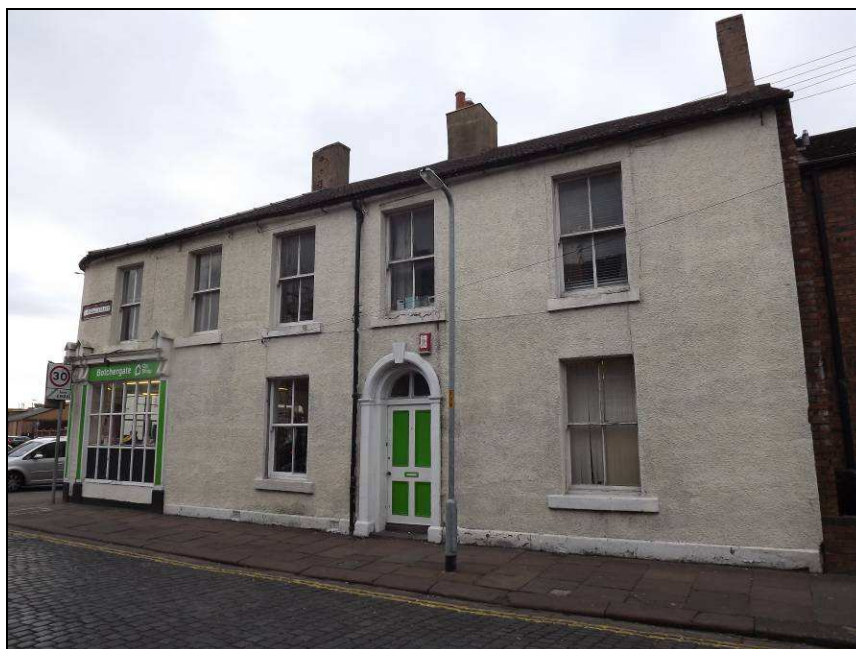
Plate 70: No.159 Botchergate and No. 1 Rydal Street as seen from the south side of Rydal Street
