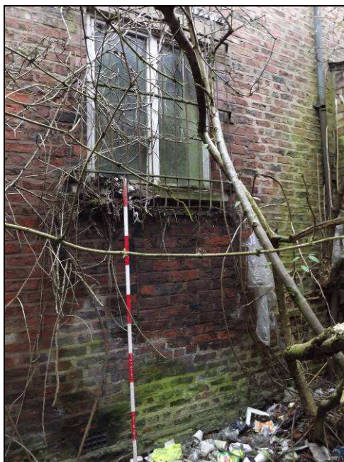
Plate 27: Detail of blocked window, south-east elevation of No. 1 South Henry Street
