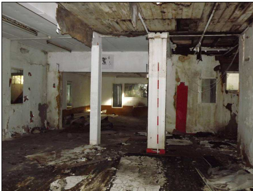
Plate 44: View looking north-east showing the ground floor space of No. 149 Botchergate
