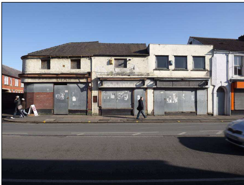
Plate 57: No's 149 to 153 Botchergate
