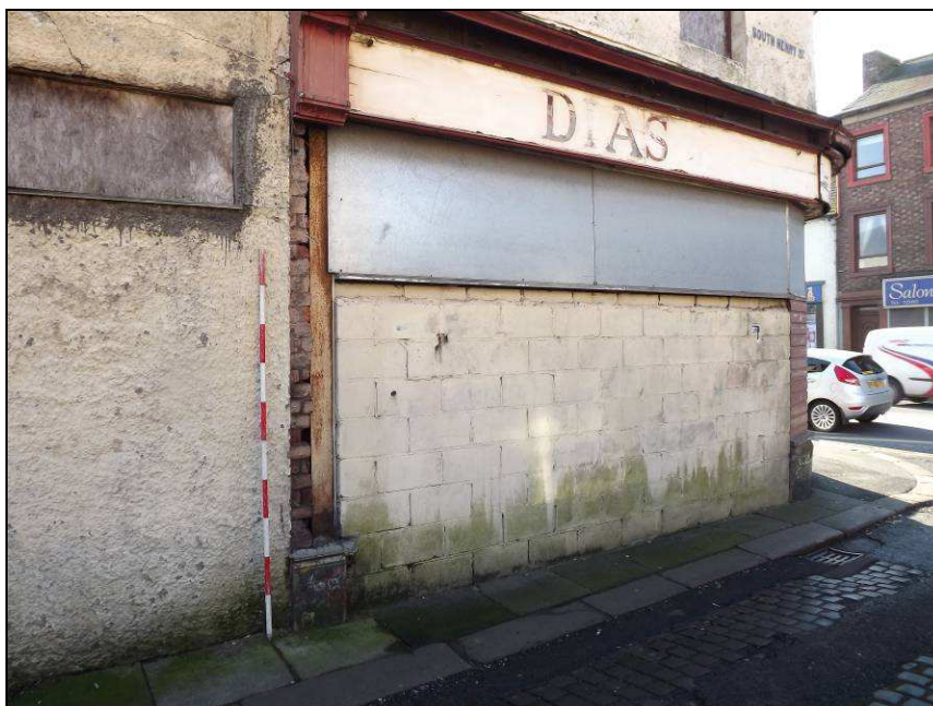
Plate 36: Detail of infilled shop front on South Henry Street, part of No. 149 Botchergate
