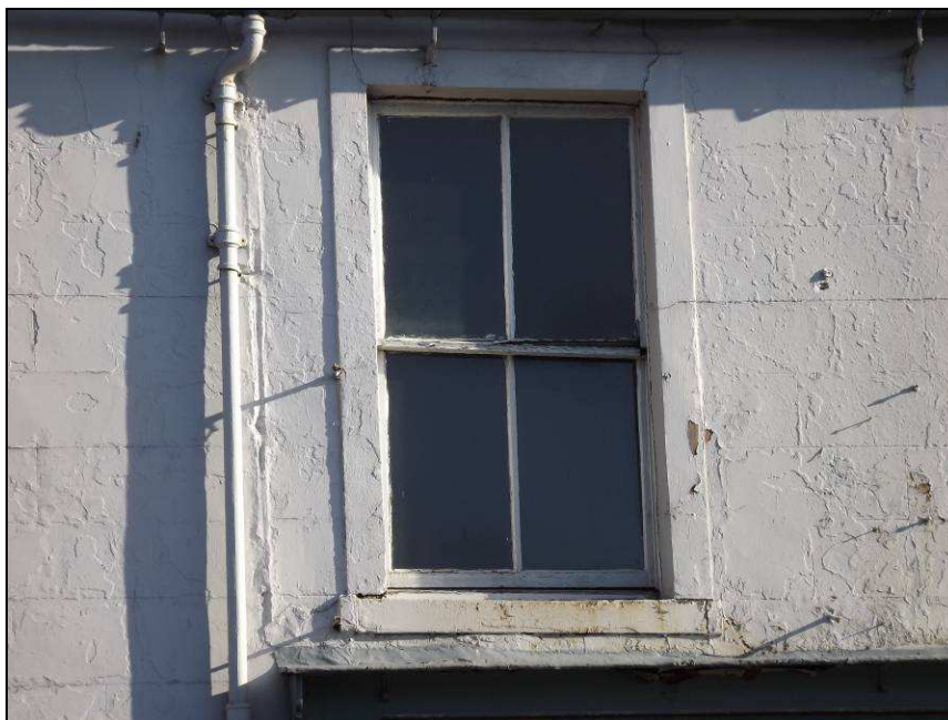
Plate 63: Detail of first floor window, No. 155 Botchergate
