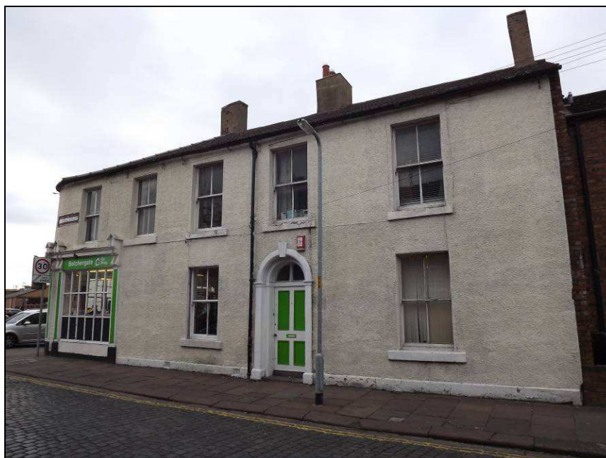
Plate 70: No.159 Botchergate and No. 1 Rydal Street as seen from the south side of Rydal Street
