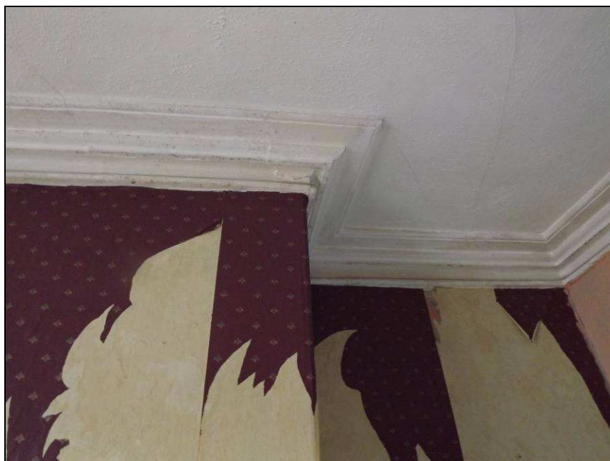
Plate 66: Detail of coving, first floor of No. 155 Botchergate
