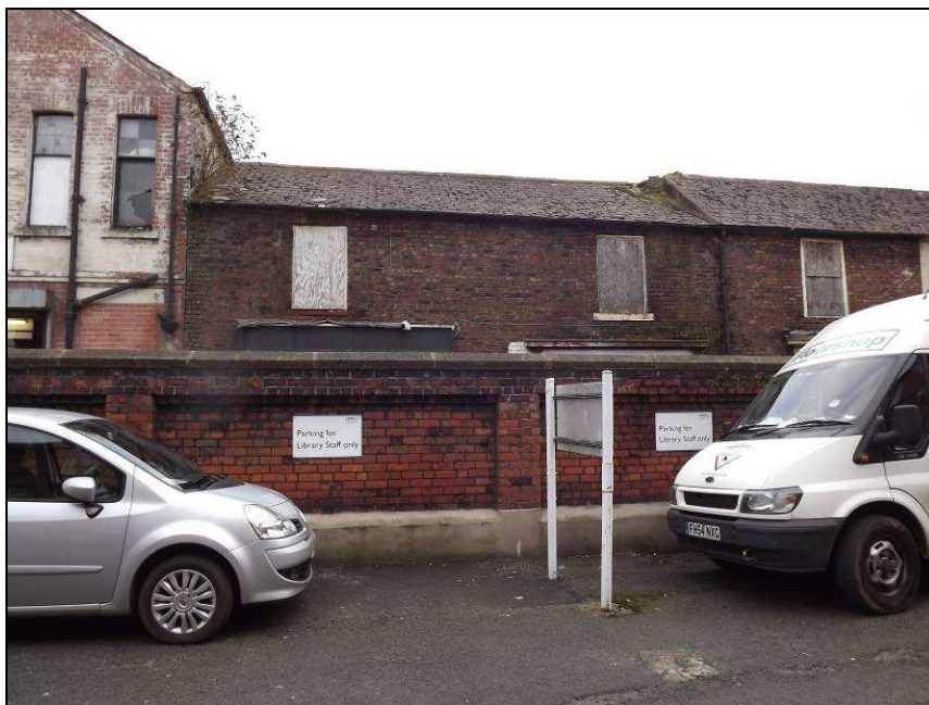
Plate 17: No's 2 and 3 South Henry Street as seen from the north-west (from the car park of the Library Services)
