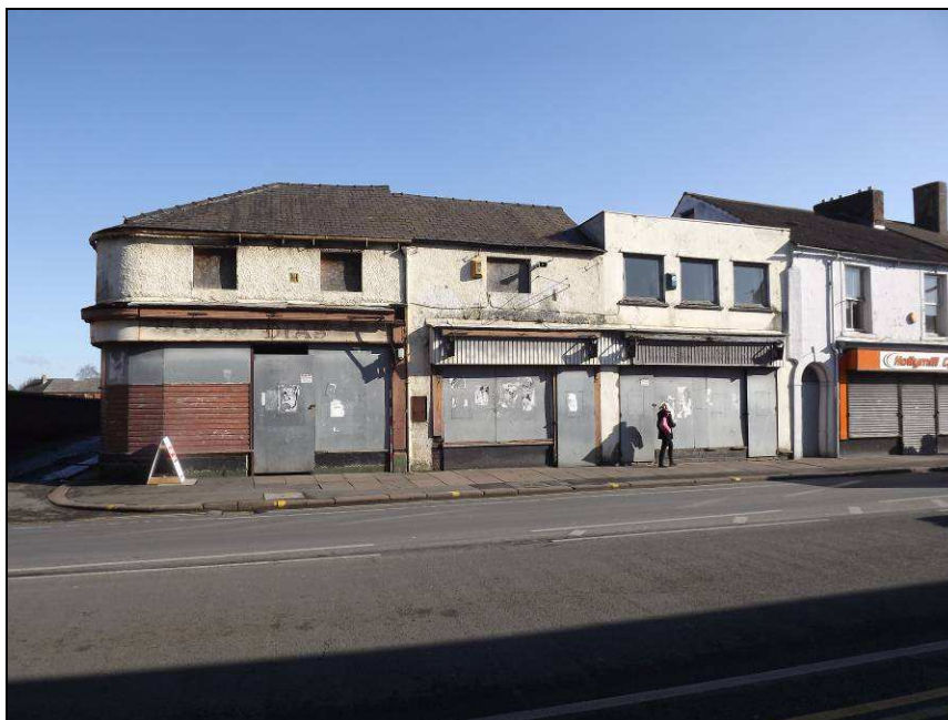
Plate 33: South-west elevation of 149-153 Botchergate showing differing roof lines
