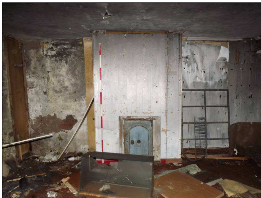
Plate 28: Former fireplace with inserted safe, north-east wall of No. 1 South Henry Street
