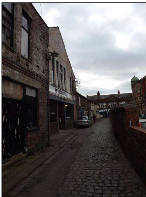
Plate 14: View looking west towards Botchergate showing South Henry Street
