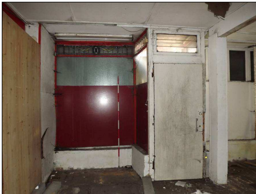
Plate 42: Detail of surviving shop window decoration, interior of No. 149 Botchergate
