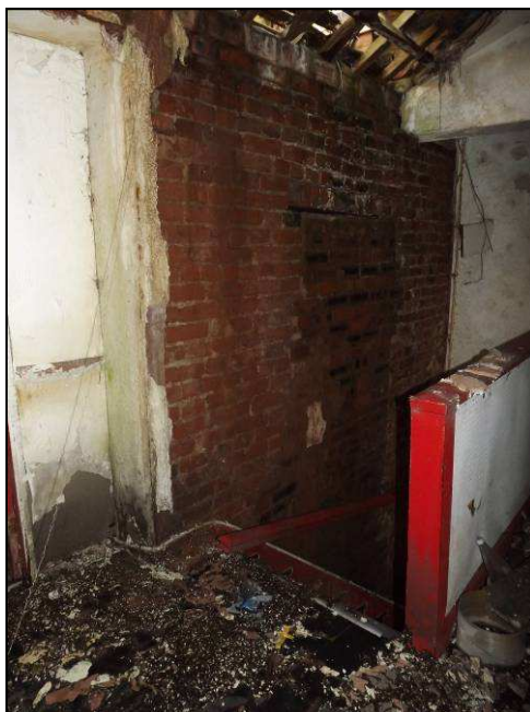
Plate 45: Detail of blocked window, first floor level, north-east wall of No. 151
