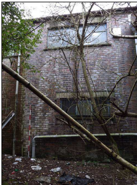
Plate 40: Modern flat-roofed addition to the rear (north-east side) of 149-151 Botchergate
