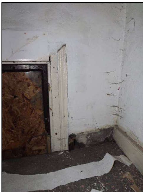
Plate 67: Detail of landing between first and second floors set across a first floor window, No. 155 Botchergate
