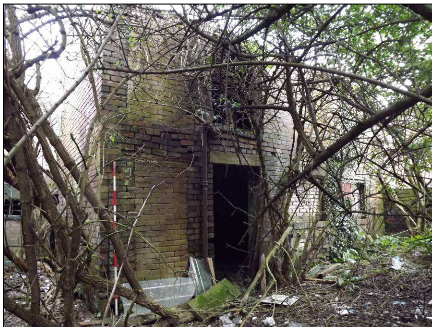
Plate 73: Building in yard to rear of Botchergate frontage
