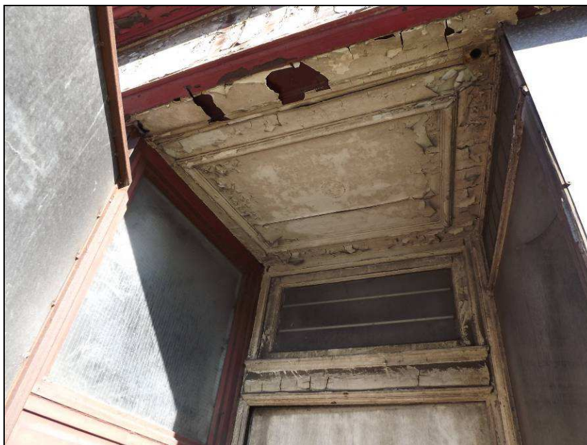
Plate 39: Detail of recessed doorway, No. 149 Botchergate
