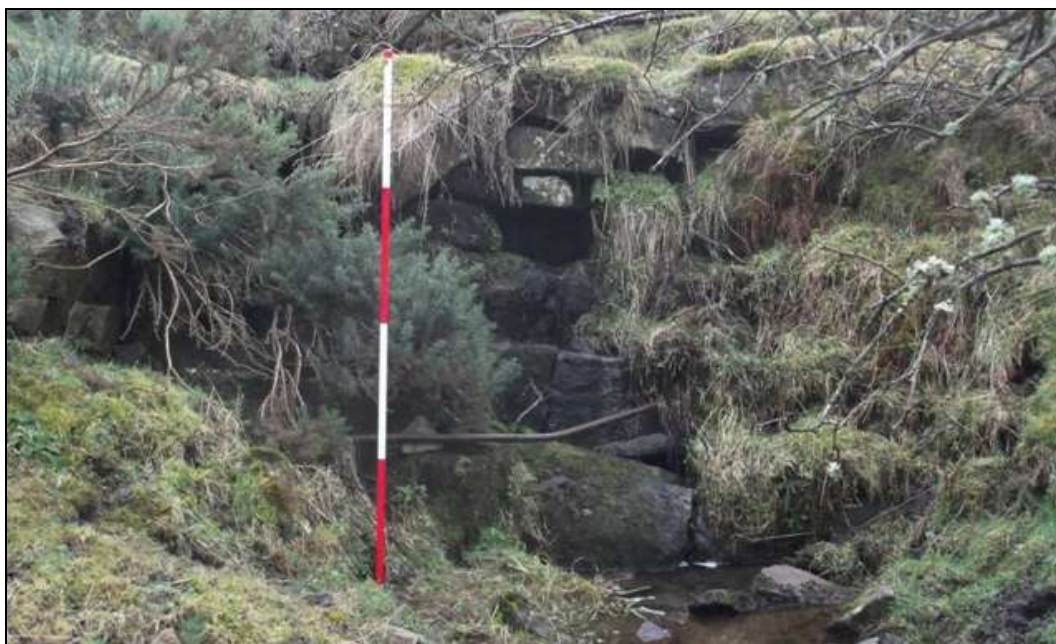
Plate 13: Site 40 Revetment Wall, facing south, scale 2m
