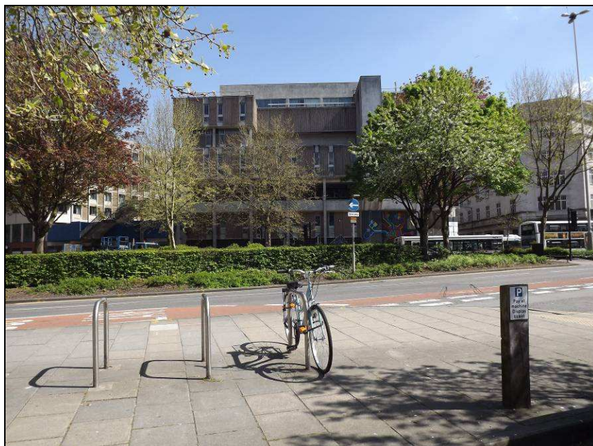
Plate 2: View looking south-east from the north side of Rupert Street
