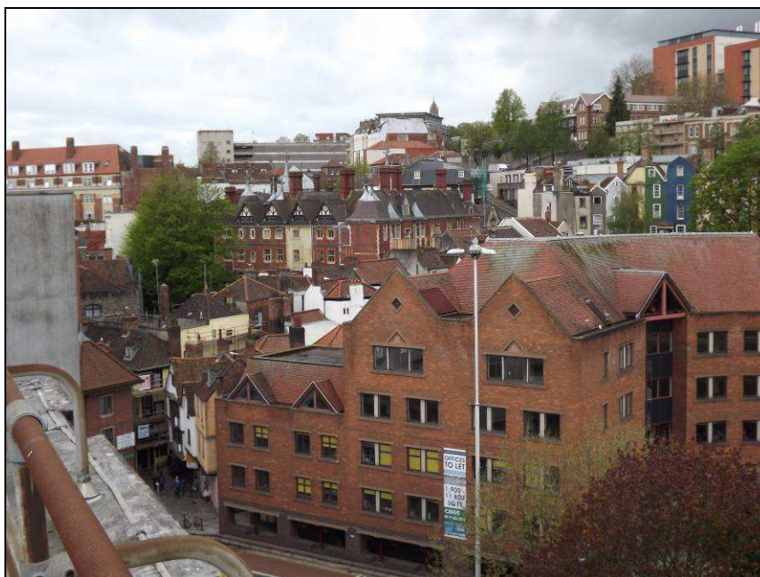
Plate 70: View looking north-west from the roof showing modern offices (Bartholomew's Court) on Rupert Street in foreground
