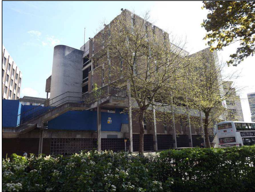
Plate 1: View looking south-west from the north side of Rupert Street
