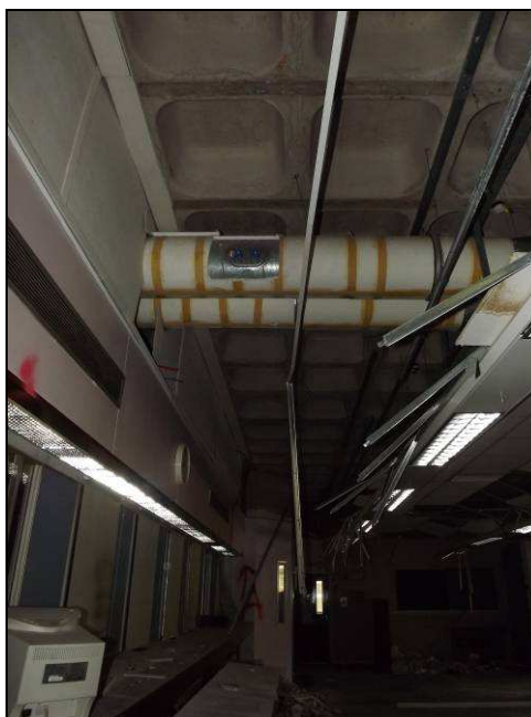
Plate 30: Detail of first floor ceiling
