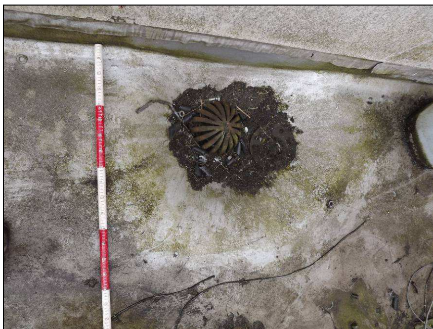
Plate 67: Detail of drainage hole, floor of roof level
