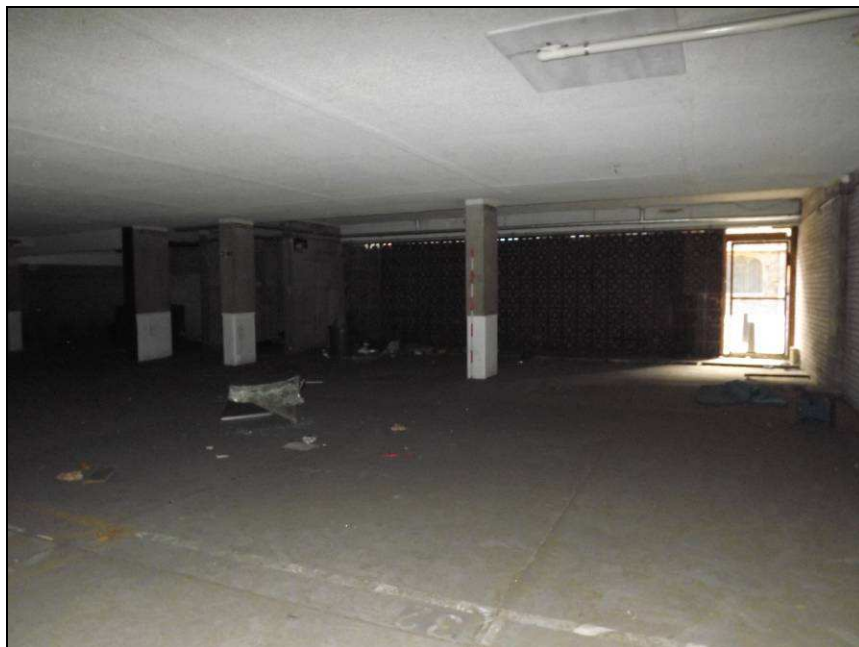
Plate 22: Ground floor car parking area
