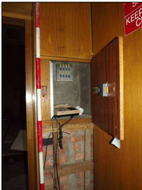
Plate 42: Detail of cupboard, lobby of Court 1, Third Floor
