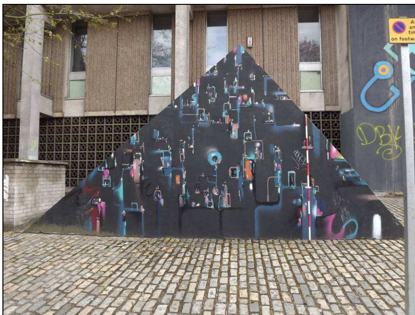
Plate 14: North-west side of substation access point, north-west side of Magistrates Court
