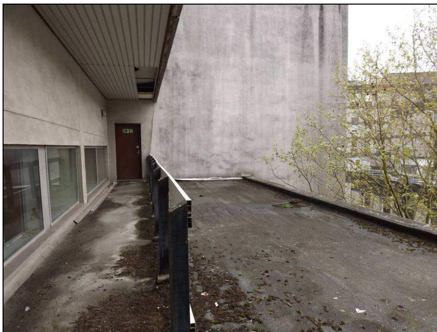
Plate 55: Mezzanine level, Fourth Floor
