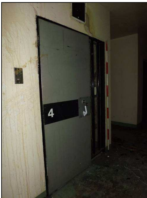
Plate 25: Detail of one of the cell doors, basement
