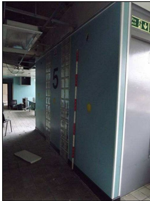
Plate 59: Partition wall between foyer and public stairwell, Fifth Floor
