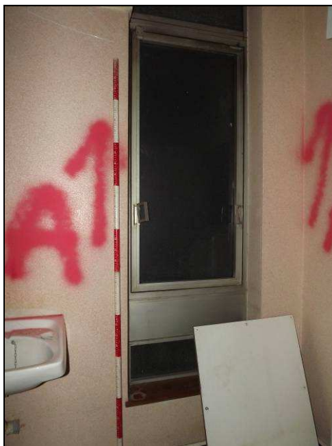
Plate 57: Detail of aluminium window, Fourth Floor
