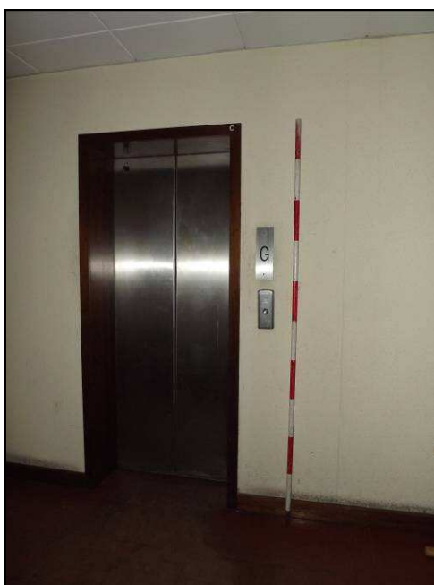
Plate 23: Detail of one of the lifts, ground floor (Scale = 2m)
