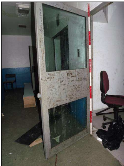
Plate 26: Detail of graffiti, interview room door in basement
