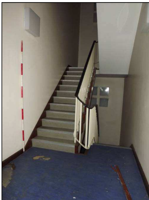
Plate 35: Example of staff staircase (Fourth Floor)
