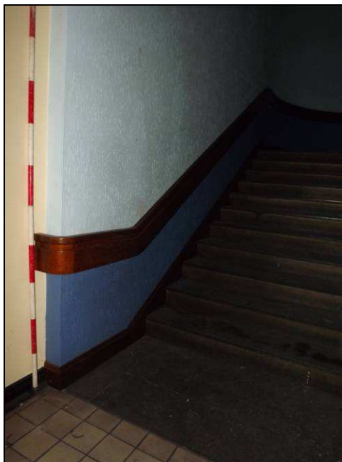
Plate 32: Example of part of one of the public staircases
