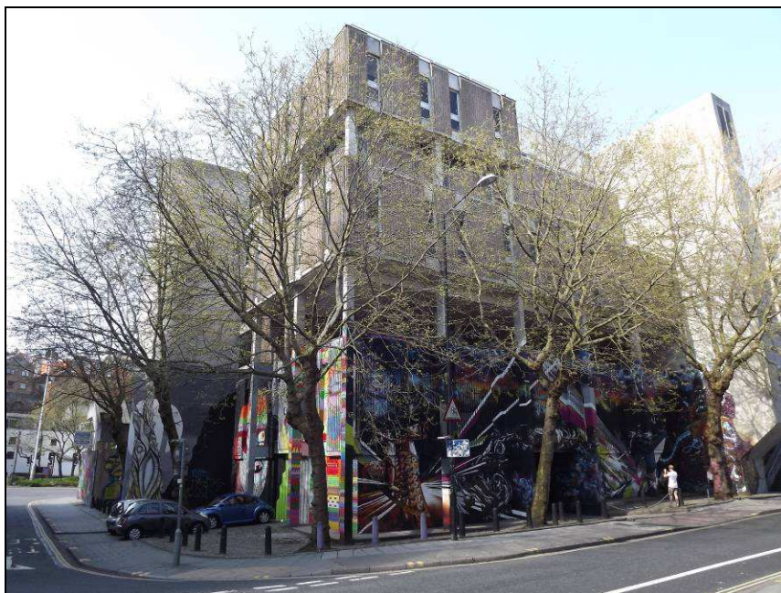
Plate 5: View looking north from the south side of Nelson Street
