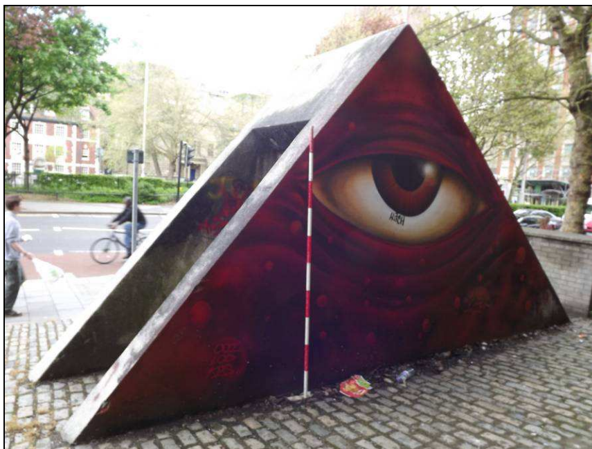
Plate 13: Detail of street art, substation access point, north-west elevation (Scale = 2m)
