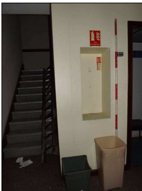
Plate 53: Recess for fire extinguisher, Third Floor
