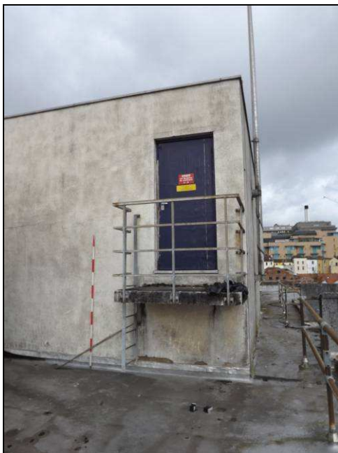
Plate 66: Roof level showing plant room for lift machinery
