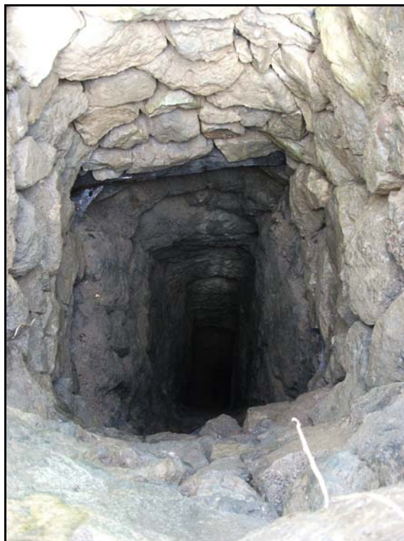
Plate 16: Feature 15 (Shaft 7) showing wooden beam supporting ginging, facing north
