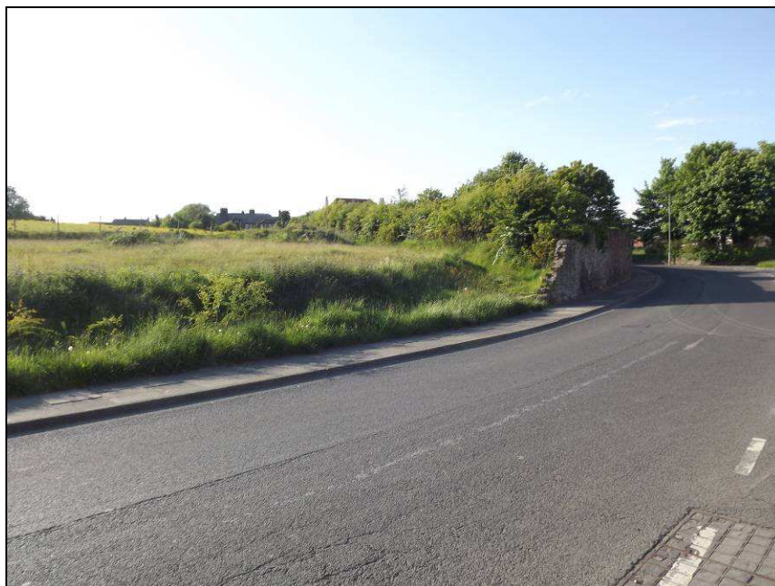
Plate 2: View looking north-east showing the southern portion of the proposed development area with removed section of stone wall
