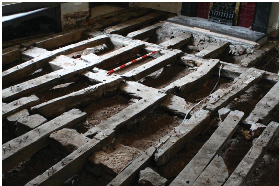
Plate 1. Ground beams and joists, viewed from the doorway ( 1m scale ).
