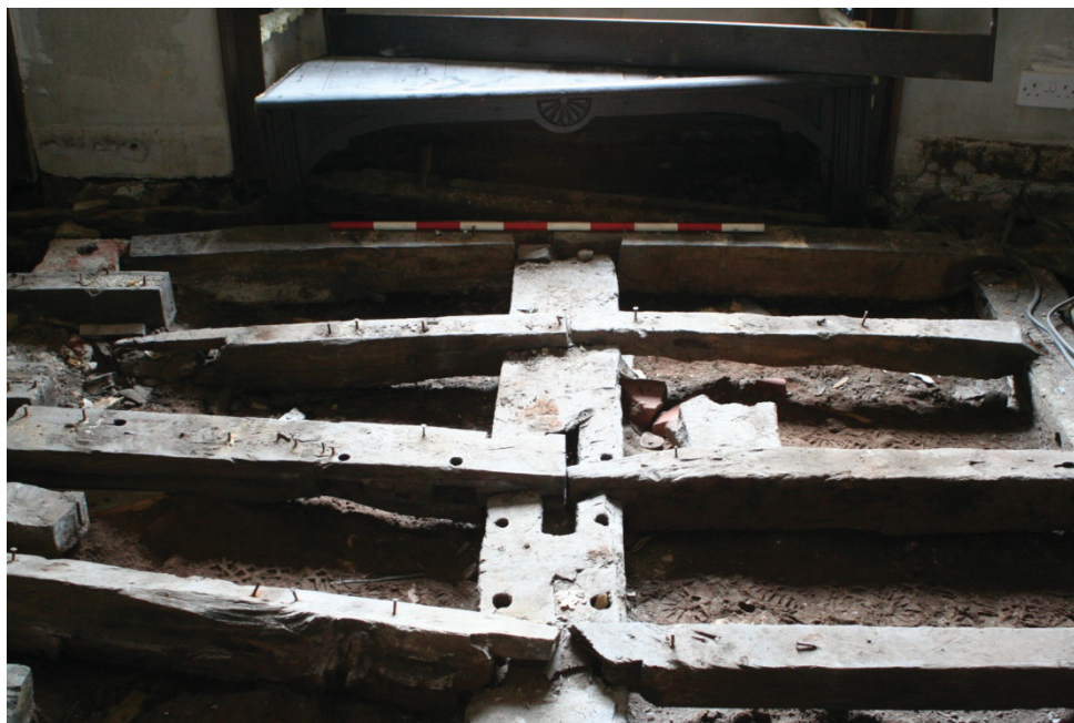
Plate 3. Central beam and joists, looking towards the window (1m scale).
