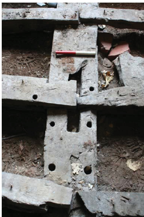
Plate 4. Central beam and joist detail (0.2m scale).
