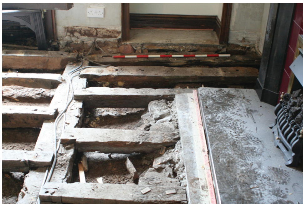
Plate 6. Floor joists near the fireplace, looking towards Cupboard 1 (1m scale).
