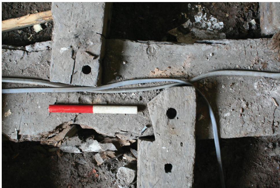
Plate 7. Beam and joist detail near the fireplace (0.2m scale).
