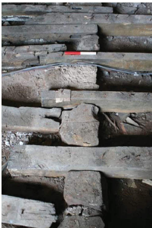
Plate 8. Stone bedding support between the window and Cupboard 2 (0.2m scale).
