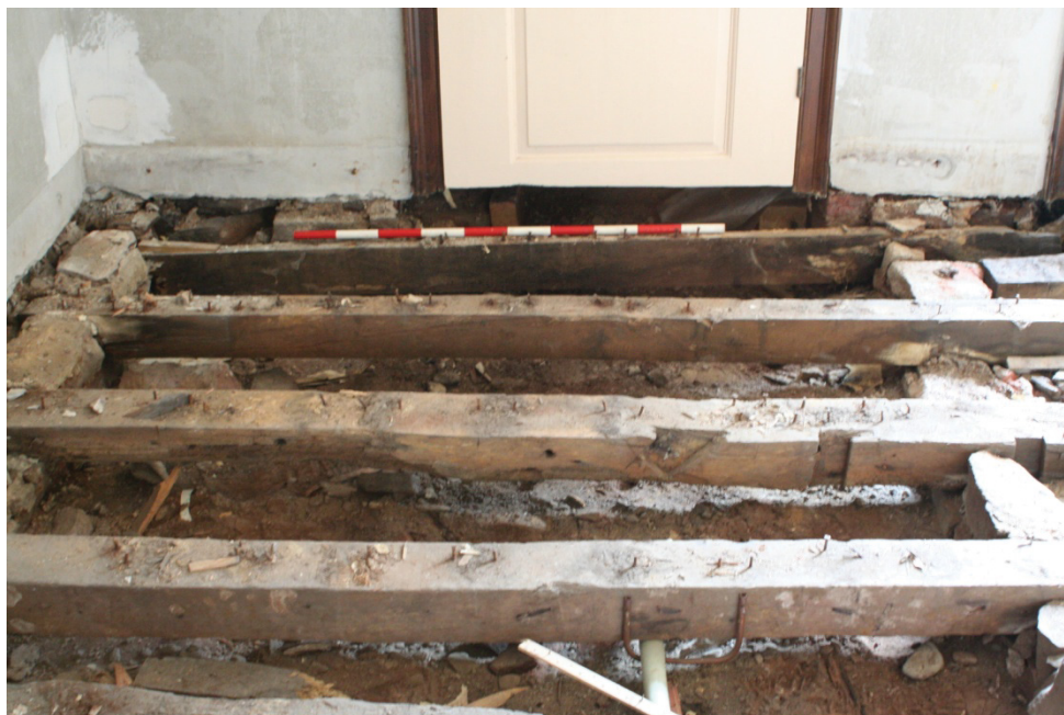
Plate 5. Floor joists, looking towards Cupboard 2 (1m scale).
