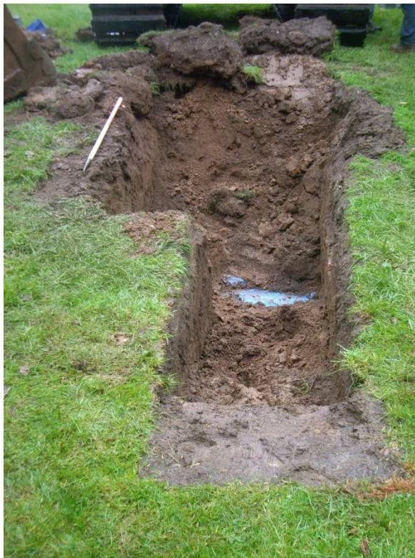
Plate 1: Overall shot of Trial Hole One (facing north)
