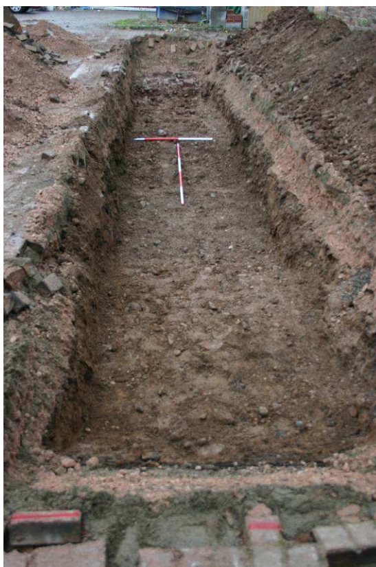
Plate 1: Trench 1 looking south-west. 1m/2m scale
