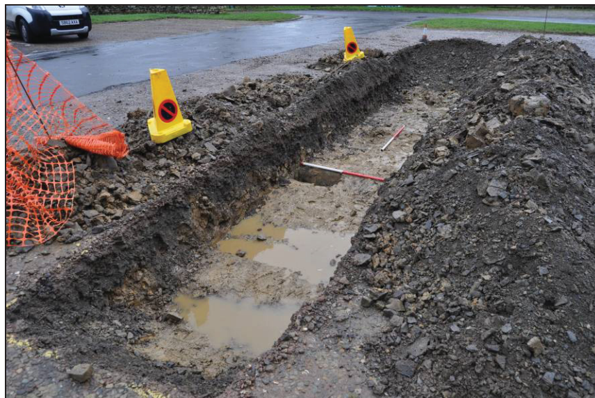
Plate 4: Trench 4 – Facing south-east, 2x1m scales
