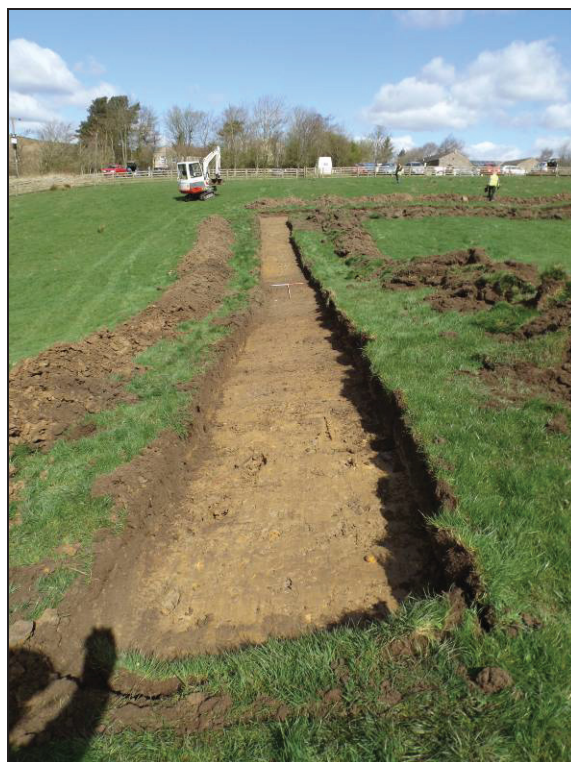
Plate 7: Trench 10 – Facing north-northwest
