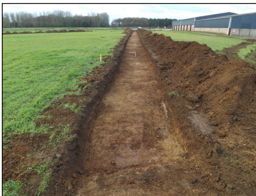
Plate 1: Shot of Trench 1, looking northeast
