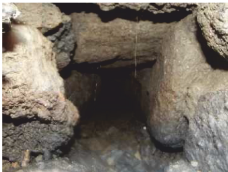
Plate 1: Stone built field drain – trial pit 59
