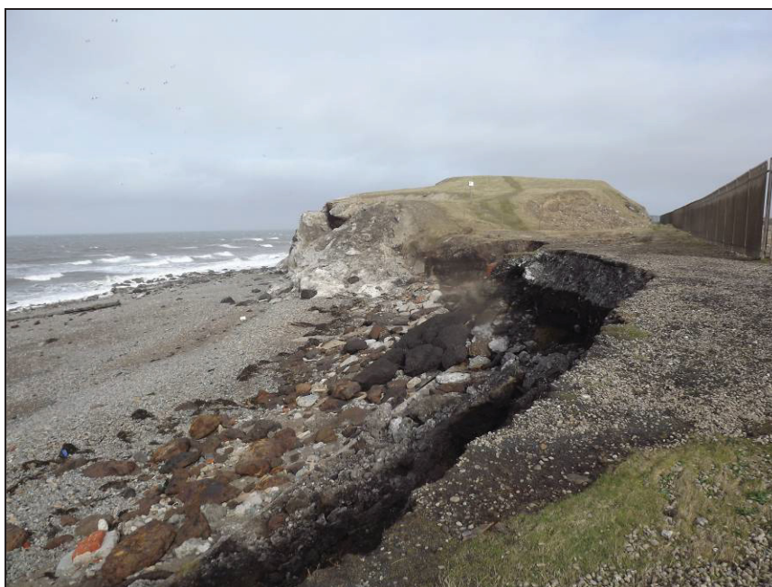
Plate 10: View looking north showing the 'slag bank' adjacent to the west side of the proposed development site
