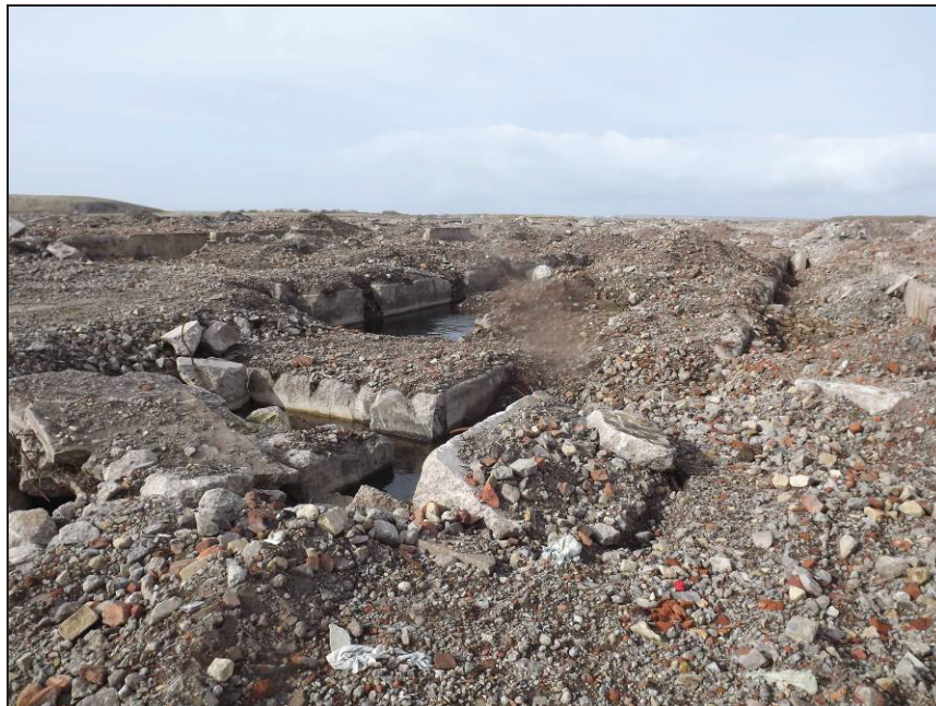
Plate 7: Central area of proposed development site showing concrete foundations
