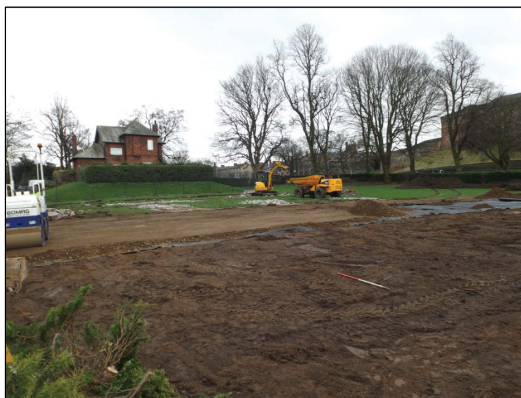
Plate 3: Topsoil strip facing southeast
