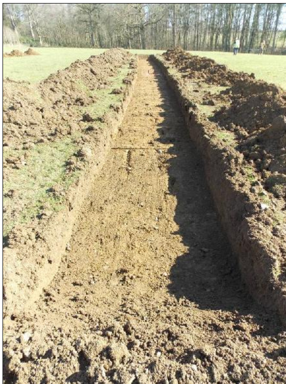
Plate 5: Trench 6 looking east-southeast
