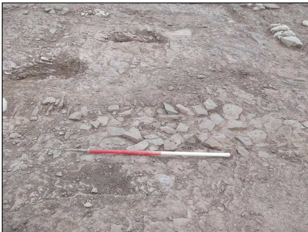
Plate 76: Trench [4217], showing foundation stones {4066} and wall {4019}, looking north
