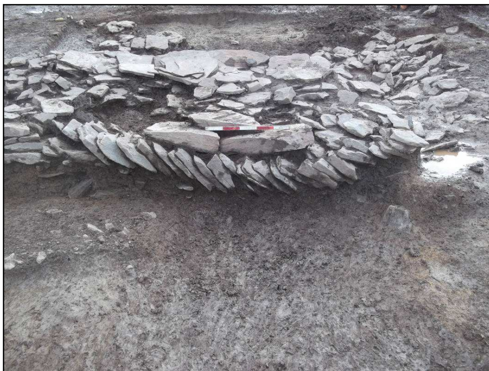
Plate 113: Repaired foundations {4228} and wall {4229}, looking south
