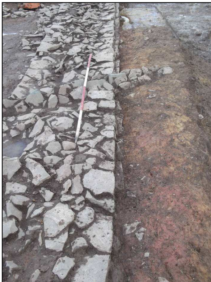
Plate 111: Foundation stones {3123}/{3226}, looking west
