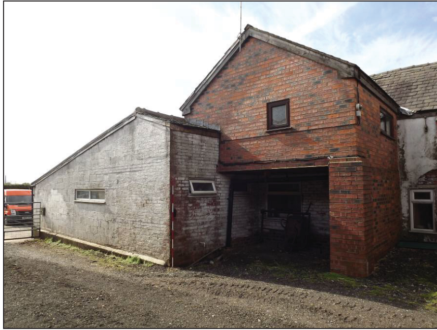
Plate 26: South end of the north-east elevation showing modern additions
