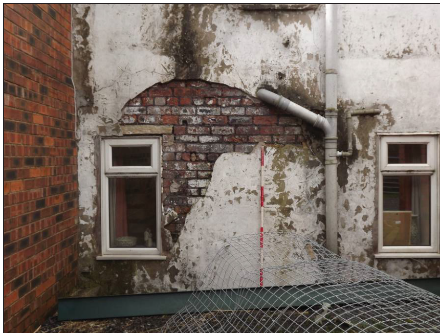
Plate 25: Detail of exposed brickwork of earliest phase of house, north-east elevation
