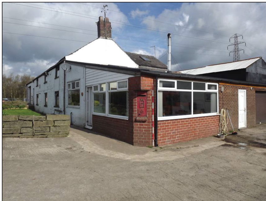
Plate 11: Single-storey extensions at south-east end of house
