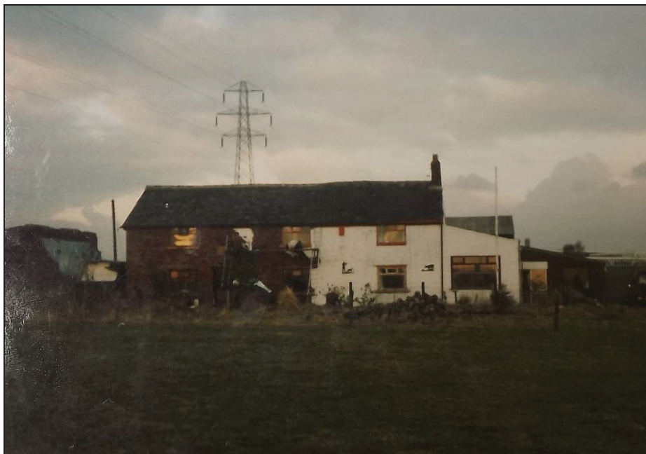
Plate 5: South-west elevation showing farm buildings at north end partly demolished
