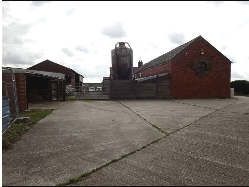
Plate 36: View looking south showing the farm buildings (left of photograph) in relation to the house range
