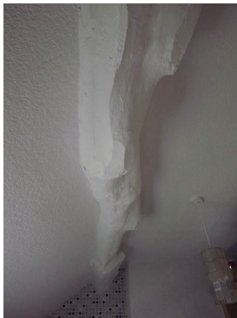
Plate 33: Detail of purlin in Bedroom 2
