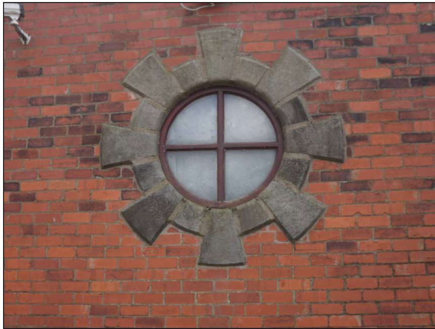
Plate 21: Detail of window in north-west elevation
