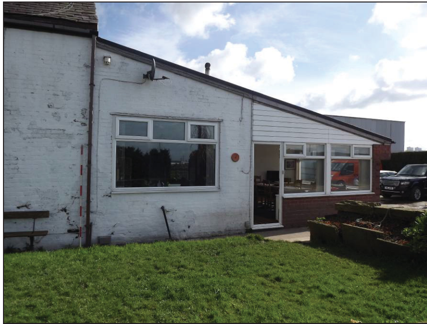
Plate 10: Single-storey extensions at the south-east end of the house, south-west elevation
