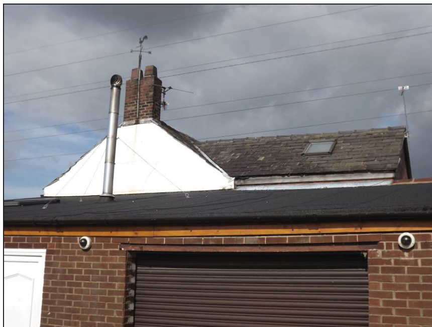
Plate 29: Detail of chimney stack, south-east elevation
