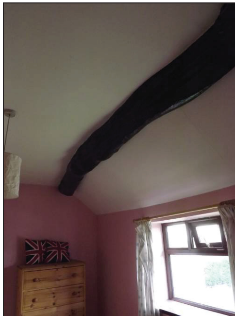
Plate 35: Detail of purlin in Bedroom 4
