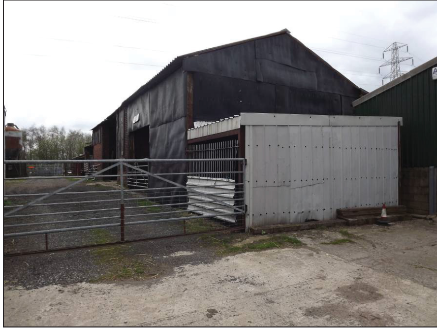
Plate 38: View looking north showing south-west elevation of large agricultural shed
