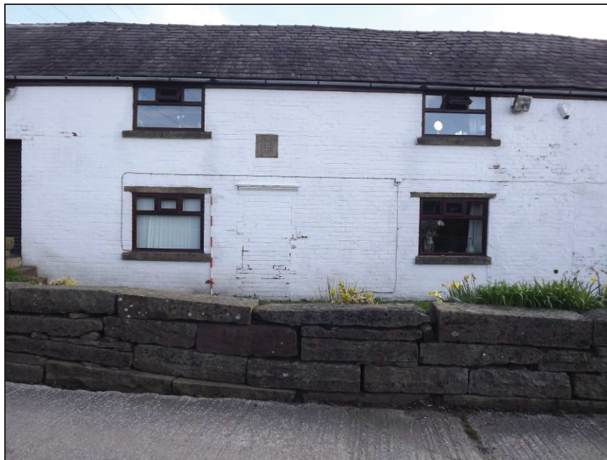
Plate 15: Central section of the south-west elevation showing the rebuilt section of the house and a former doorway
