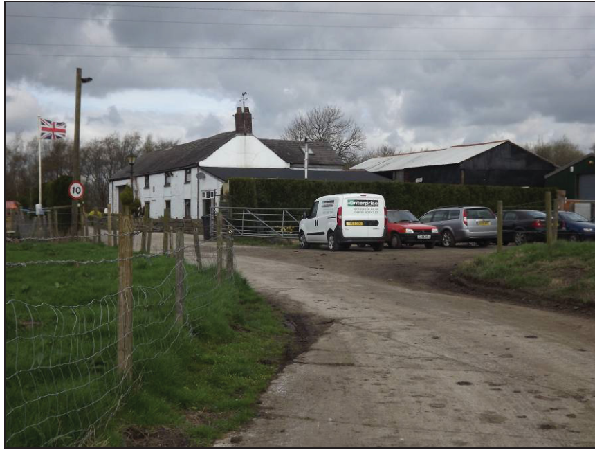
Plate 8: View looking north-west showing the house at Ferney Field Farm, with agricultural buildings to its north-east side
