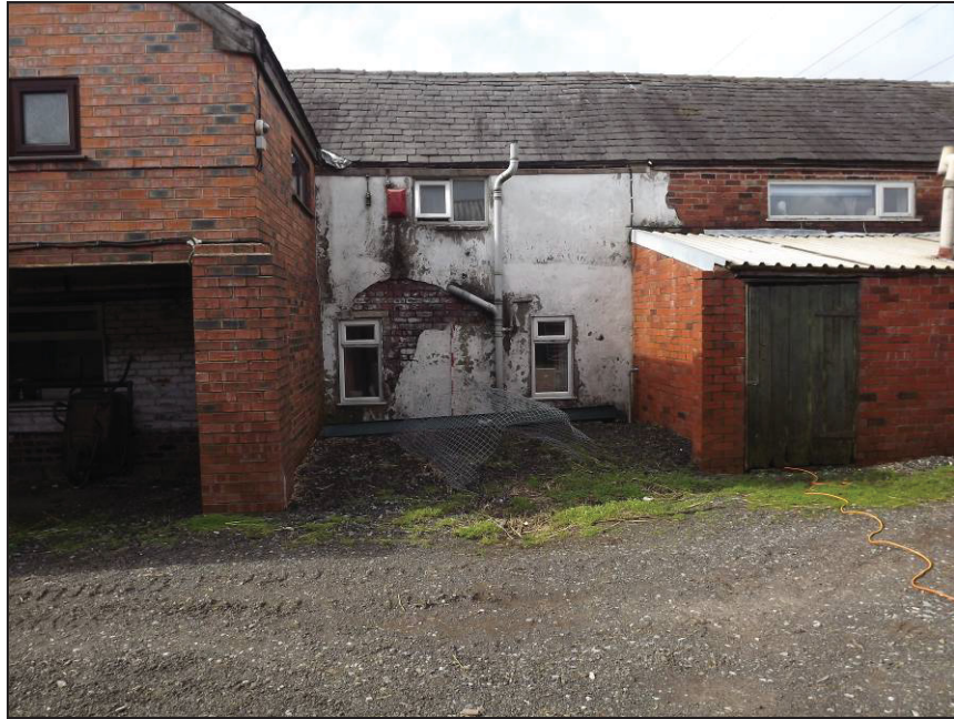
Plate 24: Earliest phase of the house covered in render, north-east elevation
