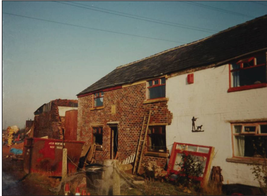
Plate 6: South-west elevation showing reconstructed section of house and partly demolished farm buildings
