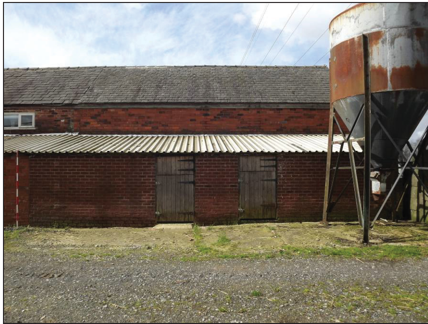
Plate 23: North-east elevation showing change in construction in roof covering and in brickwork
