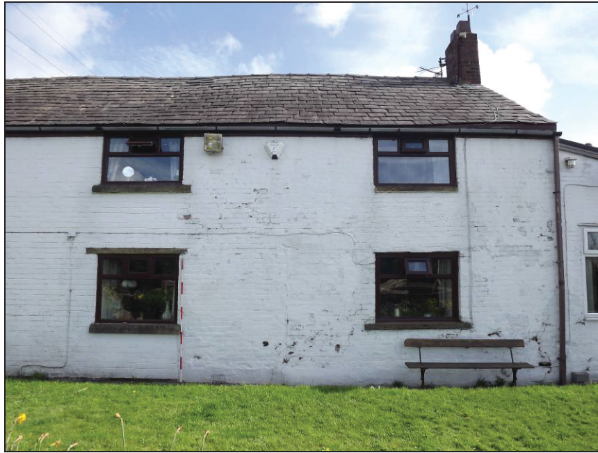
Plate 14: South-west elevation showing earlier brickwork and blocked doorway, with reconstructed section of house to the left of the ranging pole
