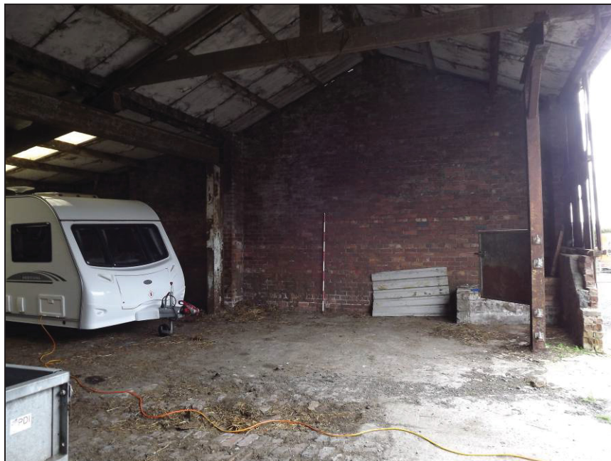
Plate 39: View looking south showing interior wall of agricultural shed
