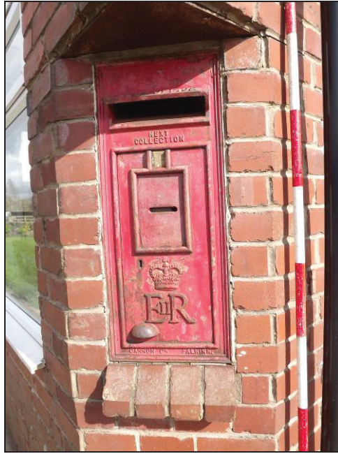
Plate 12: Detail of salvaged post box built into the south-east extension
