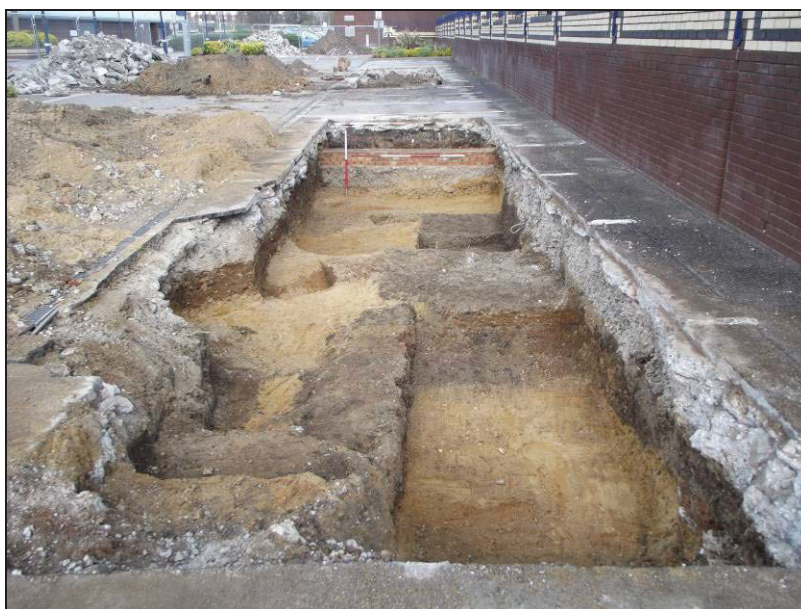
Plate 13: Overview of Trench 4b, looking north
