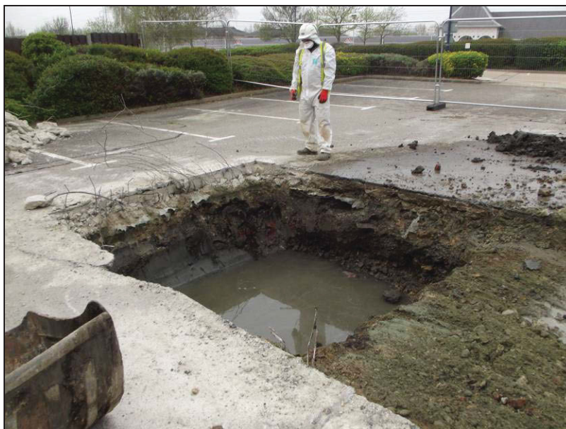
Plate 6: Water polluted with Hydrocarbons at the southern extent of Trench 2b, looking south-west
