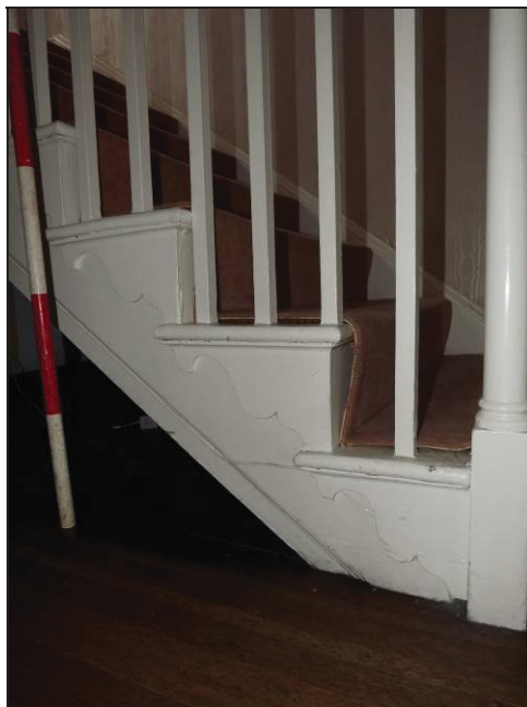
Plate 44: Detail of tread ends, main staircase in Room 4
