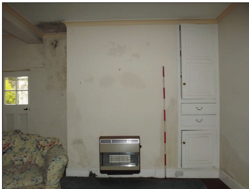
Plate 51: East wall of Room 8 showing possible original cupboards and location of fireplace
