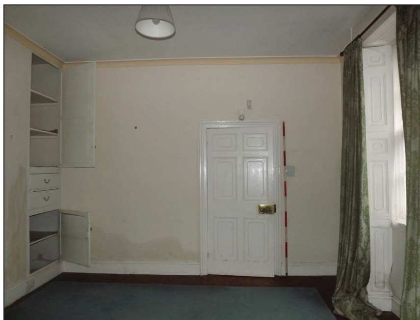
Plate 50: South wall of Room 8 showing the same detailing on the door and window surround (Scale = 2m)
