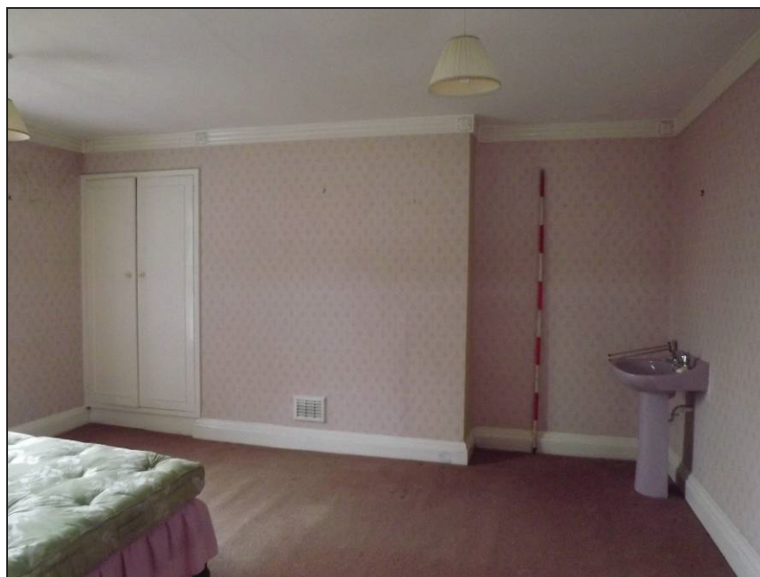
Plate 70: West wall of Room 18 showing projecting chimney breast of former fireplace
