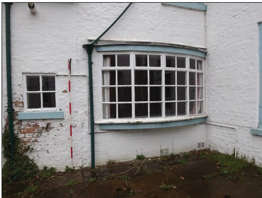
Plate 22: Detail of inserted bay window, west elevation of east wing
