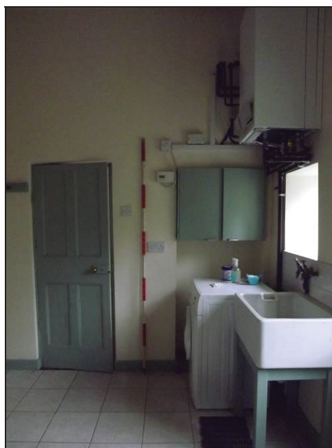
Plate 62: South wall of Room 12 showing present door to Room 11, and possible blocked door to right of photograph
