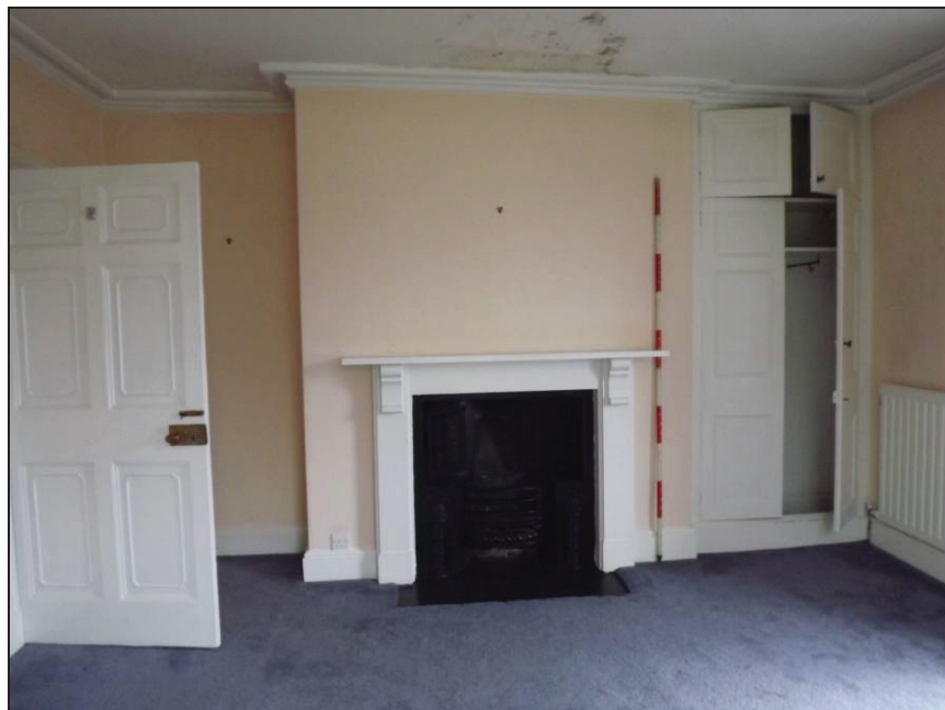
Plate 72: East wall of Room 19 showing hob grate fireplace
