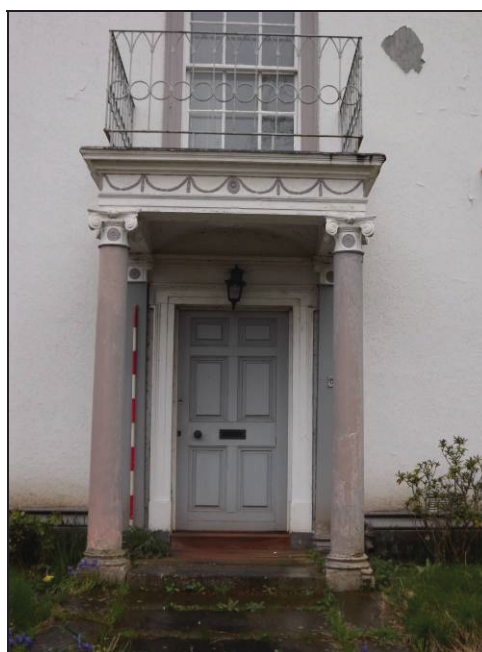
Plate 7: Detail of main entrance, south elevation (Scale = 2m)
