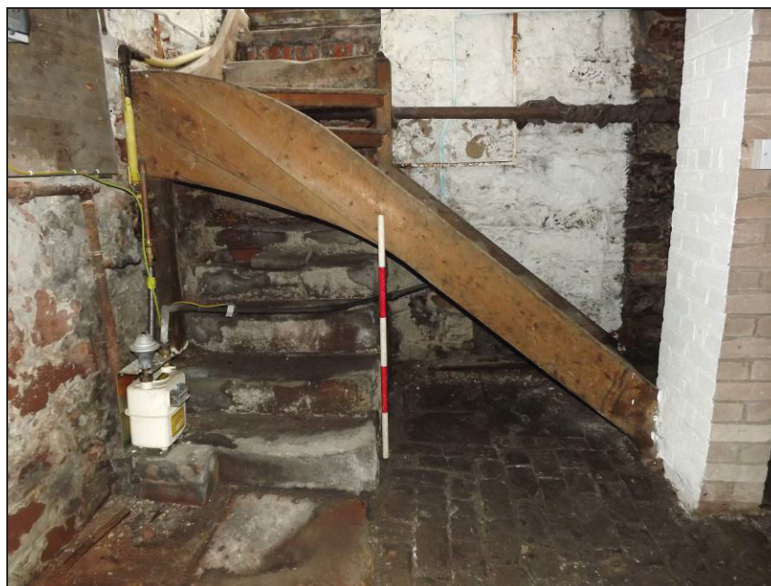
Plate 89: View looking north showing the original stone steps to the cellar and the present wooden stairs (Scale = 1m)
