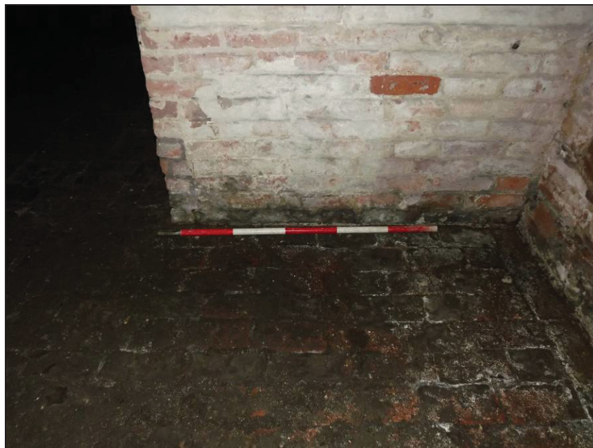
Plate 91: Detail of brick floor, cellar (Scale = 1m)
