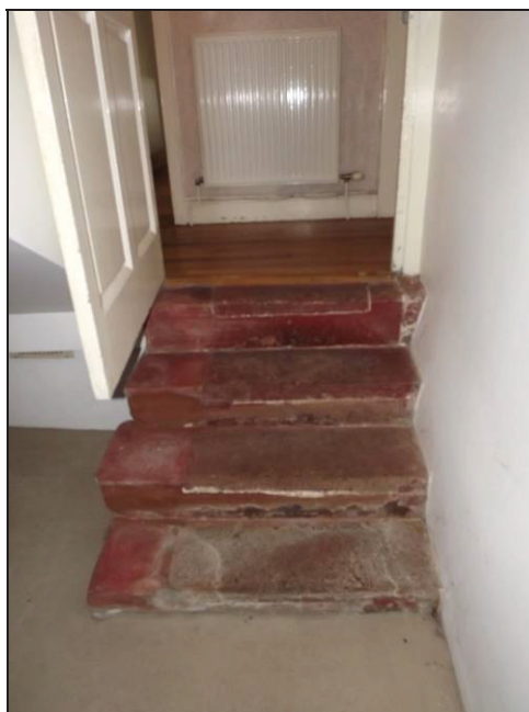
Plate 57: View looking west showing the stone steps in Room 10
