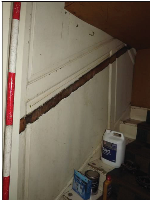
Plate 56: Detail of panelling for former staircase, Room 10
