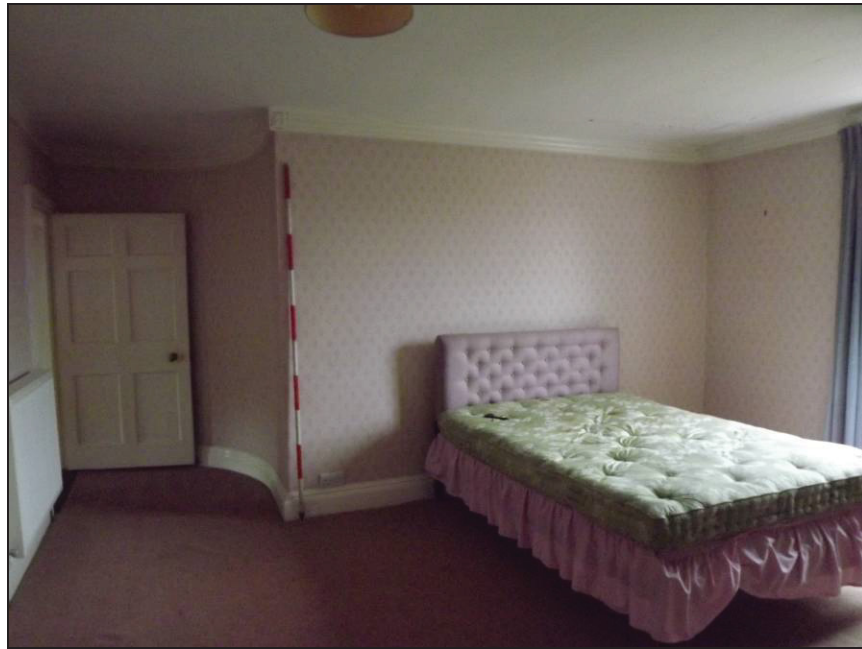
Plate 71: East wall of Room 18 showing curved wall (Scale = 2m)
