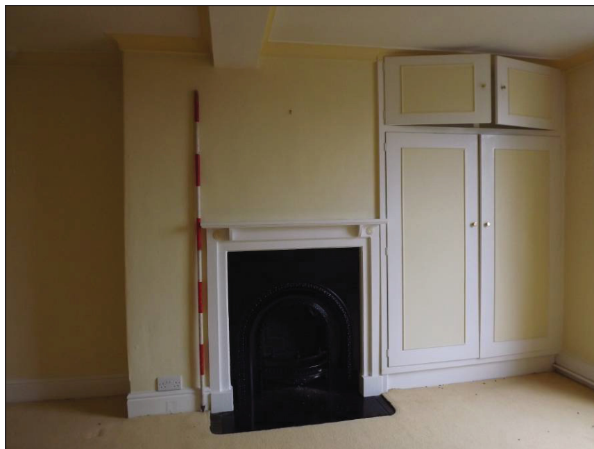
Plate 84: Fireplace and cupboard, east wall of Room 24
