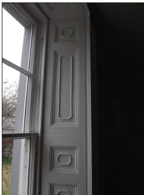
Plate 29: Detail of window surround, south wall of Room 1
