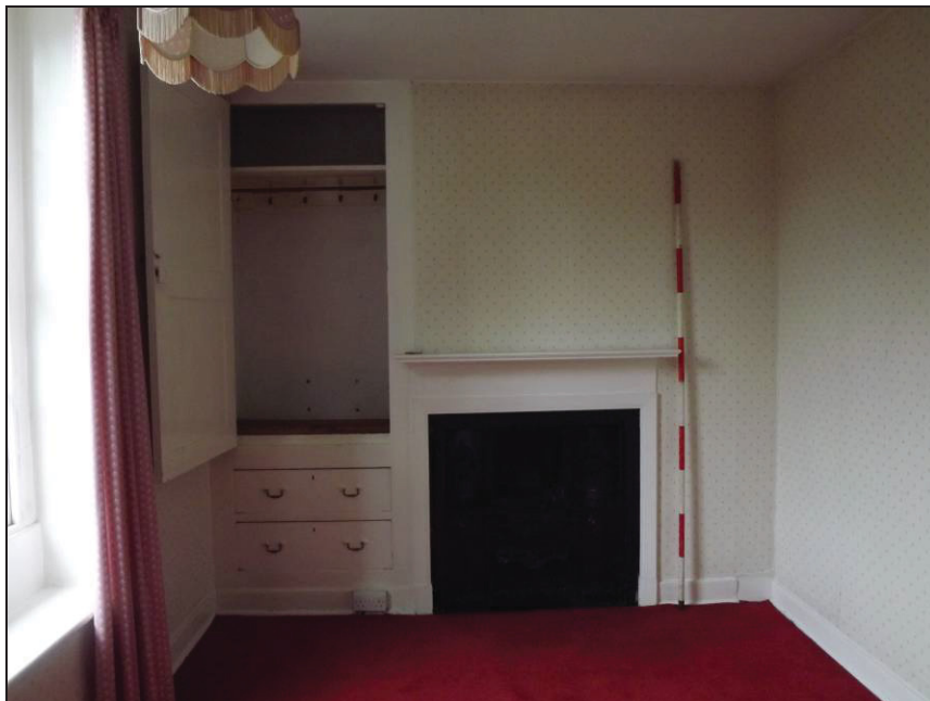
Plate 65: Fireplace, east wall of Room 15
