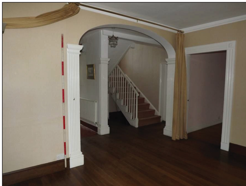
Plate 32: Arched opening, north wall of Room 1
