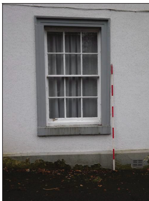
Plate 13: Detail of window in west elevation (Scale = 2m)
