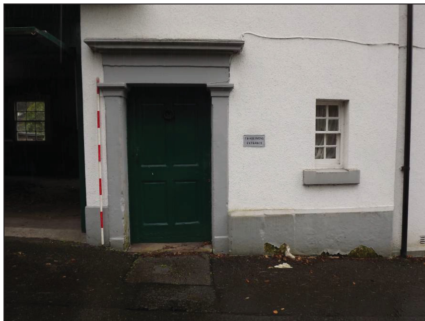
Plate 12: Northern doorway, west elevation, with 'Tradesmens Entrance' sign
