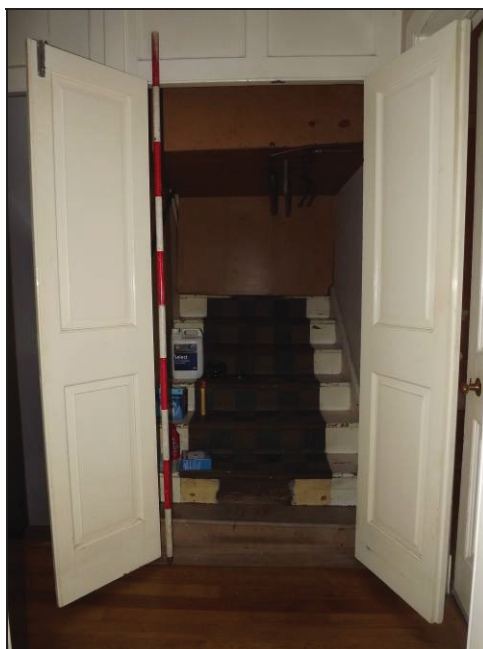
Plate 55: Detail of former staircase, ground floor Room 10
