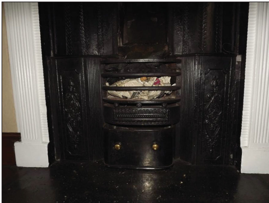
Plate 28: Detail of hob grate, Room 1
