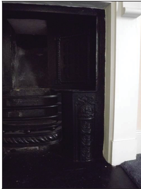
Plate 73: Detail of fireplace, Room 19
