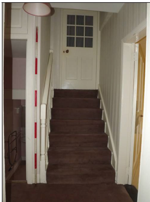
Plate 85: View looking east showing part of the stairway in Room 25, with the bathroom in the lower section of the former staircase to left of photograph
