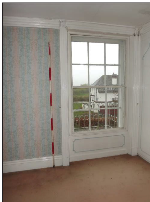
Plate 82: Detail of window surround, south wall of Room 23
