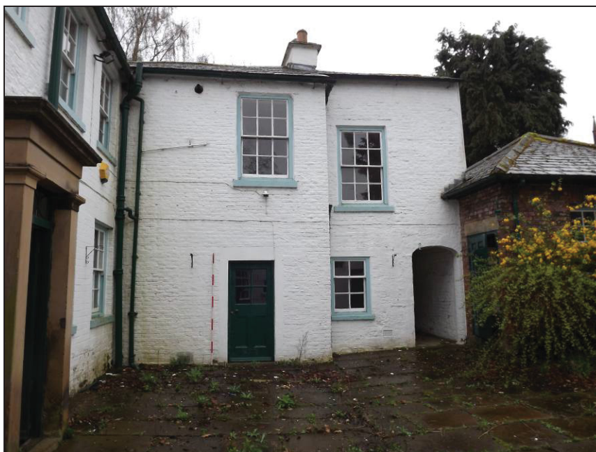
Plate 23: East elevation of the western wing (Scale = 2m)
