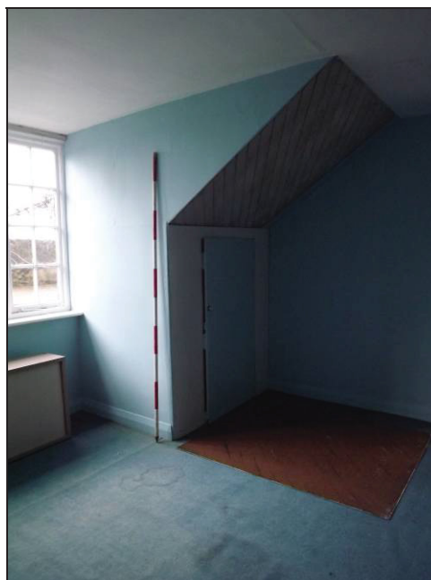
Plate 88: Detail of the form of the south side of the roof to create one of the dormers
