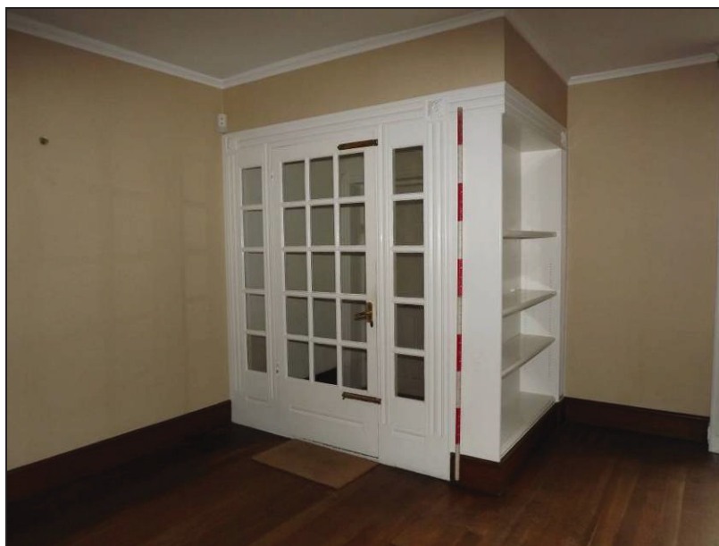
Plate 25: Detail of vestibule, south-east corner of Room 1
