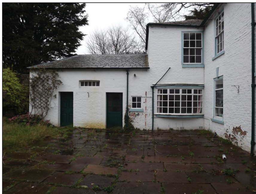
Plate 21: West elevation of the east wing (Scale = 2m)
