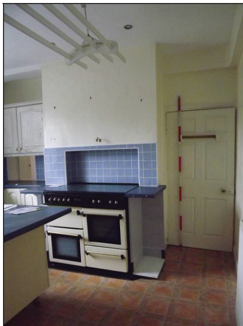
Plate 46: Location of former fireplace or range, east wall of Room 5
