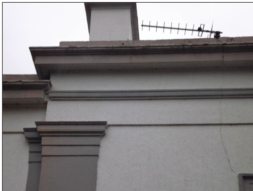
Plate 6: Detail of eaves cornice, south elevation
