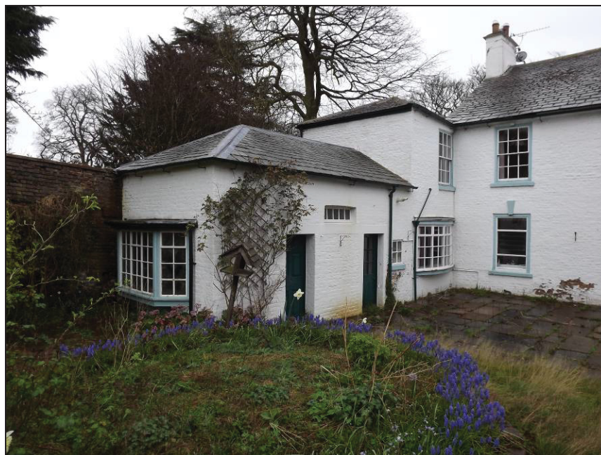
Plate 20: East wing showing two-storey section and one-storey addition
