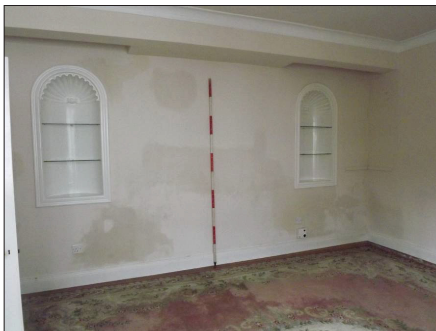
Plate 59: Detail of niches, east wall of Room 11
