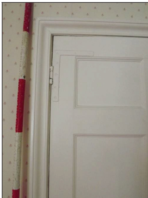
Plate 67: Detail of L-shaped hinge, Room 15
