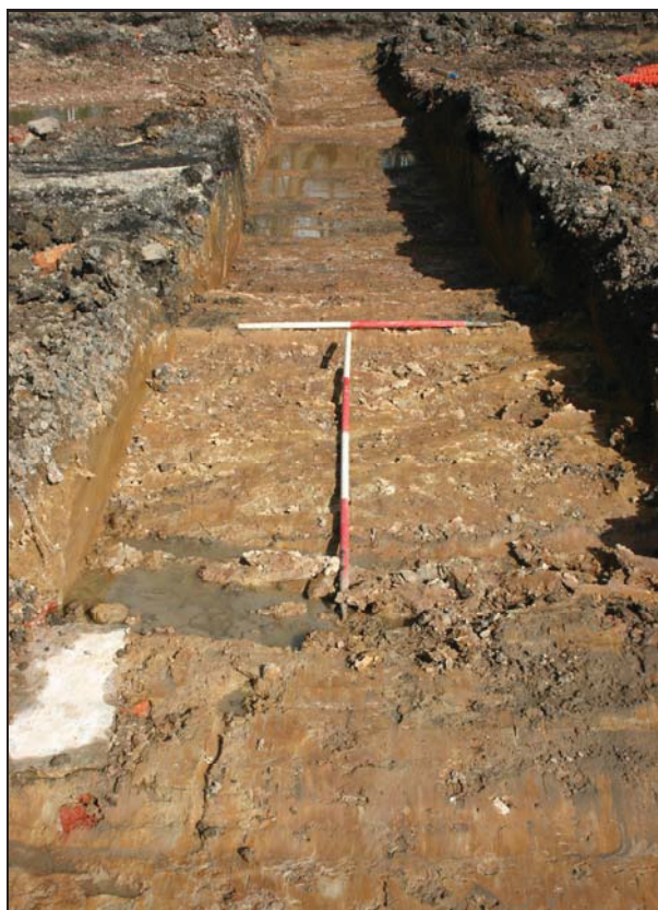
Plate 8: Trench 7 looking east showing location of possible wall foundation
