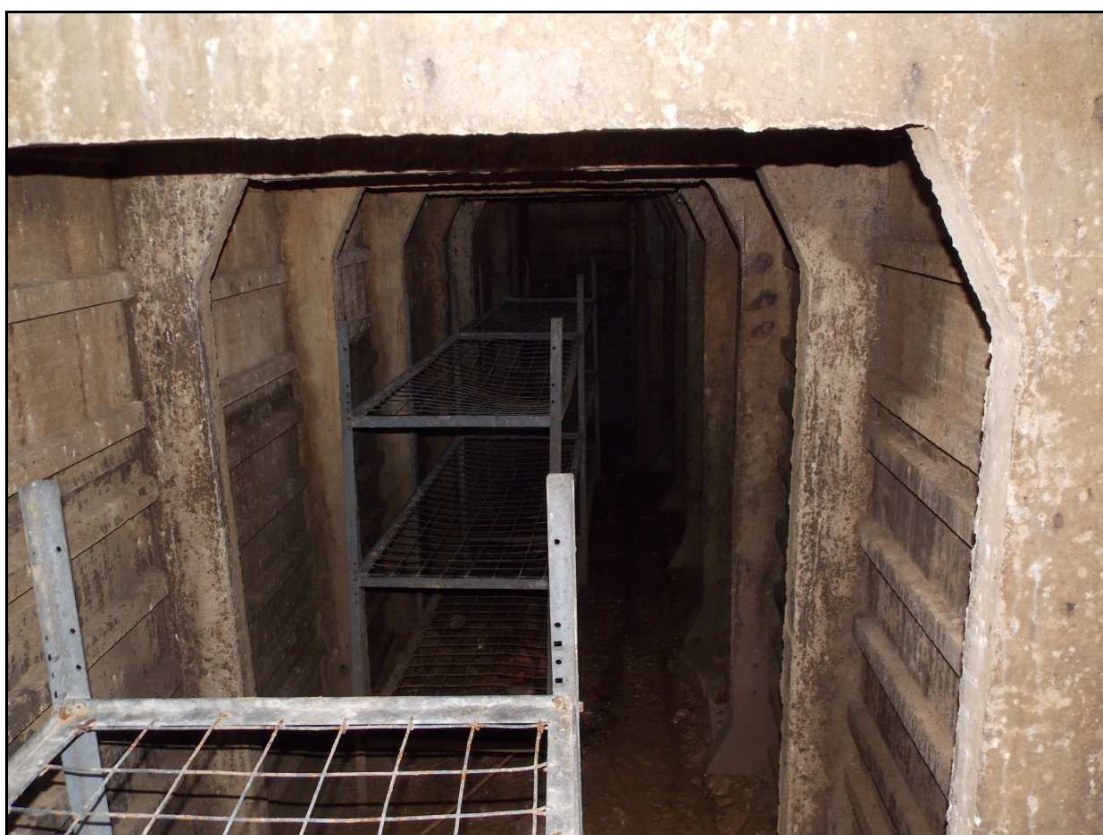
Plate 10: Interior shot of corridor D, showing bunk beds, looking south
