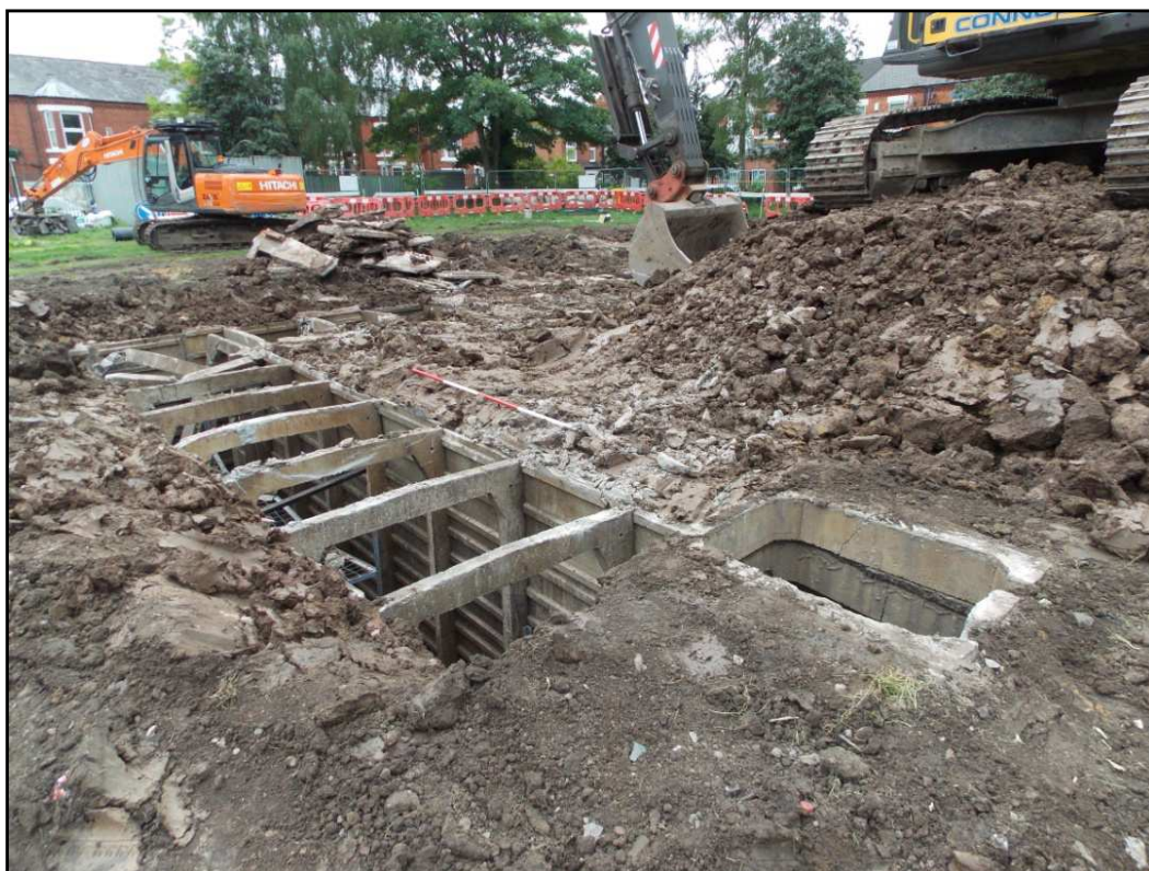
Plate 2: Shot of corridor E, showing escape hatch {110}, looking southwest
