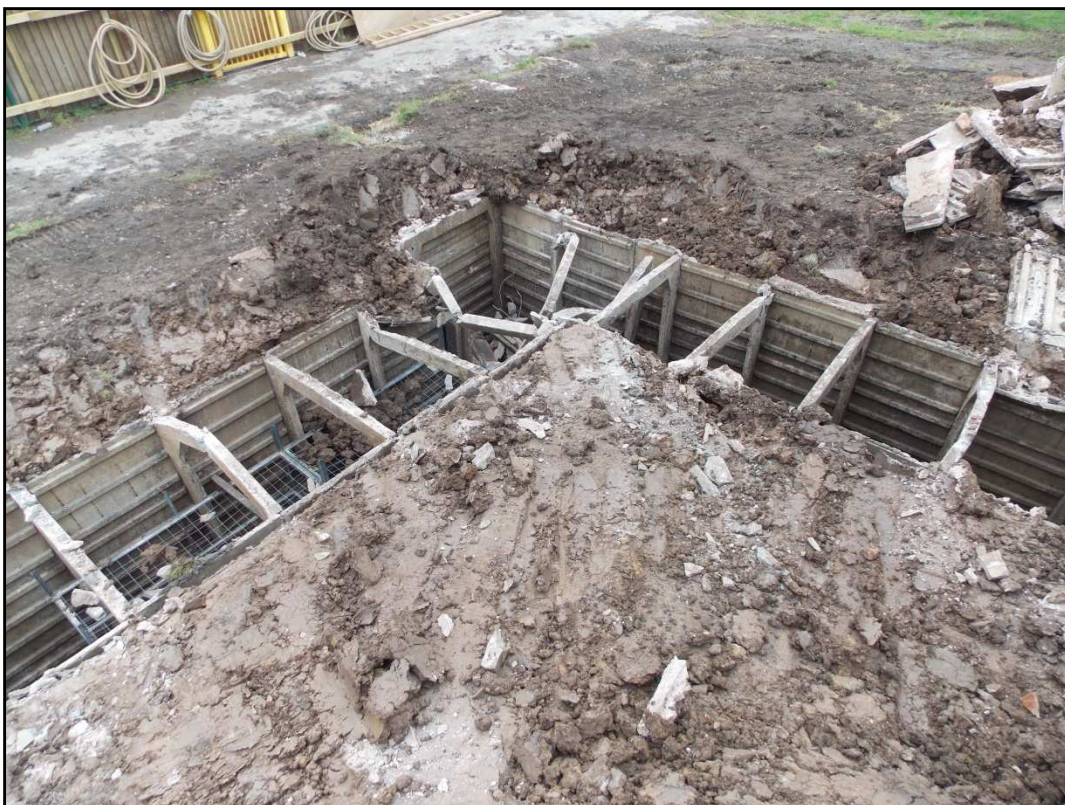
Plate 5: Shot of corridors C & E, showing bunk beds on left side, looking southeast
