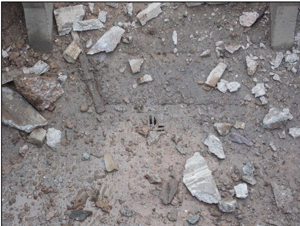
Plate 15: Close-up shot of drain in corridor A, looking north
