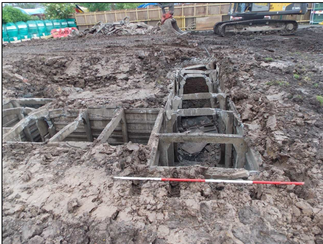
Plate 9: Shot of corridors A & B with bricked up entrance in the background, looking east
