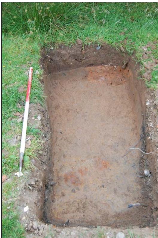
Plate 3 Trial trench 2 facing north.
