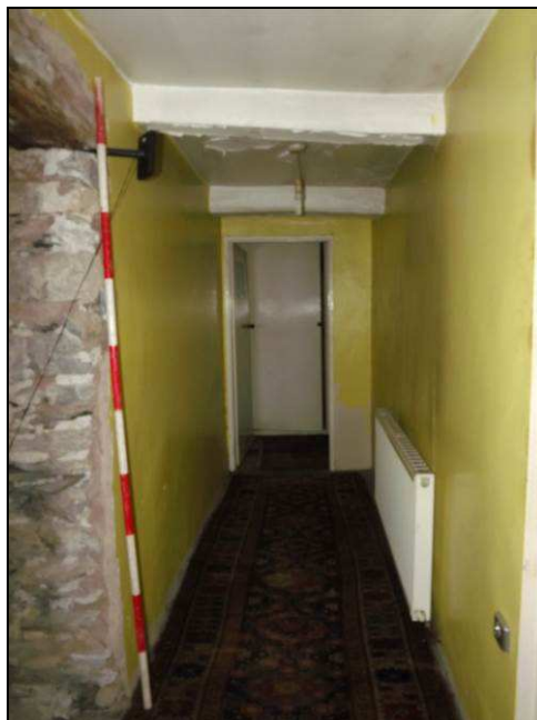
Plate 29: Detail of first floor corridor showing exposed roof tie beams
