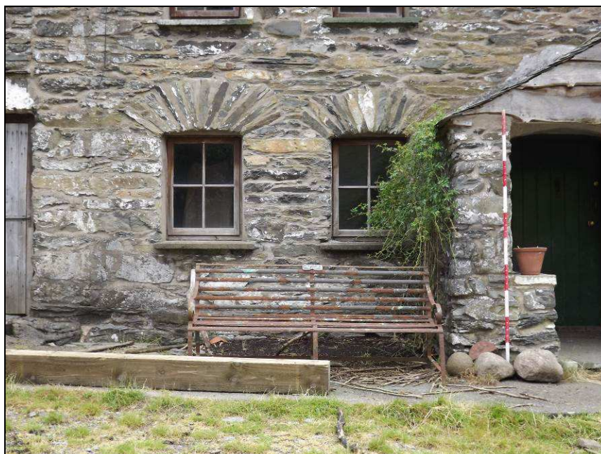
Plate 7: South-west elevation of the house showing modern windows
