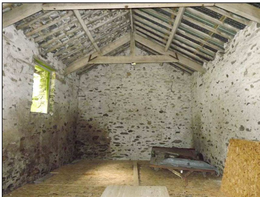
Plate 53: View looking south-east showing the interior of the barn, Building B
