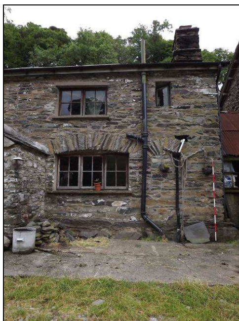
Plate 8: South-west elevation showing modern window openings and blocked fire window
