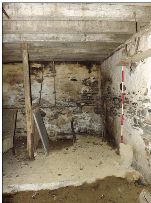
Plate 51: Detail of one of the stalls in the shippon
