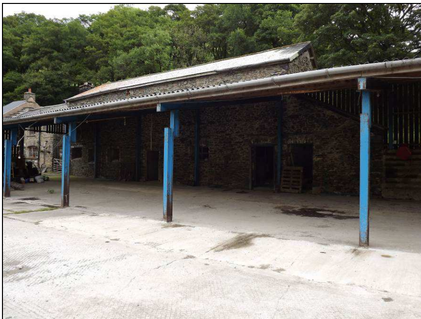
Plate 42: South-west elevation of Building B partly obscured by a modern shed
