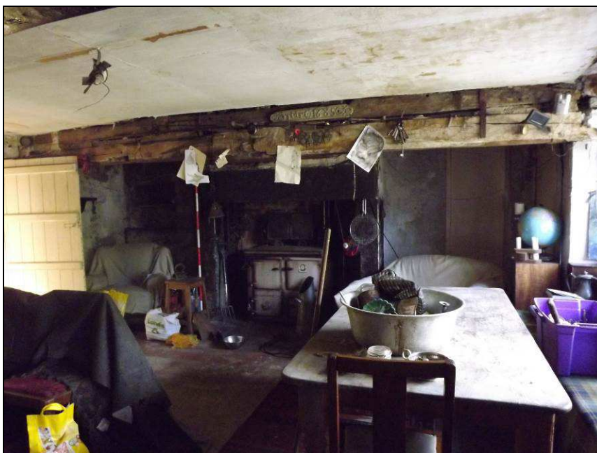
Plate 13: Detail of the large timber beam and later range, living room
