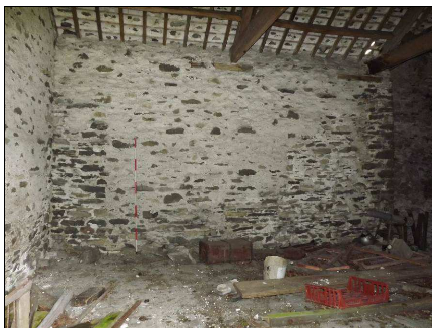
Plate 38: Interior of upper barn, Building A
