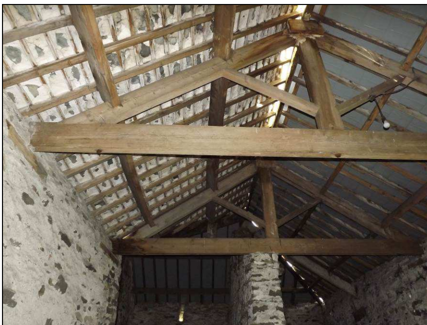
Plate 40: Detail of upper barn roof trusses, Building A
