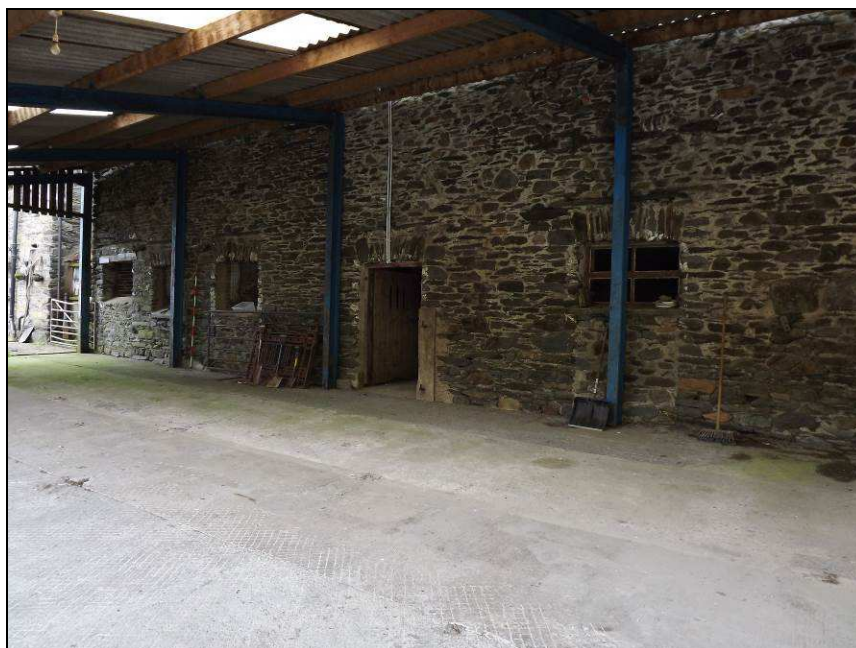
Plate 43: South-west elevation of Building B showing present doorway and windows
