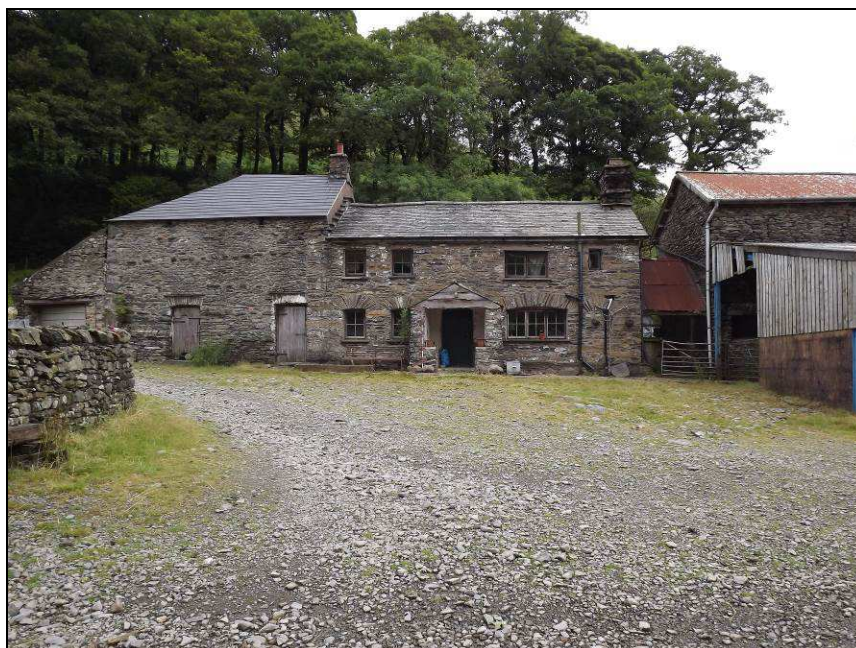
Plate 3: South-west elevation of the house and farm buildings at Low Borrowdale Farm
