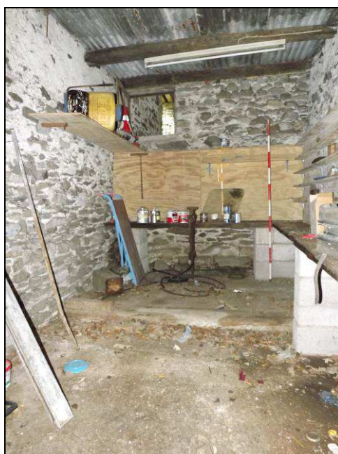
Plate 37: Interior of workshop, Building A
