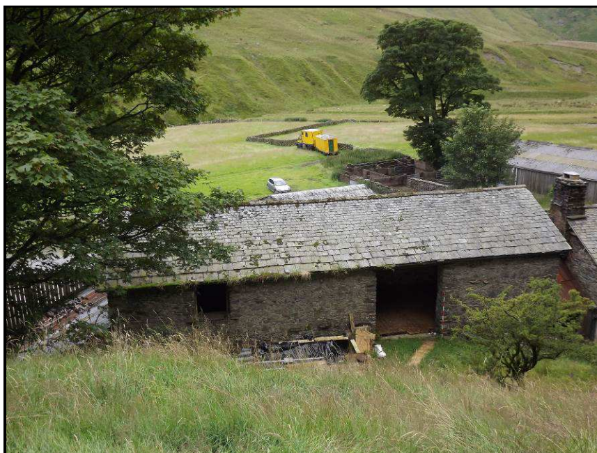
Plate 46: View looking south-west from the north-east side of Building B showing the increase in ground level
