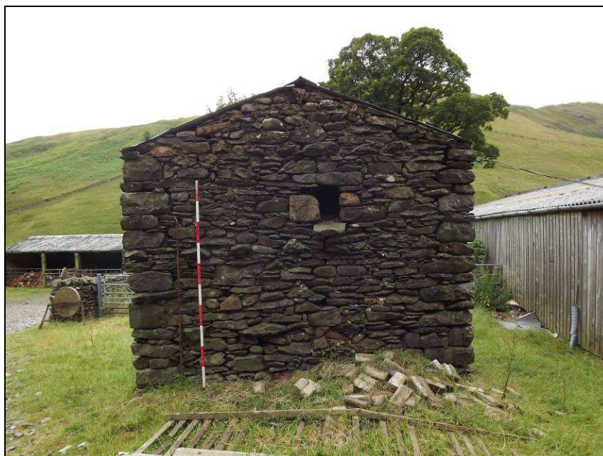
Plate 57: North elevation of Building C
