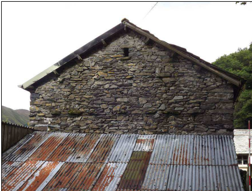
Plate 45: South-east elevation of Building B showing the square owl hole
