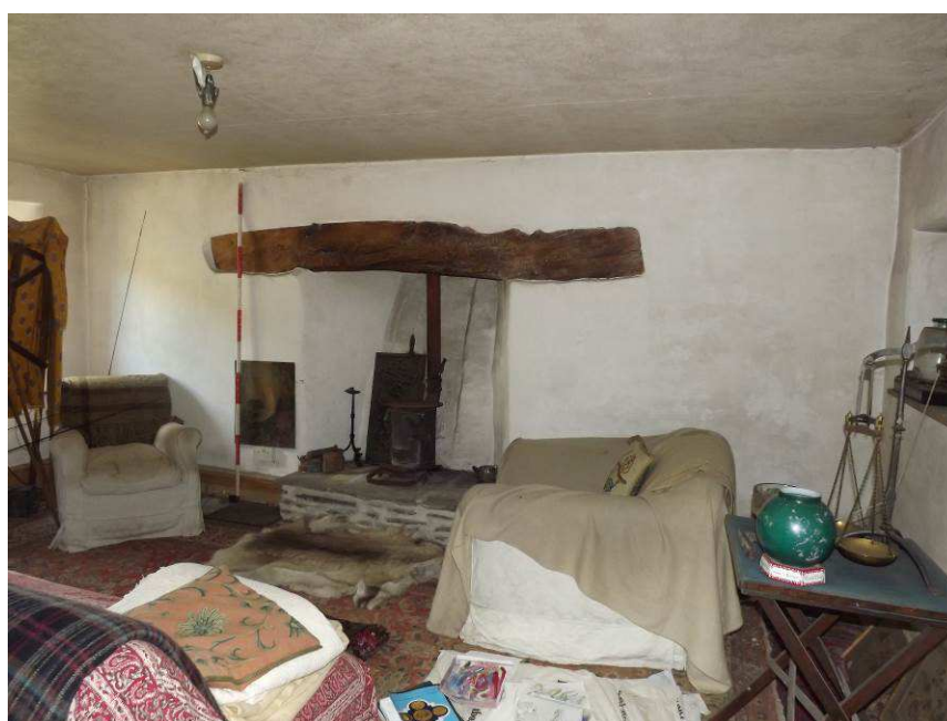
Plate 18: North-west wall of snug (former parlour) showing possible inserted fireplace (Scale = 2m)
