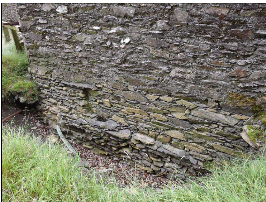
Plate 12: Detail of projecting stonework at base of central projection to the north-east elevation of the house
