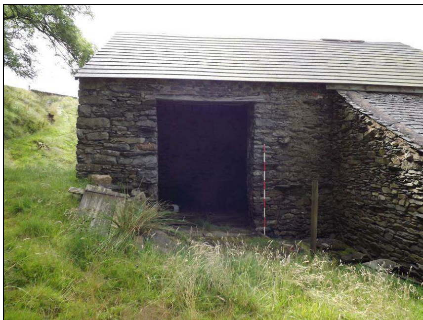
Plate 35: Large doorway in the north-west elevation of Building A
