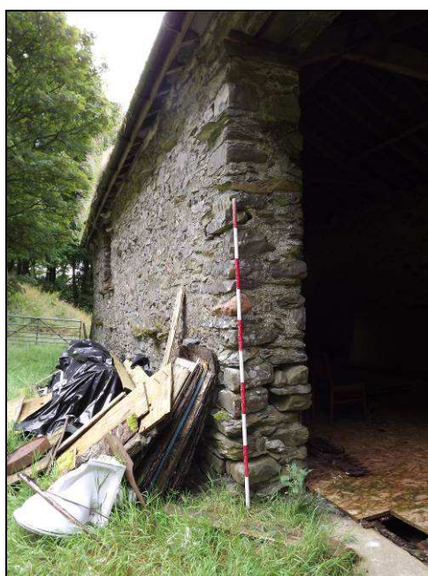
Plate 48: Detail of jamb of doorway, north-east elevation of Building B
