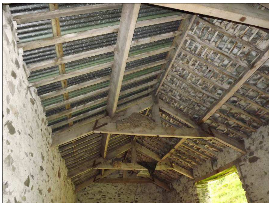
Plate 54: Detail of roof structure, Building B
