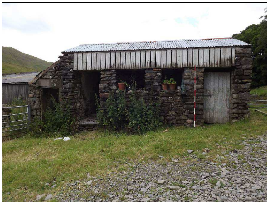
Plate 56: East elevation of Building C (Scale = 2m)
