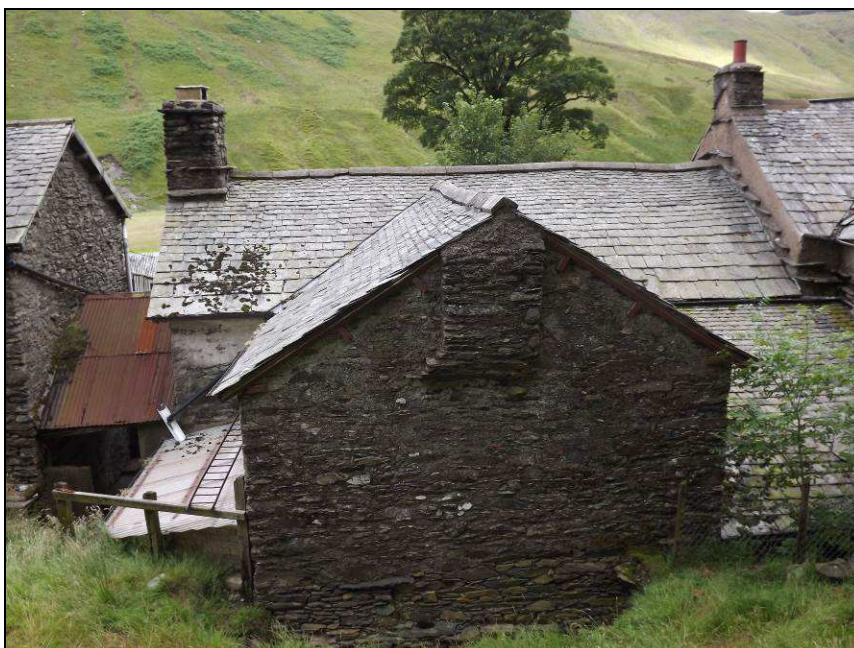
Plate 11: Two-storey projection to the main house, north-east elevation
