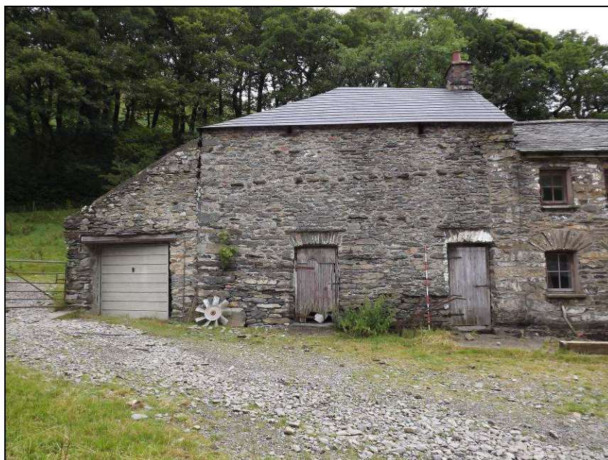
Plate 31: South-west elevation of Building A
