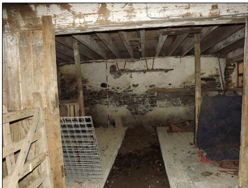
Plate 50: Interior of shippon in Building B showing stalls to either side of a central manure passage (Scale = 2m)
