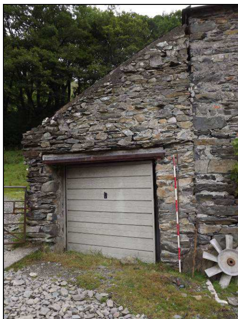
Plate 33: Garage at north-west end of Building A (Scale = 2m)
