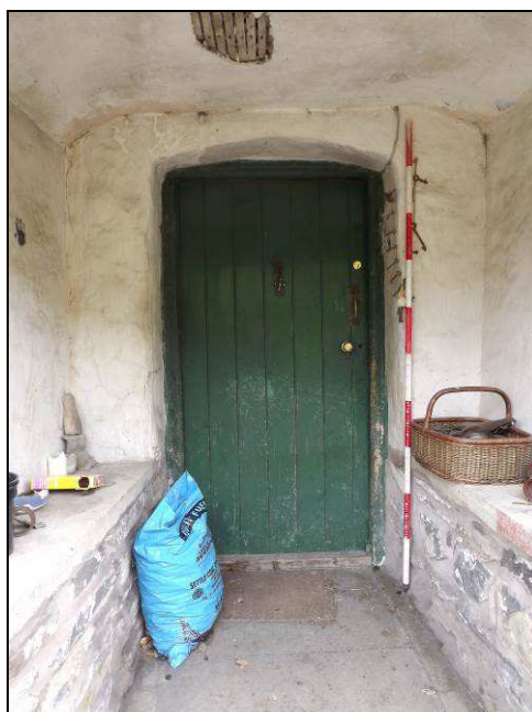
Plate 6: Detail of main entrance housed within the porch, south-west elevation
