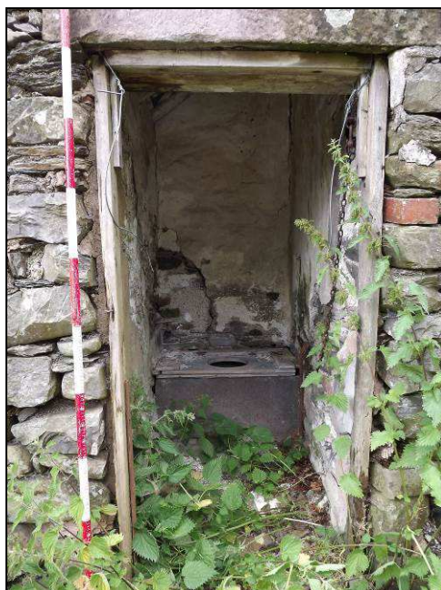
Plate 59: Detail of privy/earth closet, Building C
