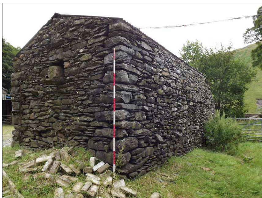
Plate 58: North and west elevations of Building C
