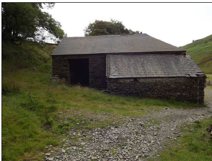
Plate 34: North-west elevation of Building A and the Garage
