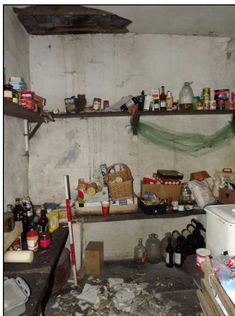
Plate 26: Interior of larder showing stone and wooden shelves (Scale = 1m)
