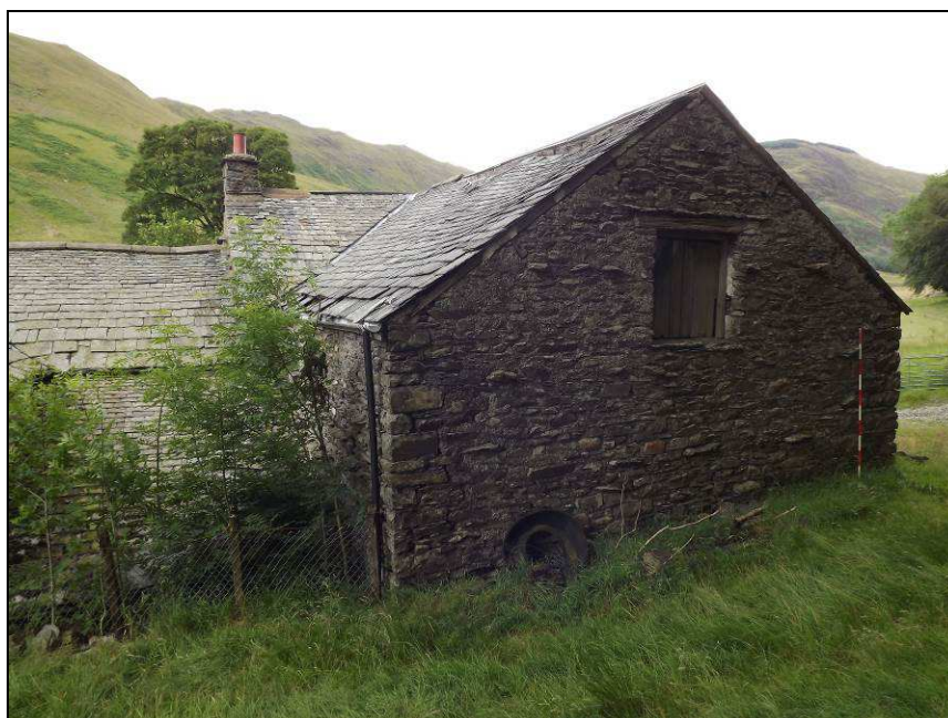
Plate 36: North-east elevation of Building A showing the pitching hole
