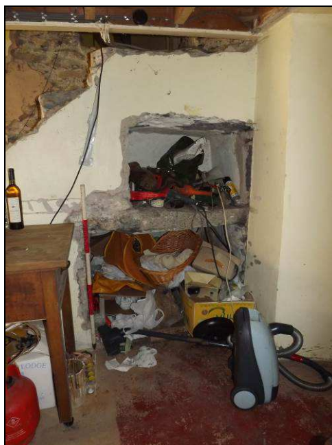
Plate 21: Detail of recesses below the staircase in the kitchen (Scale = 1m)
