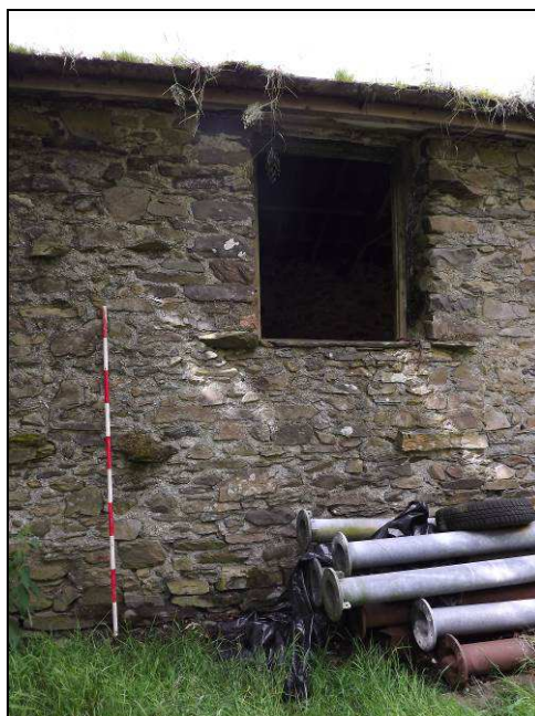
Plate 49: Pitching hole, north-east elevation of Building B
