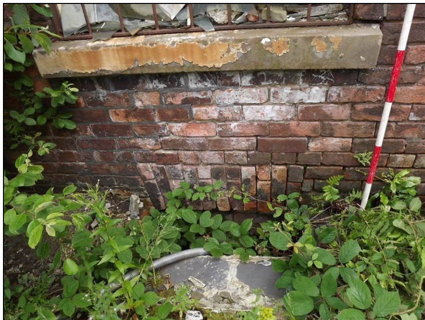
Plate 25: Basement window, west elevation
