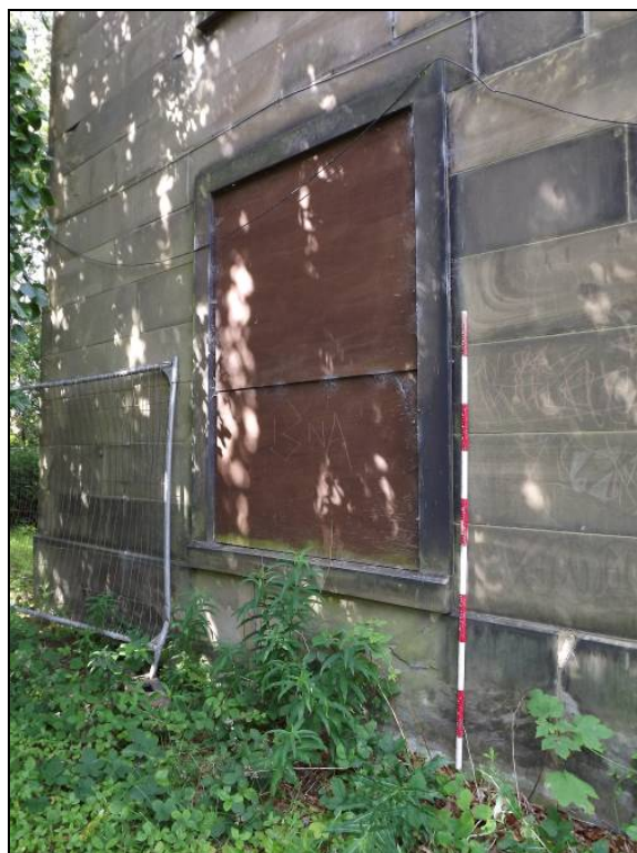
Plate 8: Detail of ground floor window surround, east elevation
