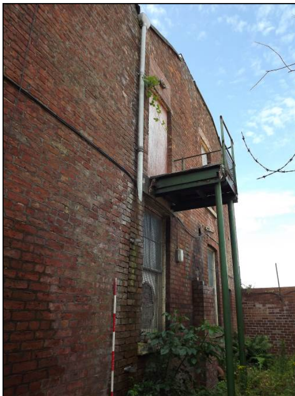
Plate 17: North elevation showing vertical construction break (in line with the white downpipe)
