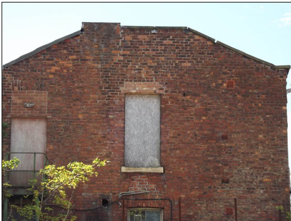
Plate 21: North elevation showing two windows, one of which has been converted to a fire escape
