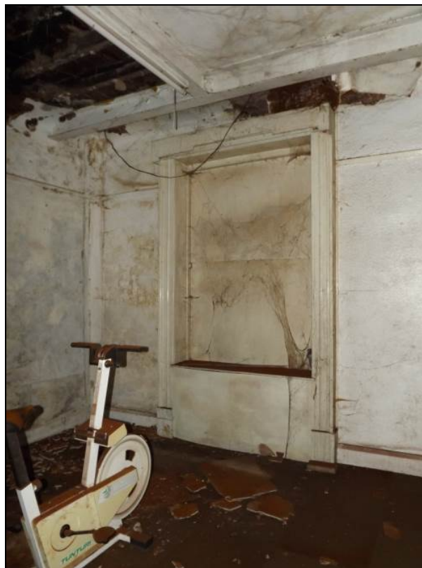
Plate 40: Original window surround, east wall of north-east room
