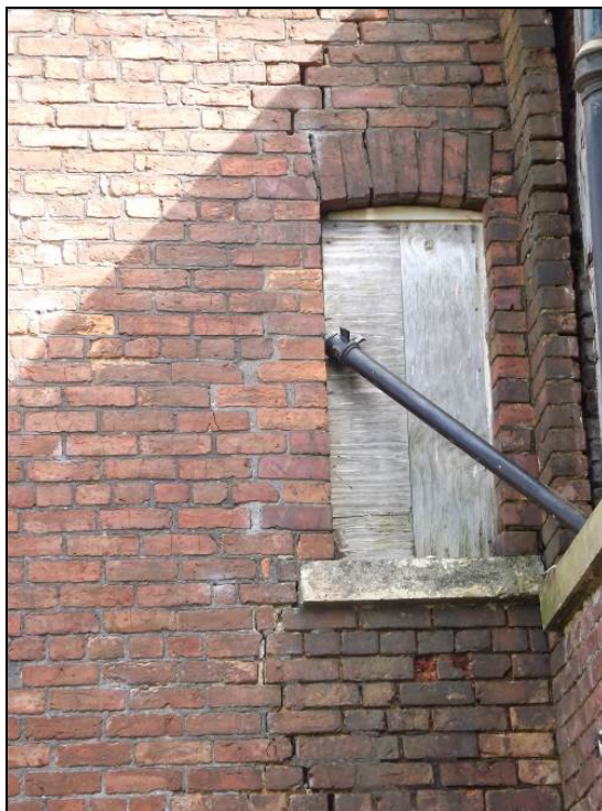
Plate 27: Detail of first floor windows in south elevation of addition
