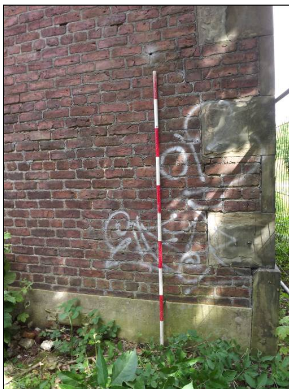
Plate 12: South-east corner of Bramhall House showing the ashlar quoins and brickwork of the south elevation (Scale = 2m)
