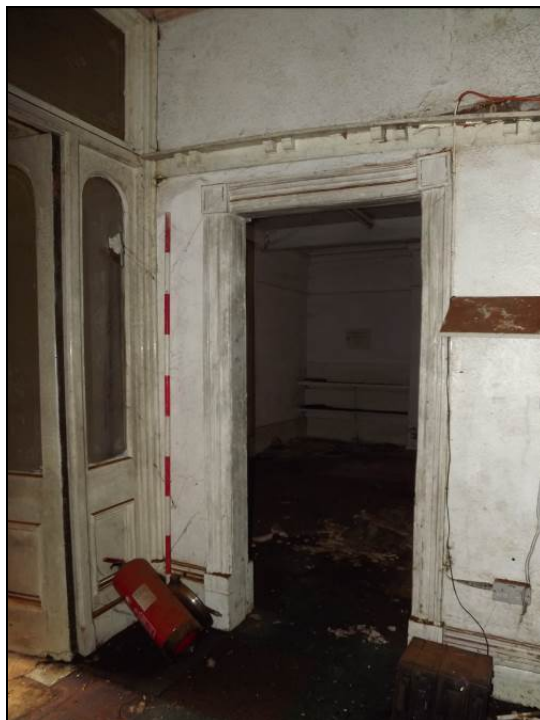
Plate 35: Doorway to south-east room, ground floor (Scale = 2m)
