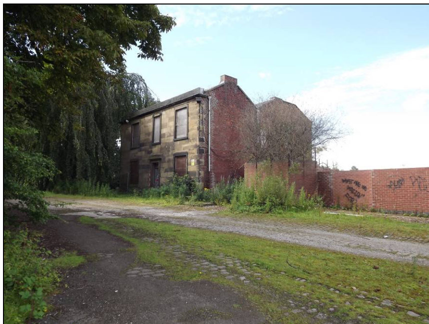
Plate 3: View looking south-west showing the main east elevation of Bramhall House
