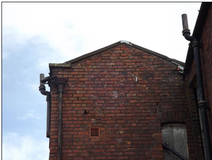
Plate 28: Detail of coping stones and kneeler, south elevation of addition
