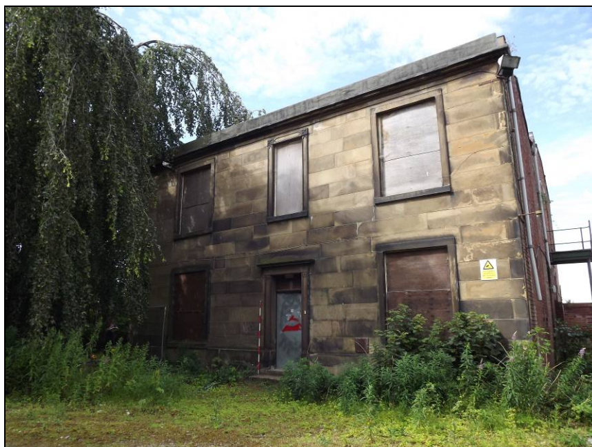
Plate 4: East elevation of Bramhall House
