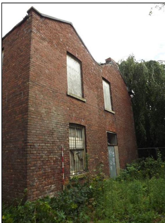
Plate 11: South elevation of Bramhall House
