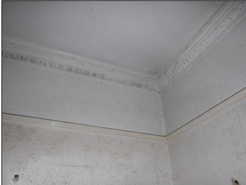
Plate 39: Detail of egg and dart coving, south-east ground floor room
