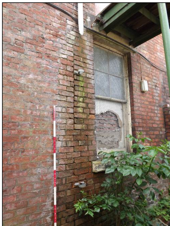
Plate 17: North elevation showing vertical construction break (in line with the white downpipe)
