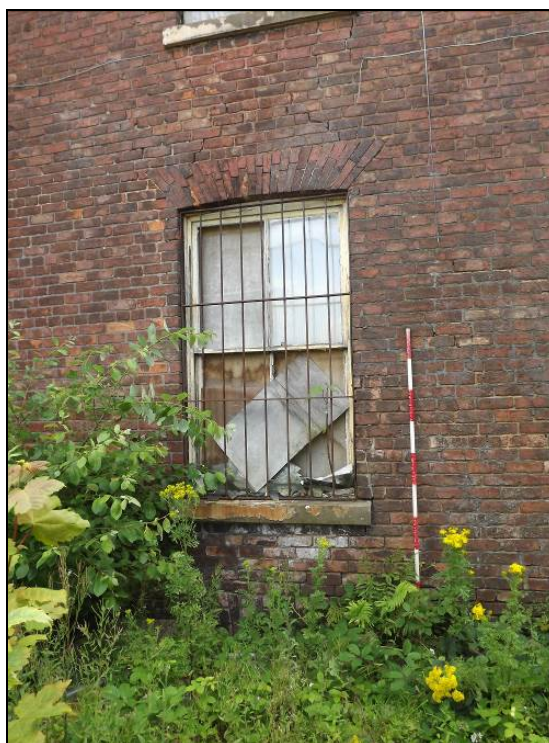
Plate 24: Detail of ground floor window, west elevation
