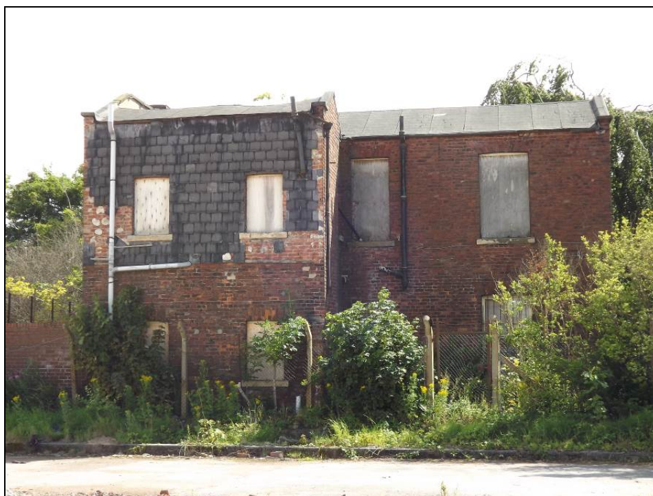
Plate 22: West elevation of Bramhall House showing the later (projecting) addition to left of the photograph
