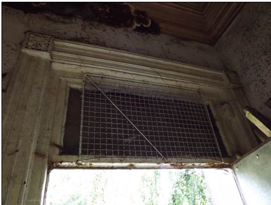
Plate 31: Detail of decorative door surround and fan light over main entrance as seen from the vestibule
