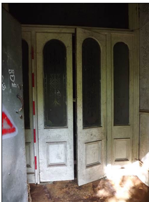
Plate 30: Detail of double doors to hallway (Scale = 2m)
