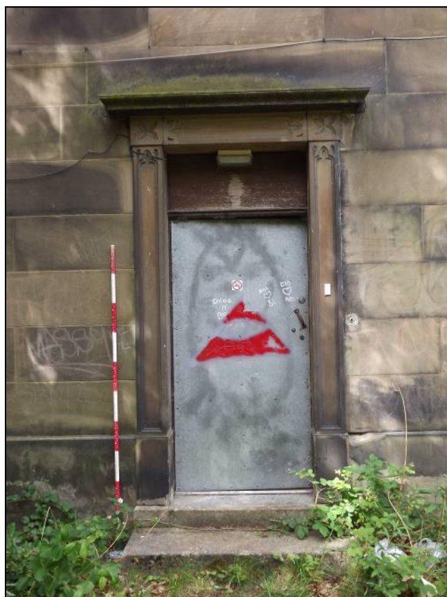
Plate 6: Detail of main entrance door surround, east elevation (Scale = 2m)
