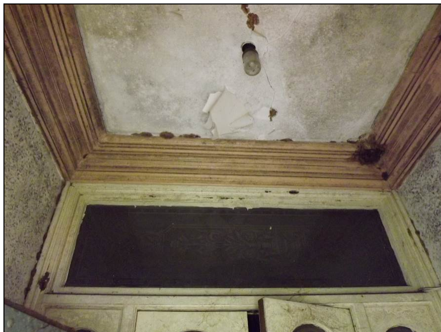
Plate 32: Detail of moulded coving in vestibule
