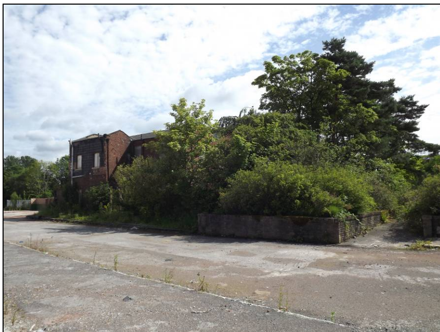
Plate 1: View looking east from the site of the former factory buildings showing the west elevation of Bramhall House
