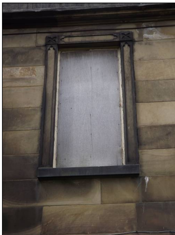
Plate 9: Detail of first floor central window, east elevation
