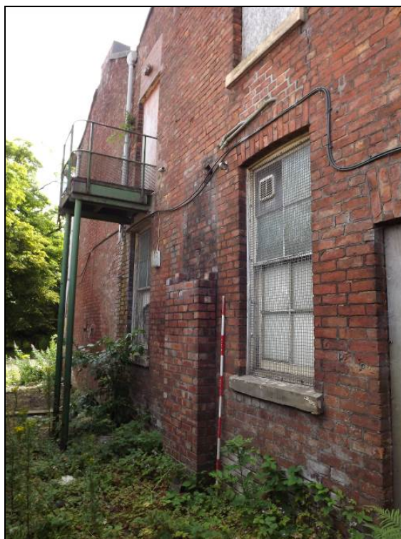
Plate 19: Ground floor window, north elevation (Scale = 2m)
