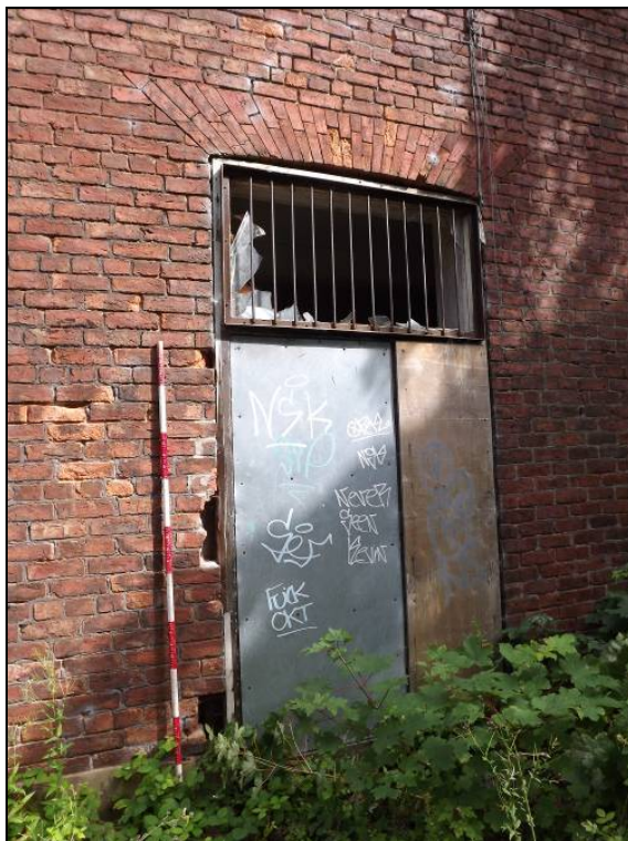
Plate 13: Detail of former French doors, south elevation
