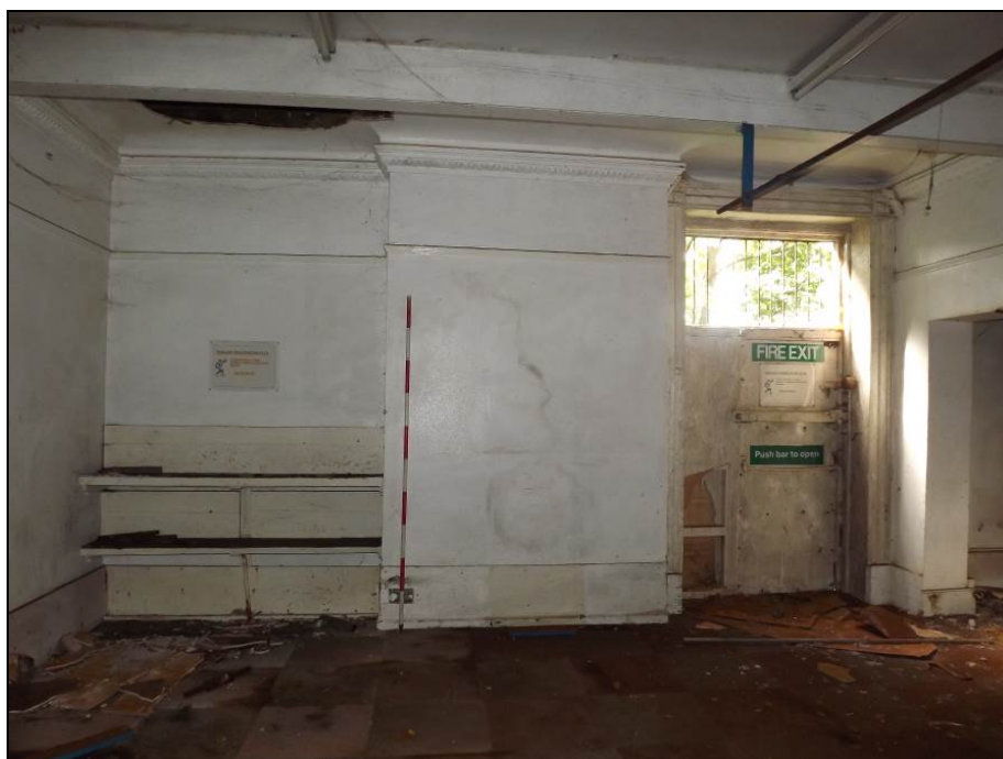
Plate 36: South wall of south-east room
