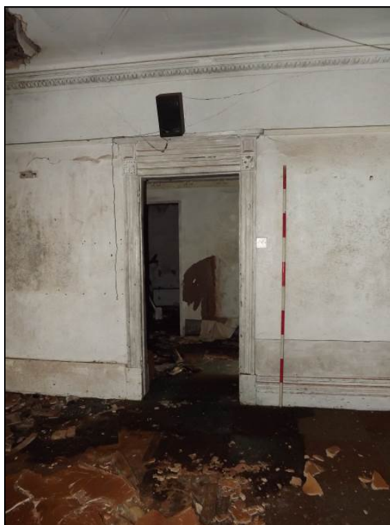
Plate 38: Detail of door surround, north wall of south-east room
