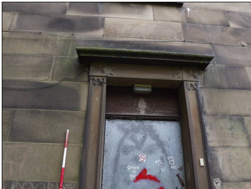
Plate 7: Detail of decorative door surround with simple projecting door hood, east elevation
