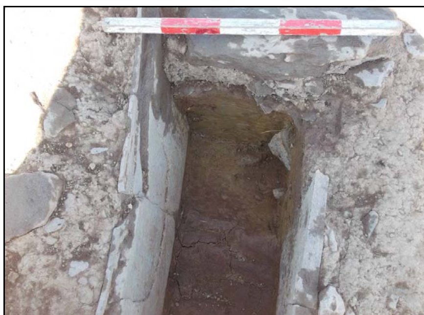
Plate 41: Culvert {1630}, looking southwest
