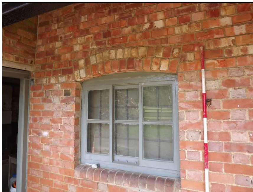
Plate 11: Tack Room window, south elevation
