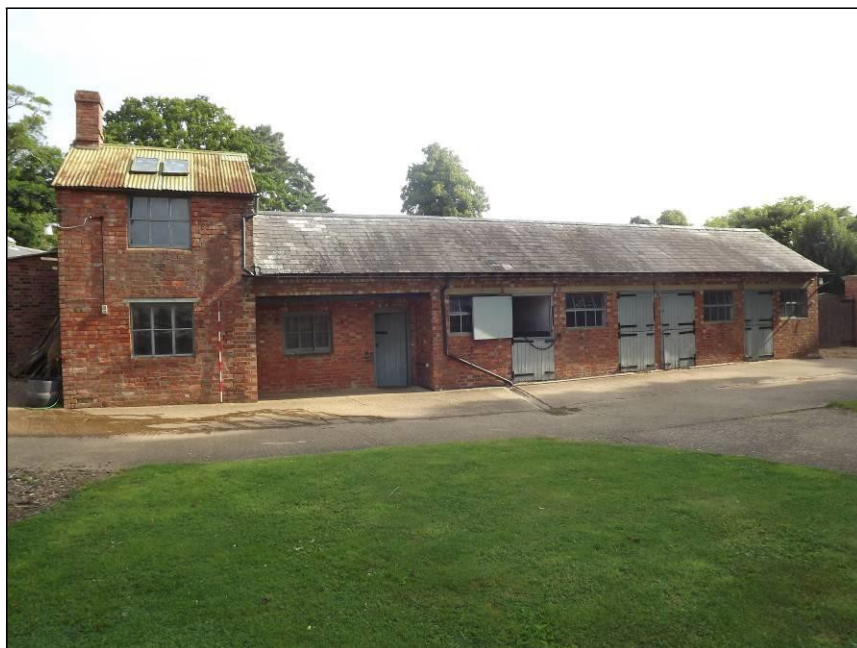
Plate 4: South elevation of the Loosebox Range
