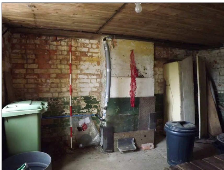
Plate 25: West wall of Store showing green and white colour scheme and former fireplace (Scale = 2m)
