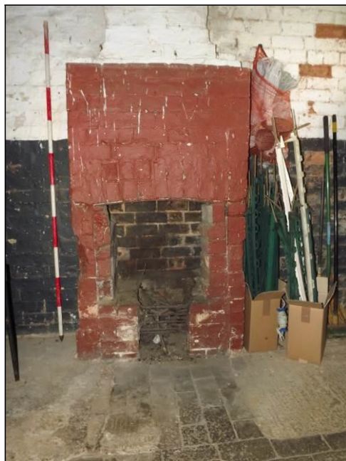
Plate 28: Detail of fireplace in Tack Room
