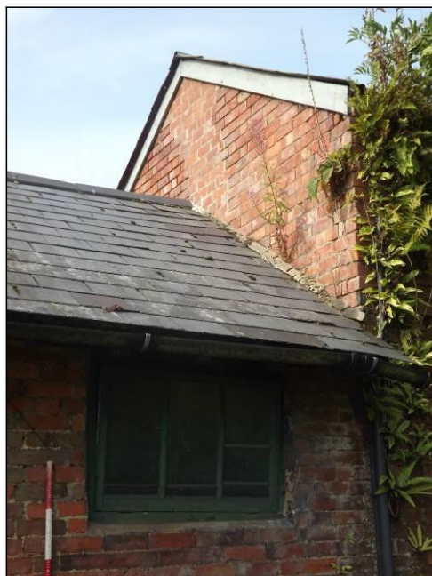
Plate 24: Scarring for the former flue, east gable of the two-storey section
