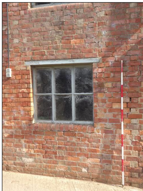
Plate 6: Detail of window in south elevation of two-storey section (Scale = 2m)
