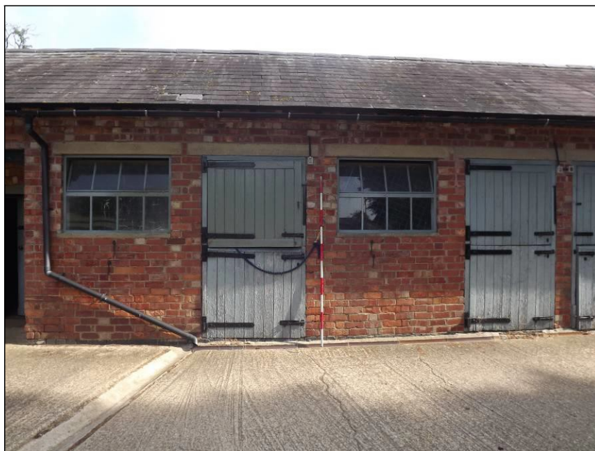
Plate 13: Detail of the loose box (stable) doors and windows, south elevation
