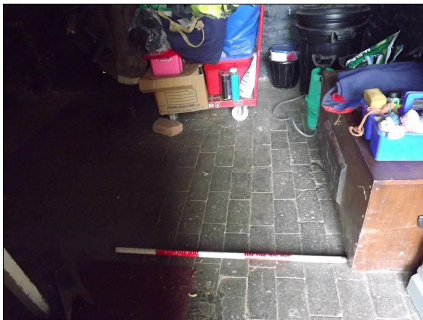
Plate 31: Detail of brick floor in Tack Room (Scale = 1m)
