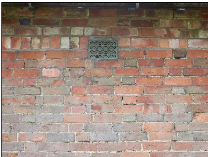
Plate 22: One of the decorative ventilation grilles, north elevation
