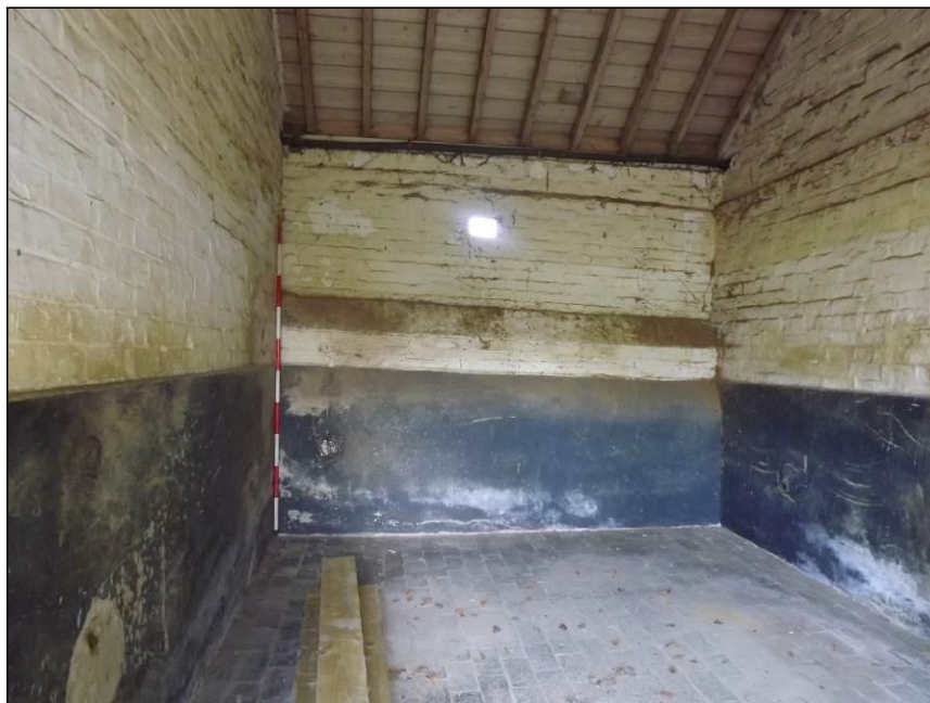
Plate 34: North wall of one of the loose boxes showing the earlier garden/boundary wall (Scale = 2m)
