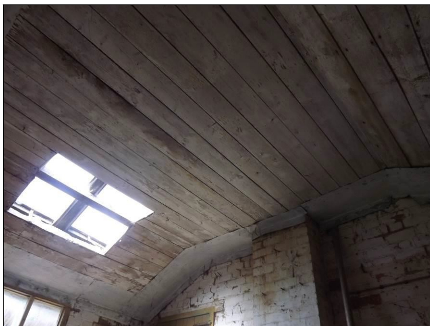
Plate 27: Wooden ceiling, first floor of Store
