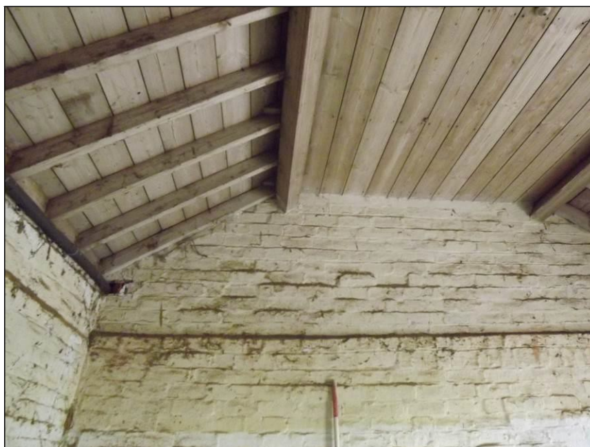
Plate 35: Detail of roof structure in the loose boxes
