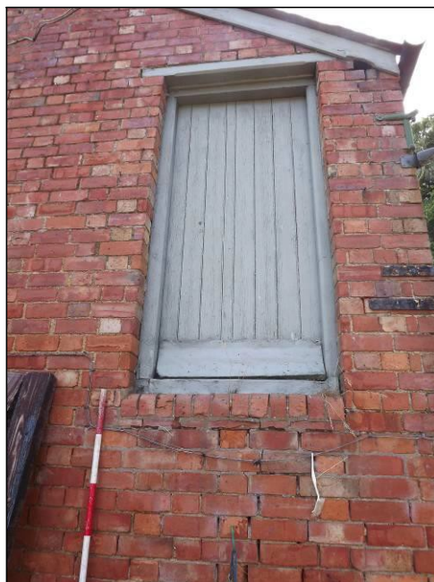
Plate 9: Detail of first floor doorway, west elevation
