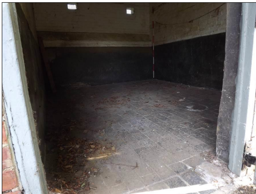
Plate 33: Detail of brick floor in Room 4
