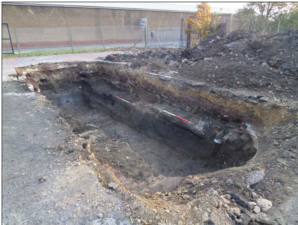
Plate 2: Overview of Trench. Looking east-north-east. 2 x 1m, 1 x 2m scales.
