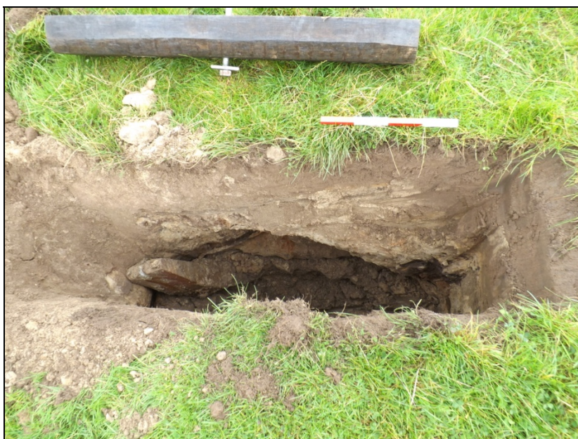
Plate 1: Pole 1. Trench for pole stay. Looking north-west. 0.40m scale
