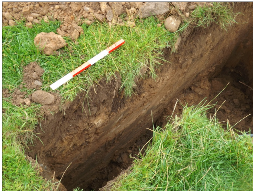
Plate 2: Pole 2. Trench for pole stay. Looking north-west. 0.40m scale
