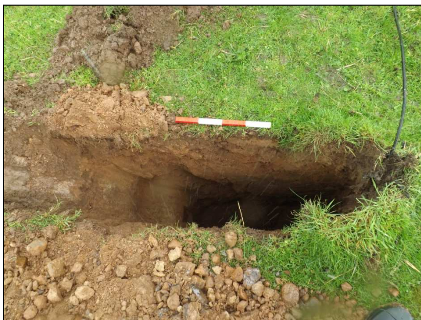
Plate 3: Pole 1. Trench for replacement pole. Looking north-west. 0.40m scale
