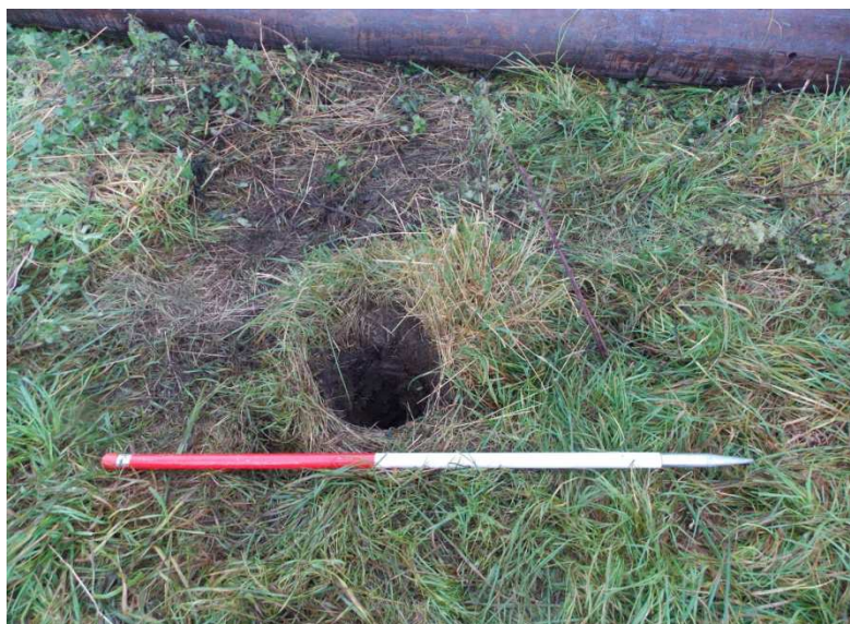
Plate 2: Original Foundation hole for pole 3
