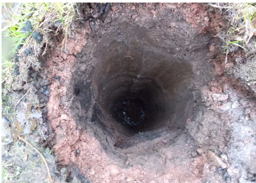
Plate 3: Foundation for pole 3 after re excavation.
