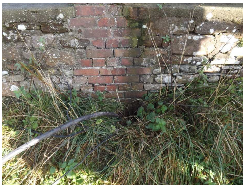
Plate 1: Original foundation for pole 1
