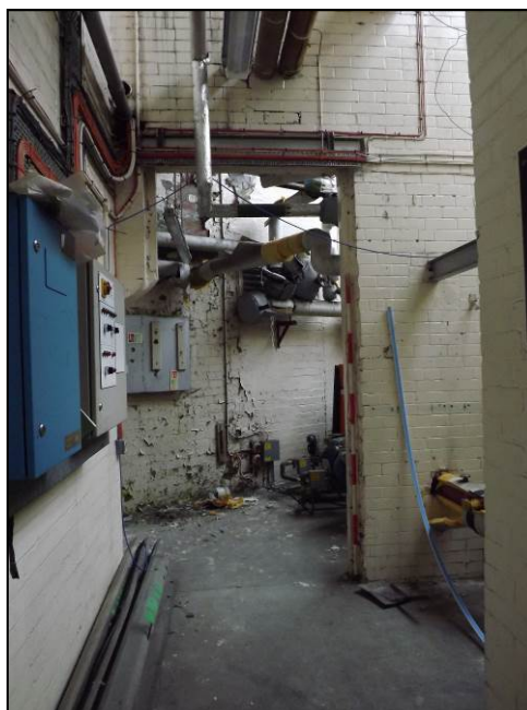
Plate 55: Boiler Room in northern corner of building
