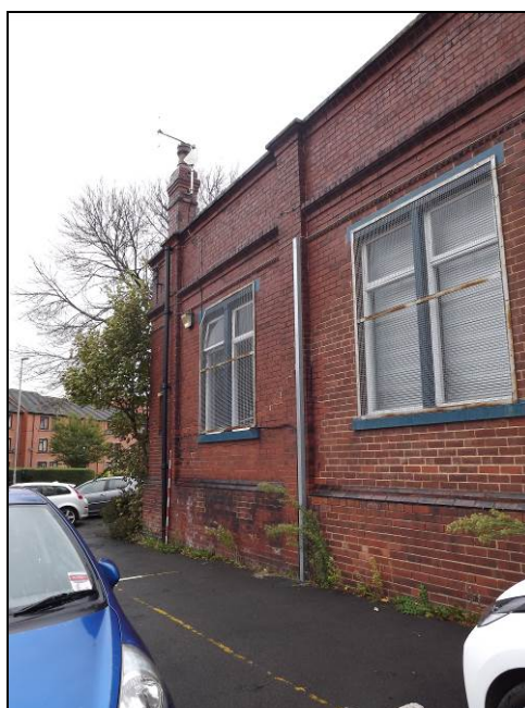
Plate 30: West end of south-west elevation showing two large windows
