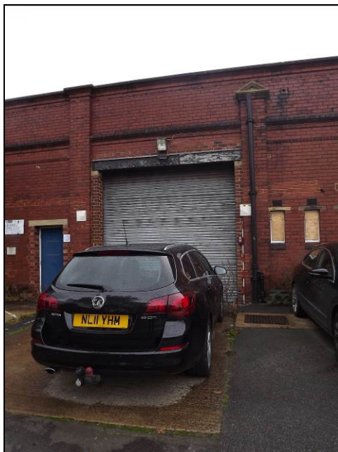
Plate 27: South-west elevation of original factory showing inserted doorways (Scale = 2m)
