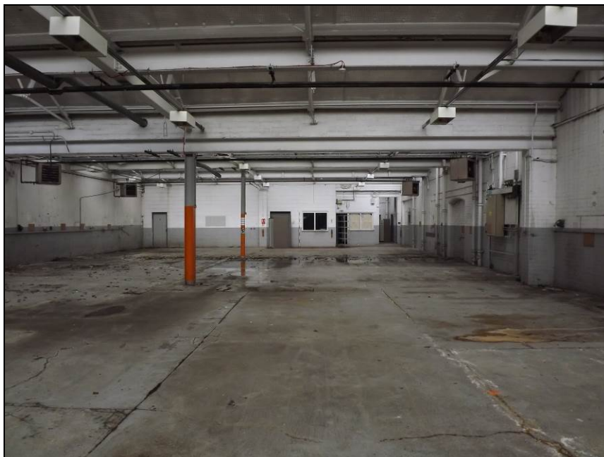
Plate 45: View looking south-west showing the interior of the c.1930 addition
