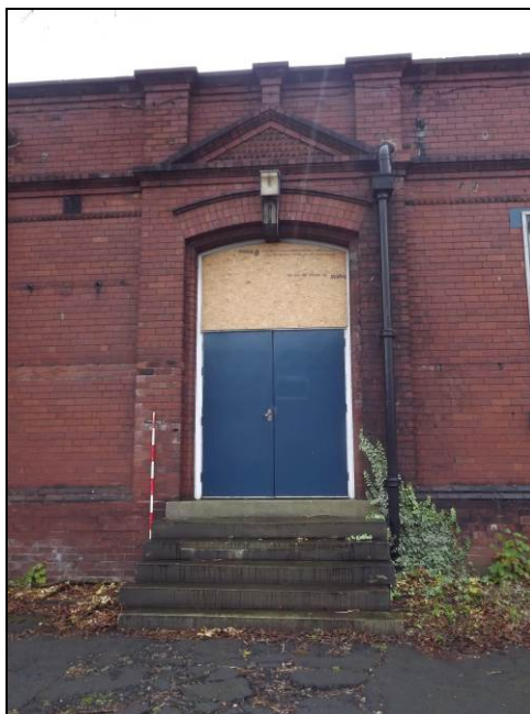
Plate 12: Detail of original doorway, north-west elevation (facing onto Belle Vue Road)
