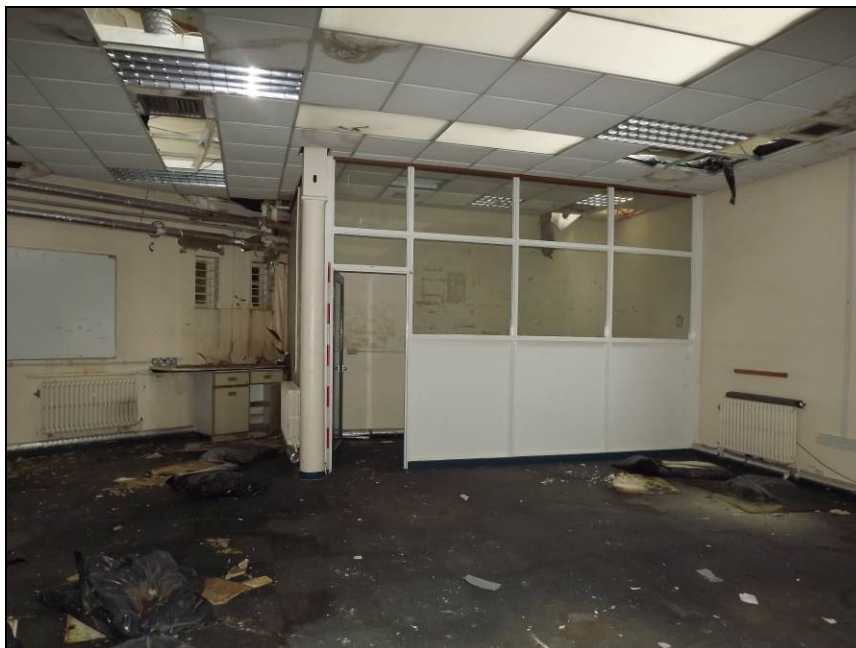
Plate 54: Room G12 showing column incorporated into an office partition (Scale = 2m)
