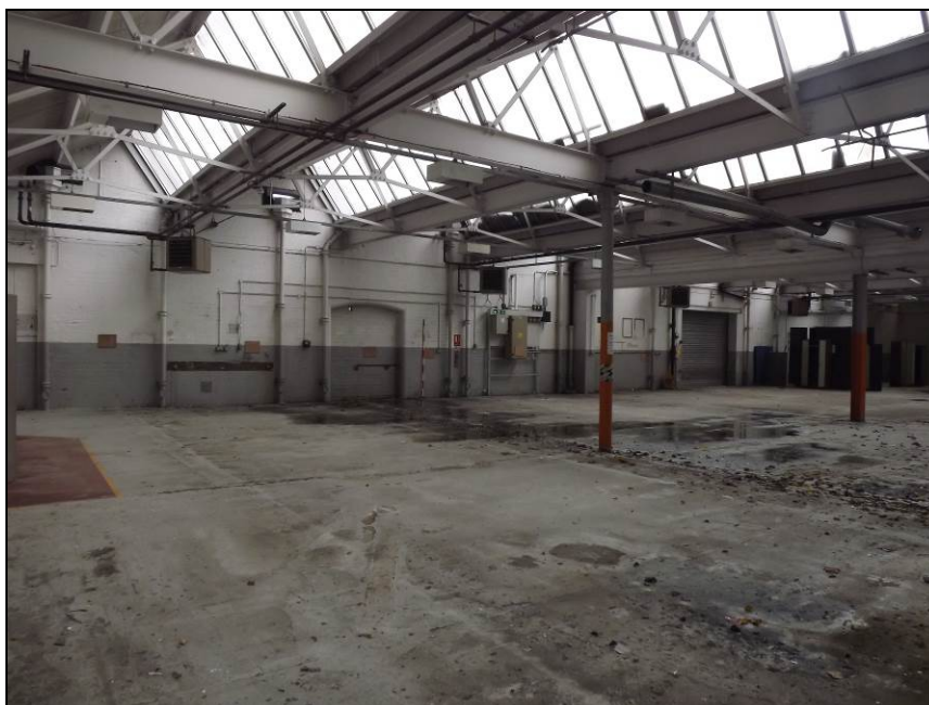
Plate 51: North-west wall of the c.1930 addition
