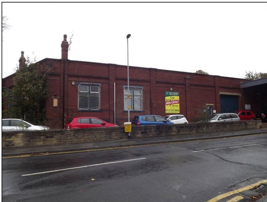
Plate 29: West end of south-west elevation
