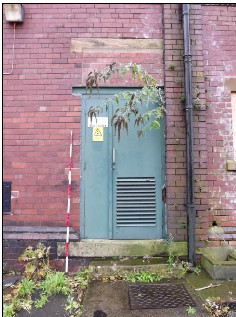
Plate 17: Detail of inserted electricity substation door, north-west elevation
