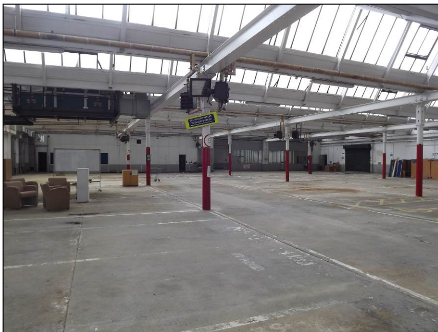
Plate 31: View looking east showing the interior of the main former factory floor
