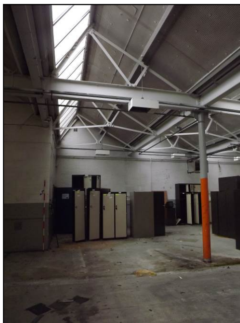
Plate 47: Detail of roof structure, c.1930 addition
