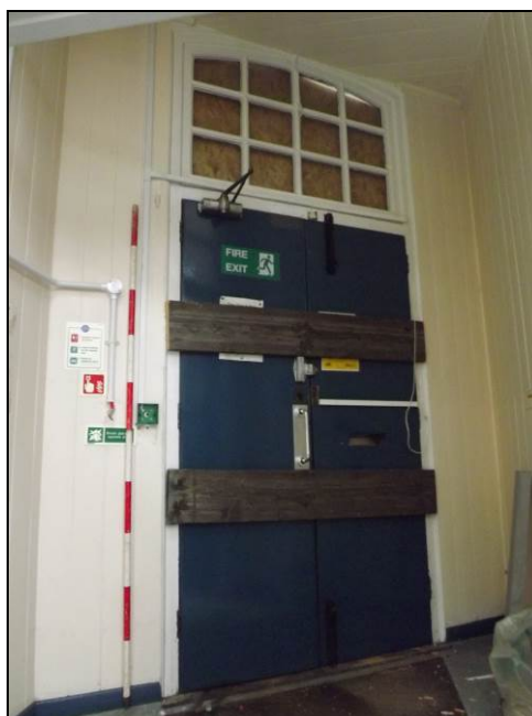
Plate 58: Original doorway, north-west elevation (Scale = 2m)
