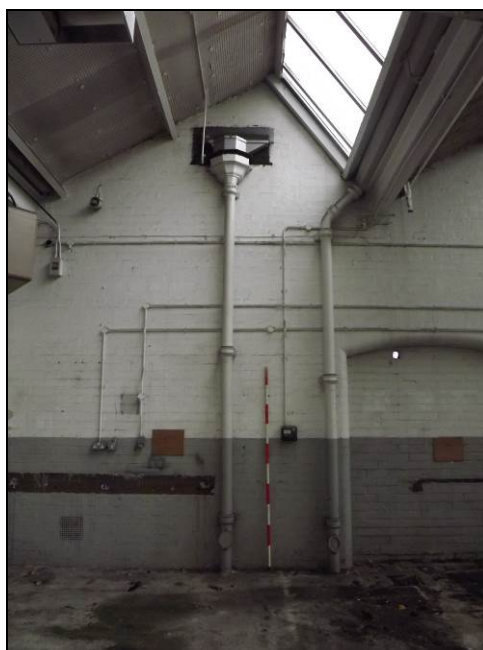
Plate 51: Detail of rainwater hopper and downpipe, north-west wall of c.1930 addition
