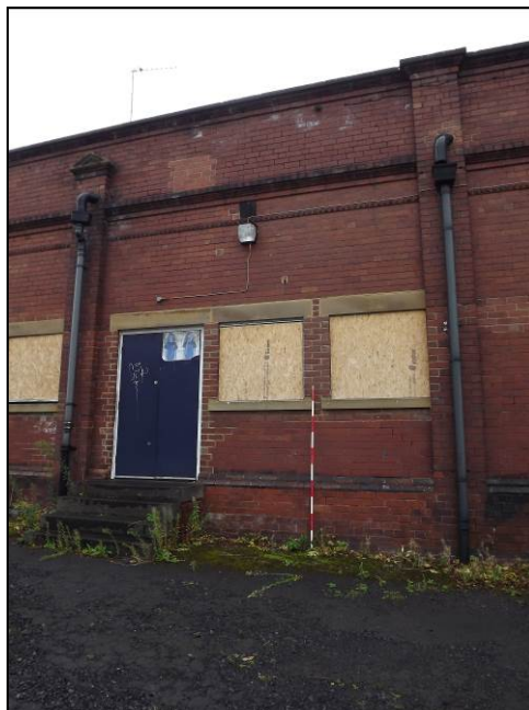
Plate 15: Detail of inserted door and windows, north-west elevation (Scale = 2m)
