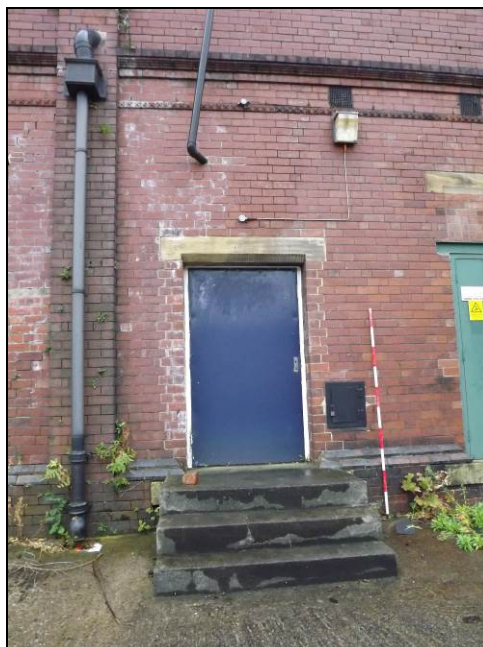
Plate 16: Inserted doorway, north end of the north-west elevation
