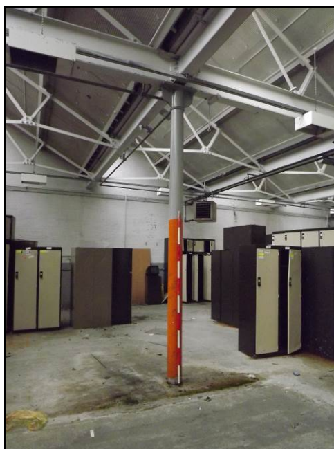
Plate 46: Detail of one of the round columns in the c.1930 addition (Scale = 2m)
