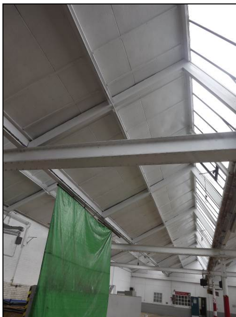
Plate 34: Detail of one of the north-lights, main former factory floor
