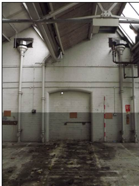
Plate 54: Original doorway (now infilled), north-west wall of c.1930 addition
