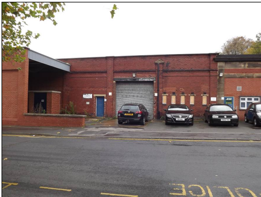
Plate 25: South-west elevation showing the difference between the original factory (left of photograph) and the c.1930 addition (right of photograph)
