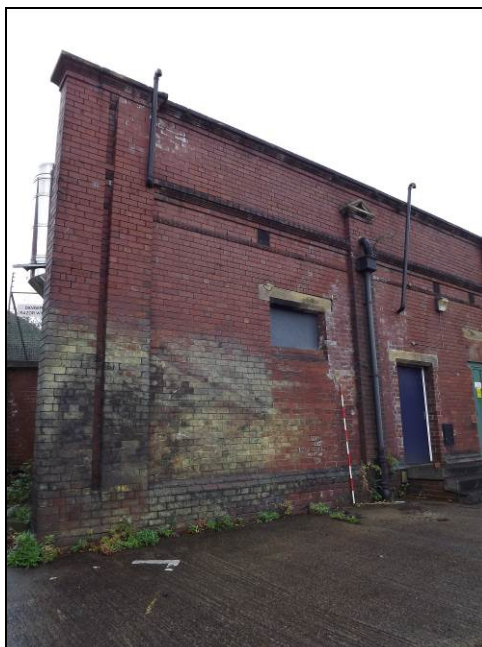
Plate 18: North end of north-west elevation showing possible former doorway converted to a window (Scale = 2m)
