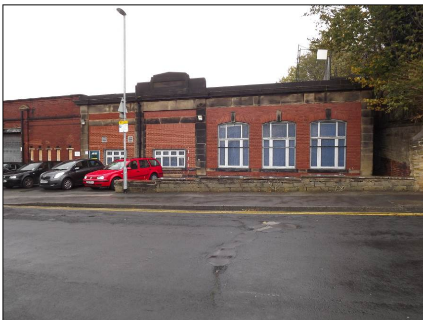
Plate 22: Eastern end of the south-west elevation showing separate construction phase
