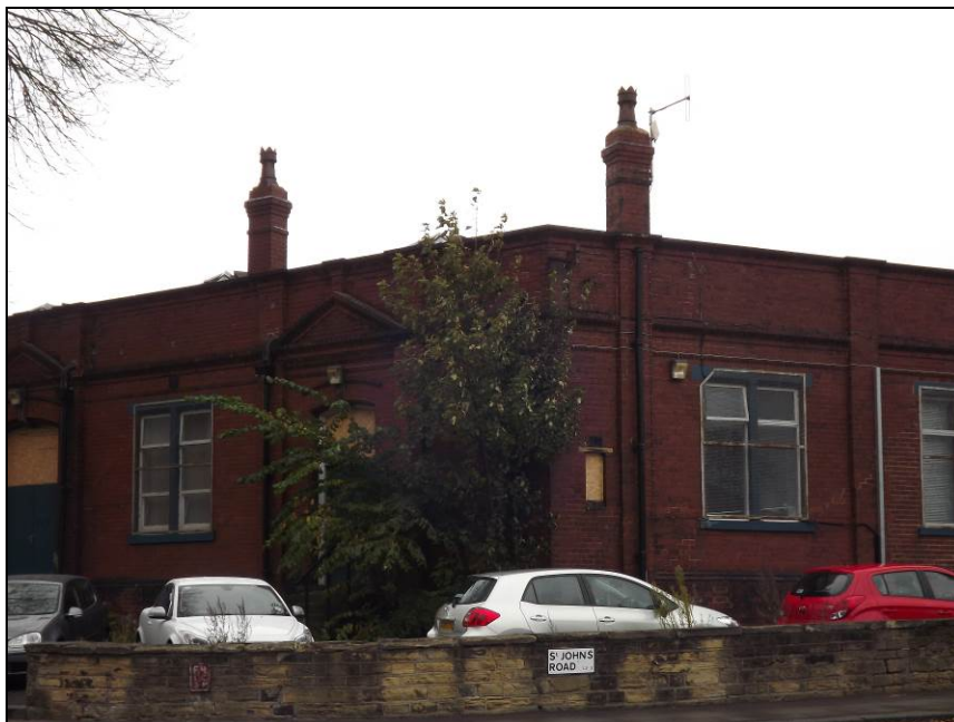
Plate 19: Detail of the two chimneys, corner of north-west and south-west elevations
