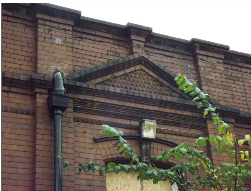
Plate 14: Detail of brick pediment over original doorway, north-west elevation
