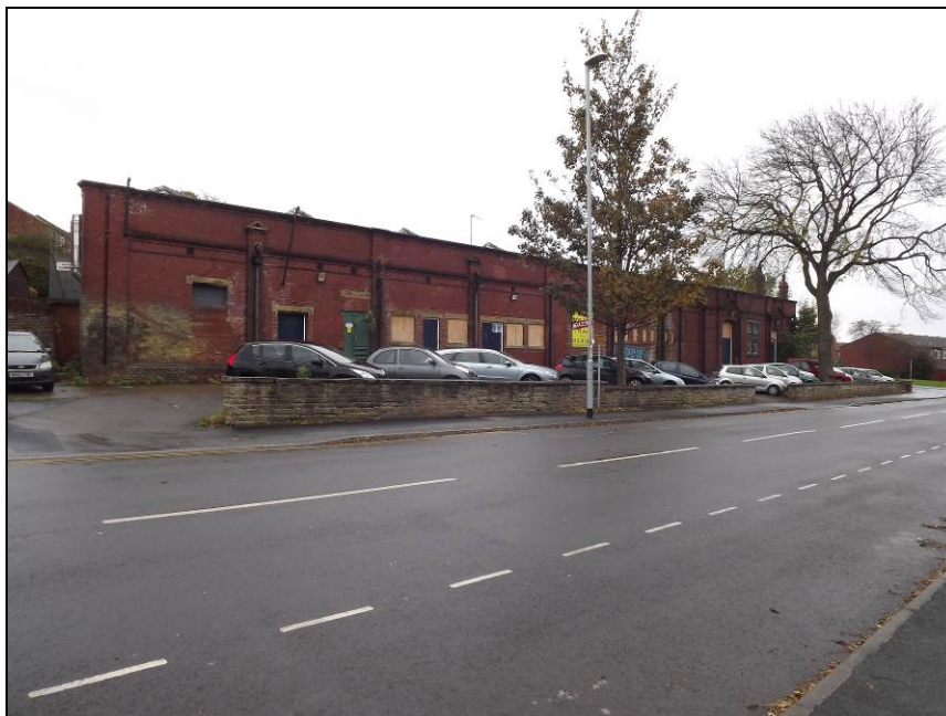
Plate 5: North-west elevation onto Belle Vue Road
