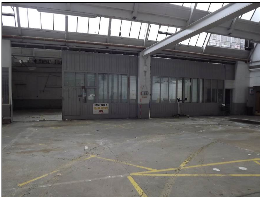
Plate 42: Detail of inserted sliding doors, north-east wall of main former factory floor
