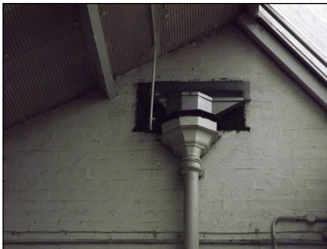
Plate 52: Detail of rainwater hopper, north-west wall of c.1930 addition
