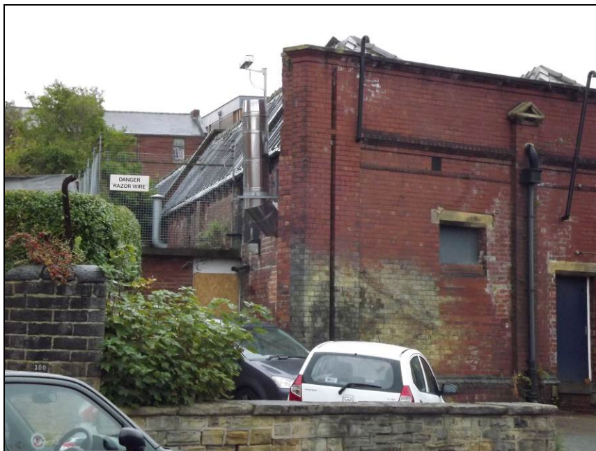
Plate 9: Detail of roof structure, north end of north-west elevation
