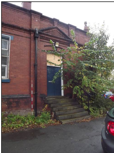
Plate 13: Southernmost original doorway, north-west elevation
