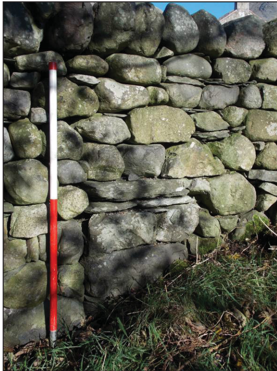
Plate 7: Feature 4, in Wall G, facing north west
