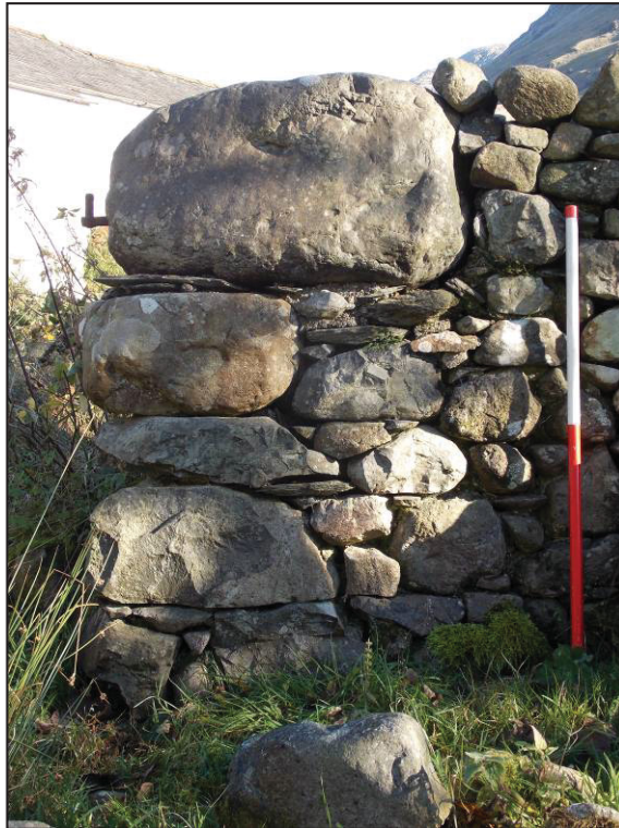
Plate 11: Feature 9 (gate pin) in Wall G, facing east north east
