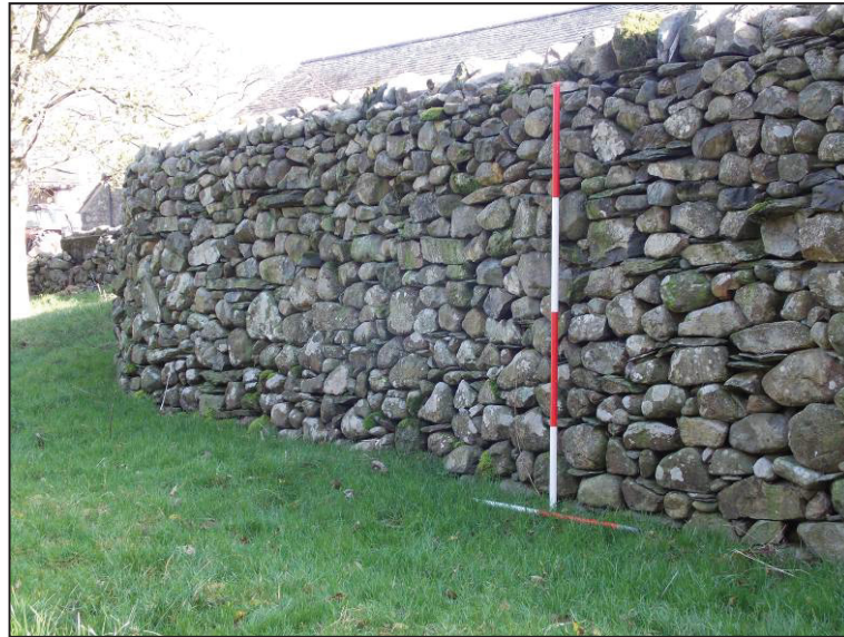
Plate 14: Wall J, facing north east
