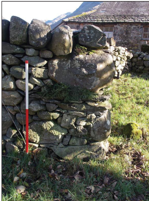
Plate 9: Feature 6 (gate pin), in Wall F, facing north west
