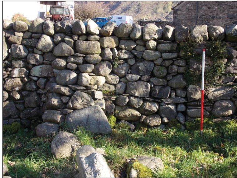
Plate 10: Features 7 (right) and 8 (left) in Wall G, facing east
