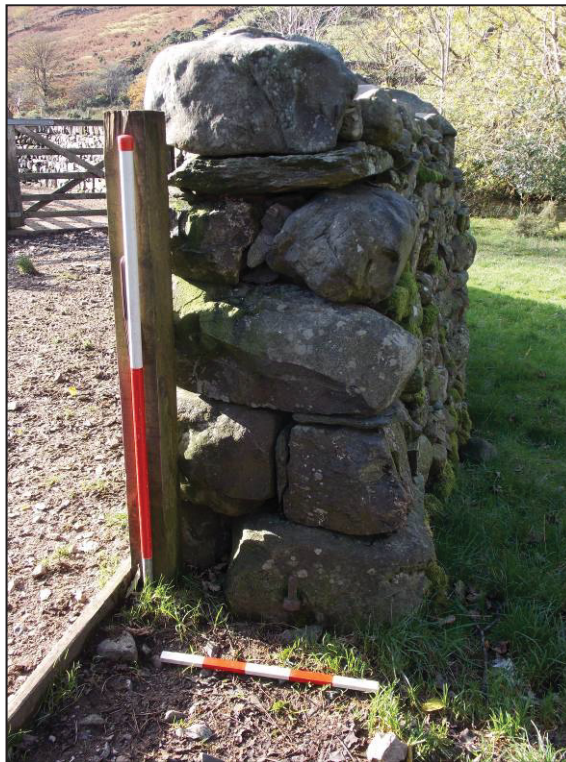
Plate 15: Feature 3 in Wall J, facing west south west
