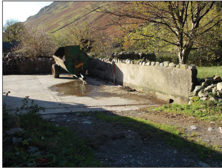
Plate 12: Modern breezeblock and concrete rendered wall, facing west south west
