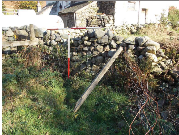
Plate 3: Wall C, northern area, facing west
