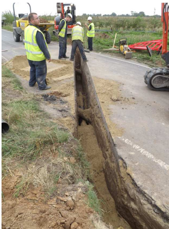
Plate 6: Excavations across Cottington Road after backfilling.
