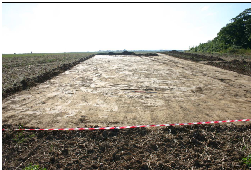
Plate 1: Access Road and compound area. 1m scale.
