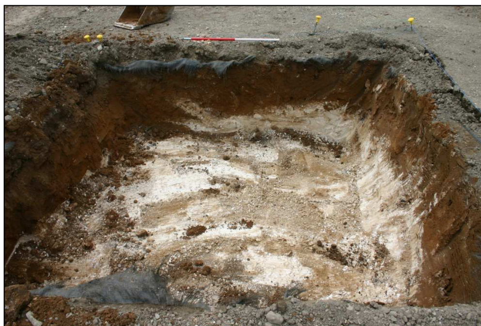
Plate 2: Cable Pit within eastern most substation. 1m scale.
