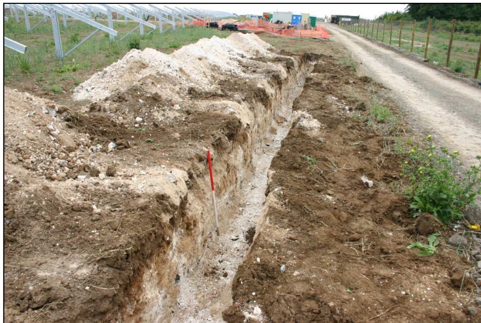
Plate 3: Purple (1.2m deep) cable trench. 1m scale.
