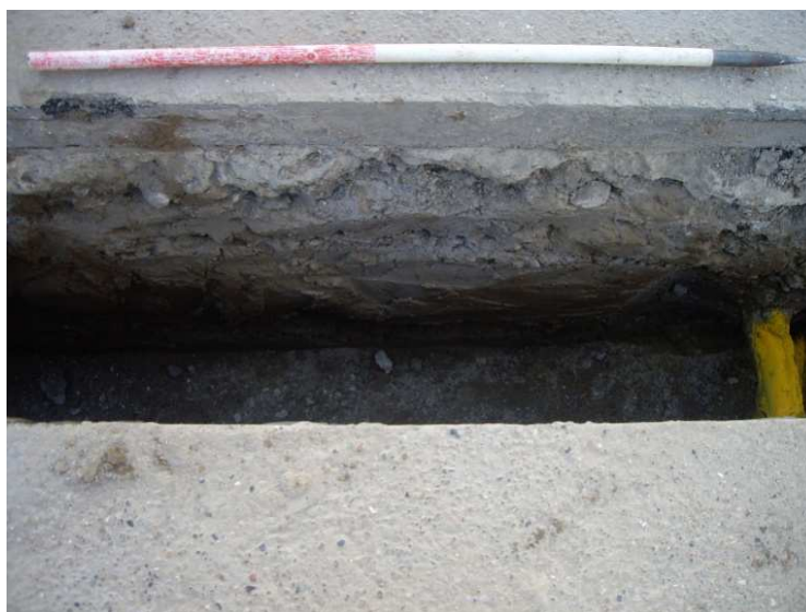
Plate 7: Section of excavation through road surface. 1.0m scale
