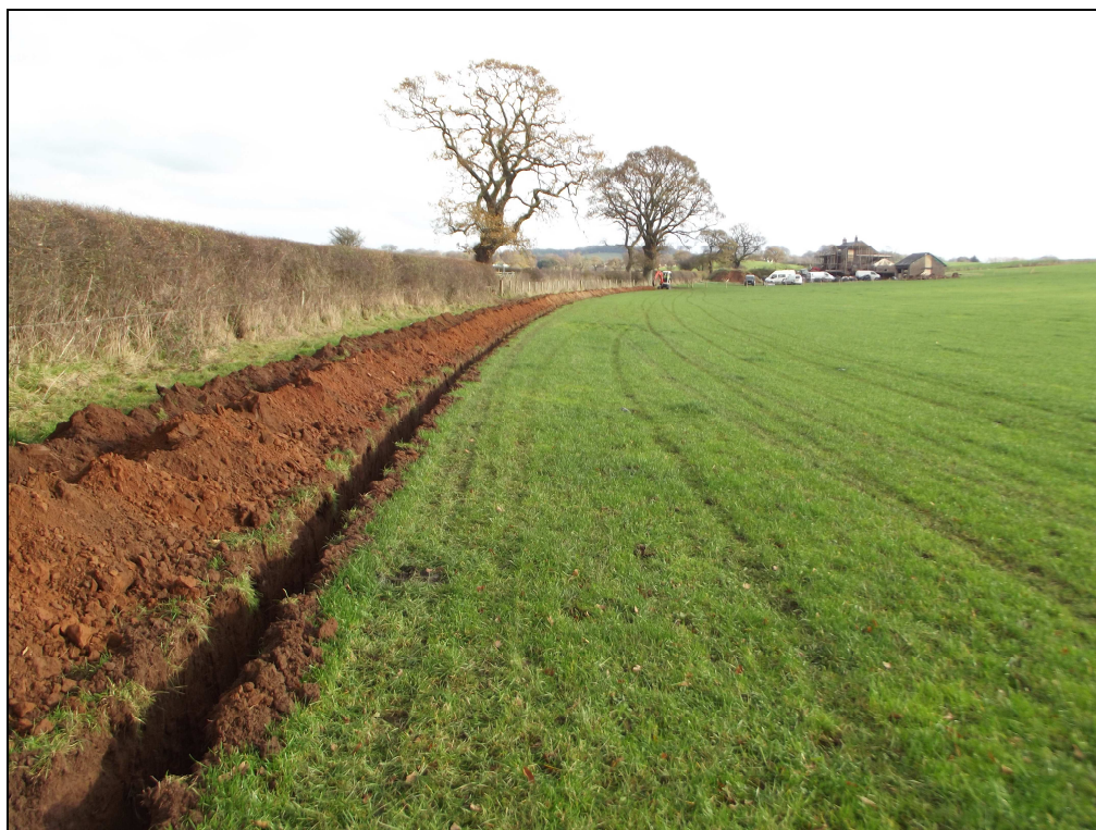
Plate 2: Cable trench looking east towards new dwelling
