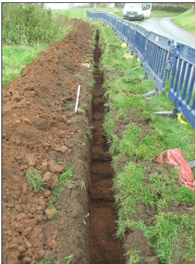
Plate 1: Cable trench at western end of route looking west
