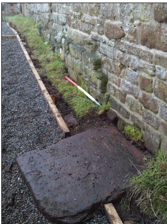
Plate 5: Sandstone slab incorporated into line of path (note earlier wall phase projecting adjacent to scale), facing north-west
