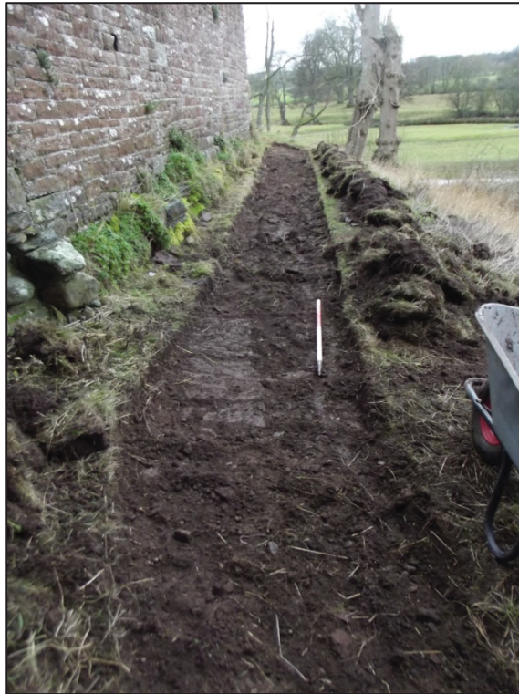
Plate 3: Two stone slabs observed towards eastern extent of upper path, north of northern surviving curtain wall, facing west
