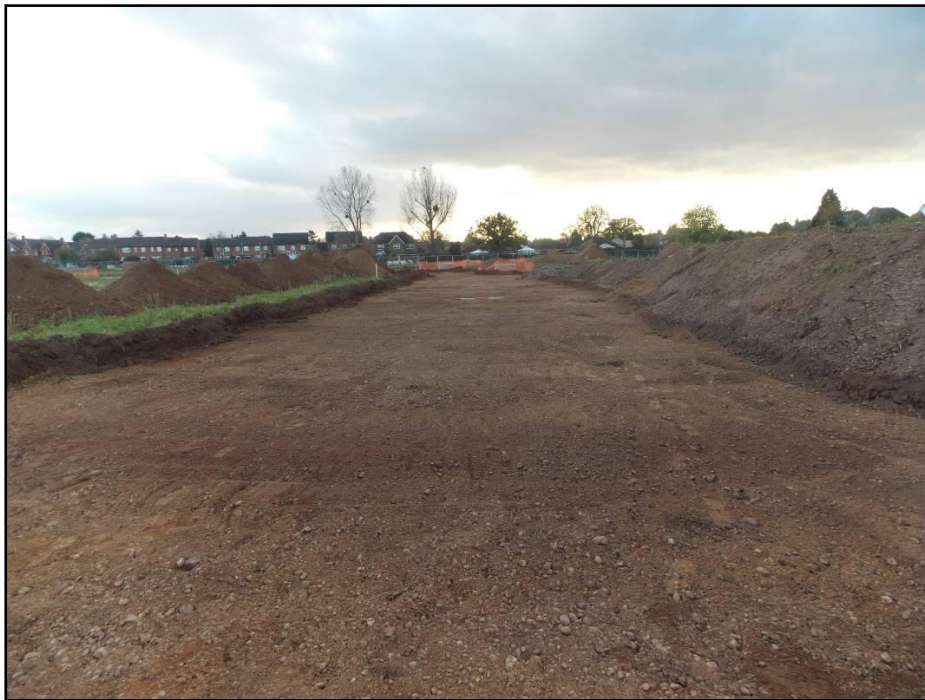
Plate 8: Road 3, looking southwest
