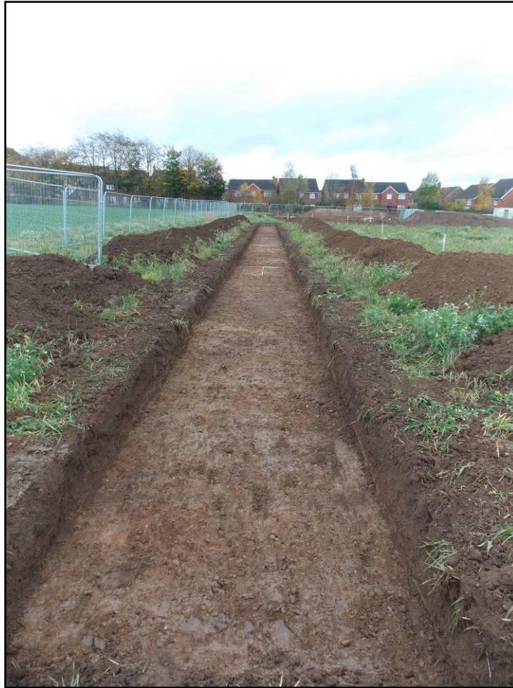
Plate 16: Trench 7, looking southwest
