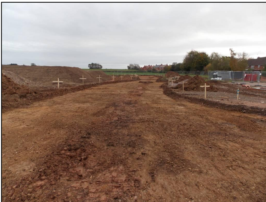
Plate 7: Road 2 – showing line of the sewerage pipe, looking southeast
