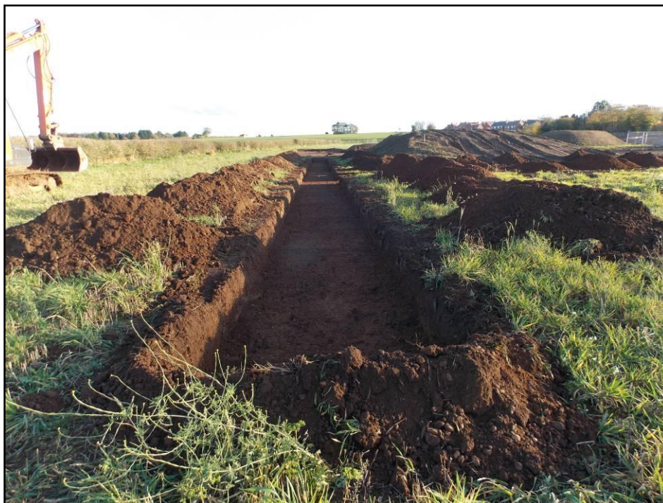
Plate 13: Trench 3, looking southeast
