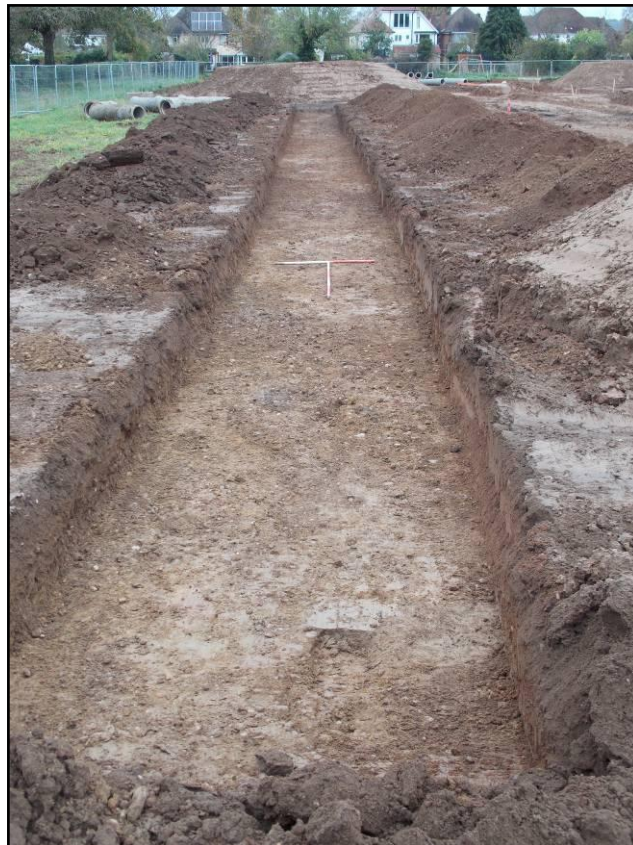
Plate 19: Trench 10, looking northwest
