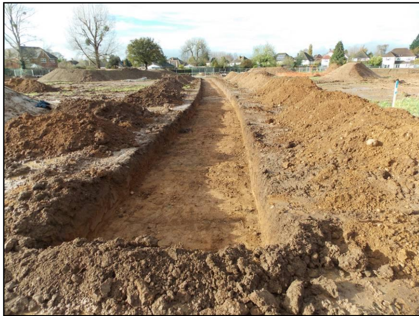
Plate 21: Trench 11, looking west northwest
