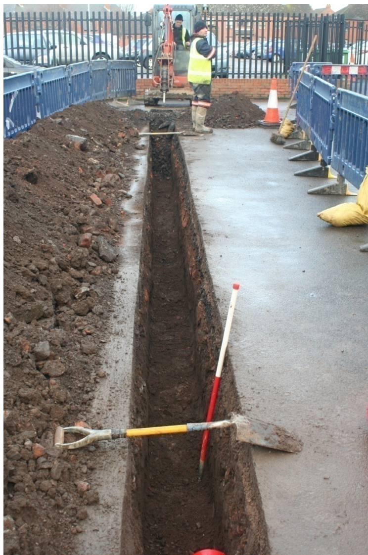
Plate 2: Service trench, showing the depth of the excavation (1m scale).
