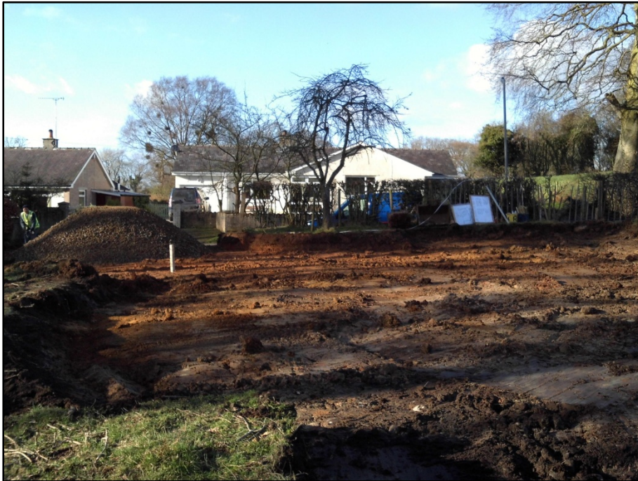
Plate 2: Topsoil strip looking north
