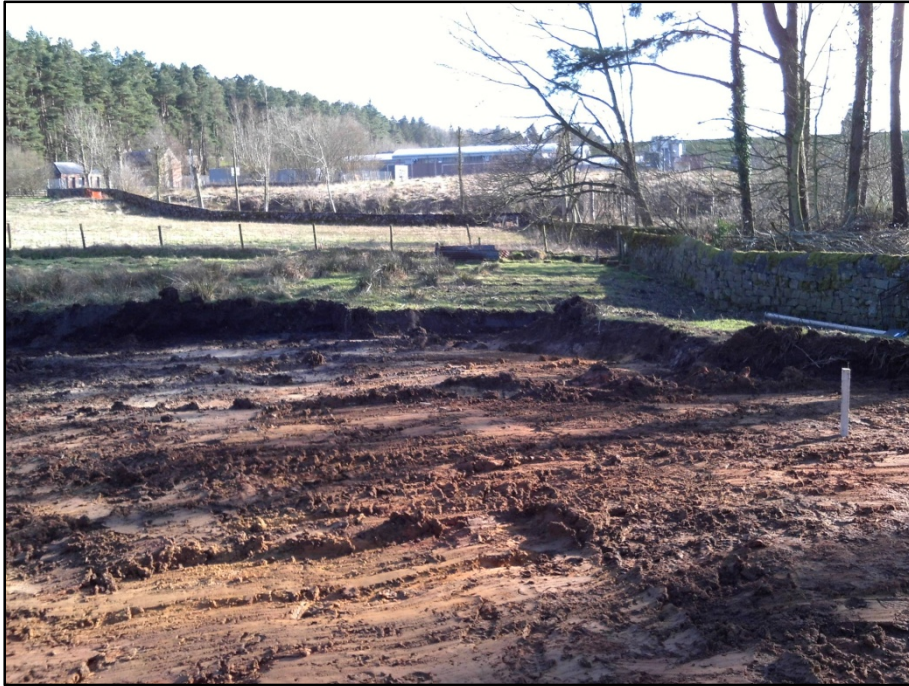
Plate 1: Topsoil strip looking south
