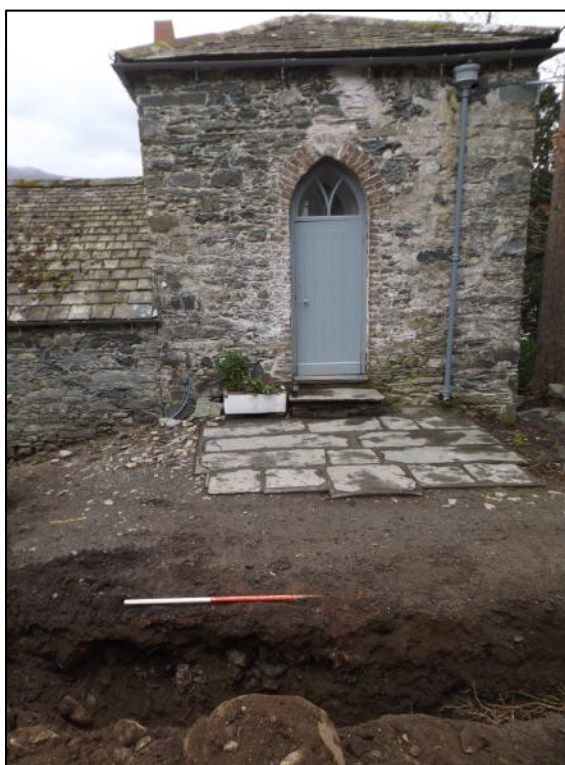
Plate 19: Made ground adjacent to church tower door (facing north-east)
