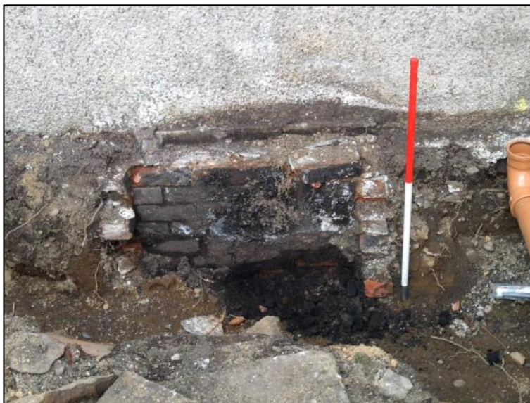
Plate 21: Removed brick structure from the north-west side of the battery house (facing south-east)
