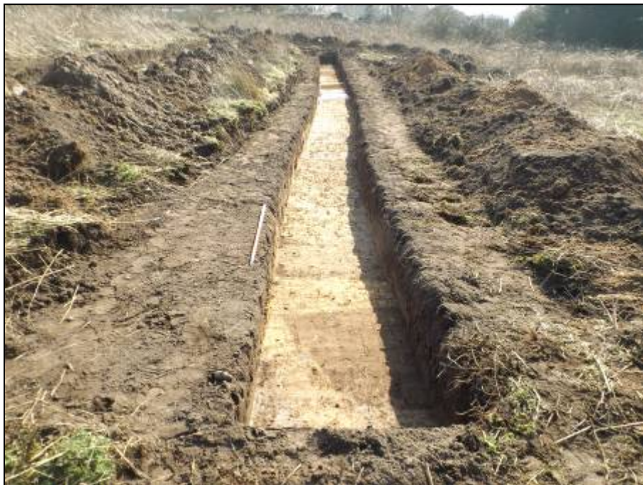
Plate 10: Trench 10, facing south south-east
