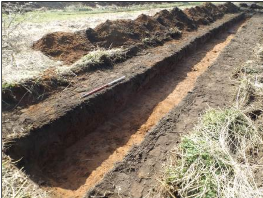
Plate 2: Trench 2, facing south south-west
