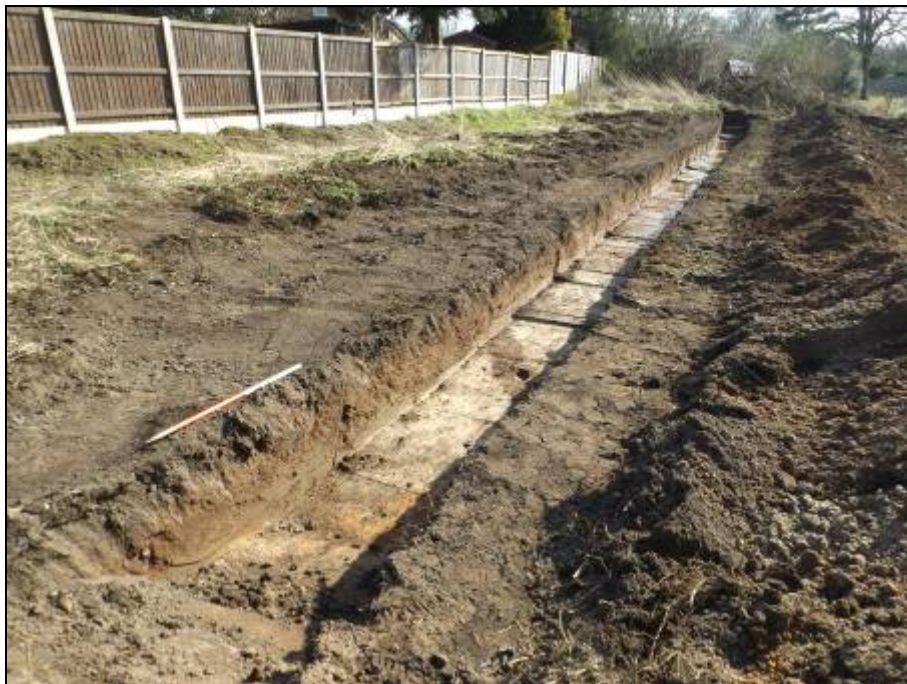
Plate 12: Trench 12, facing south south-east
