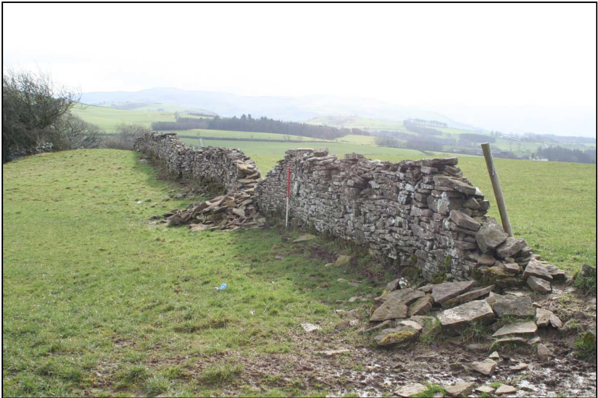
Plate 1: drystone Wall south-east of Bridekirk.
