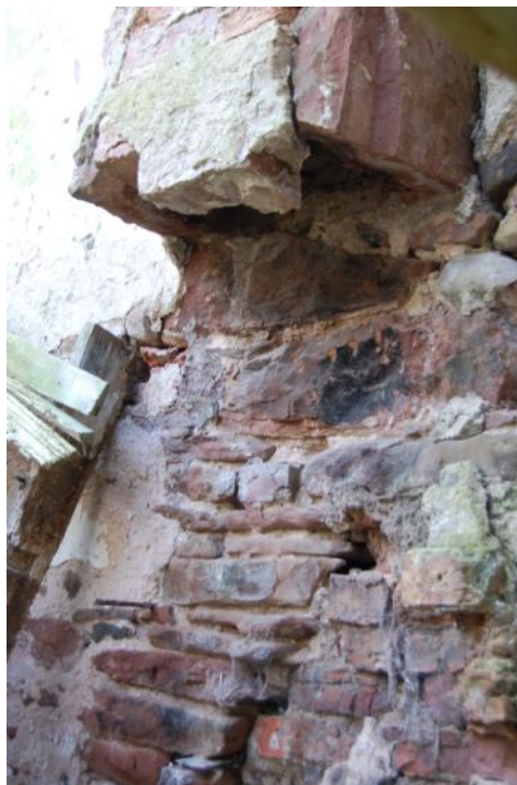
Plate 18: Base of flue in structure 5a, Unit 5
