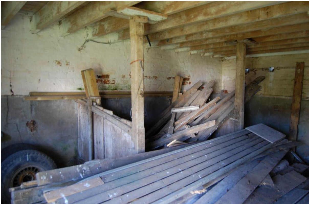
Plate 16: Southern room of structure 5b showing possible 19 th century stalls, Unit 5
