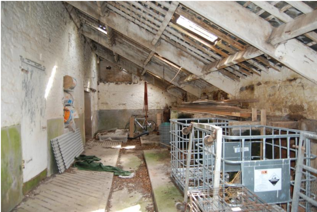
Plate 9: Interior of cat slide roof of byre, Unit 4
