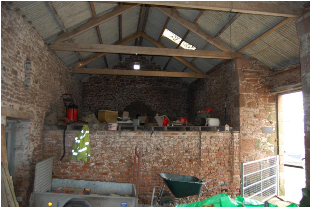
Plate 3: Brick partition wall within barn section of Unit 4
