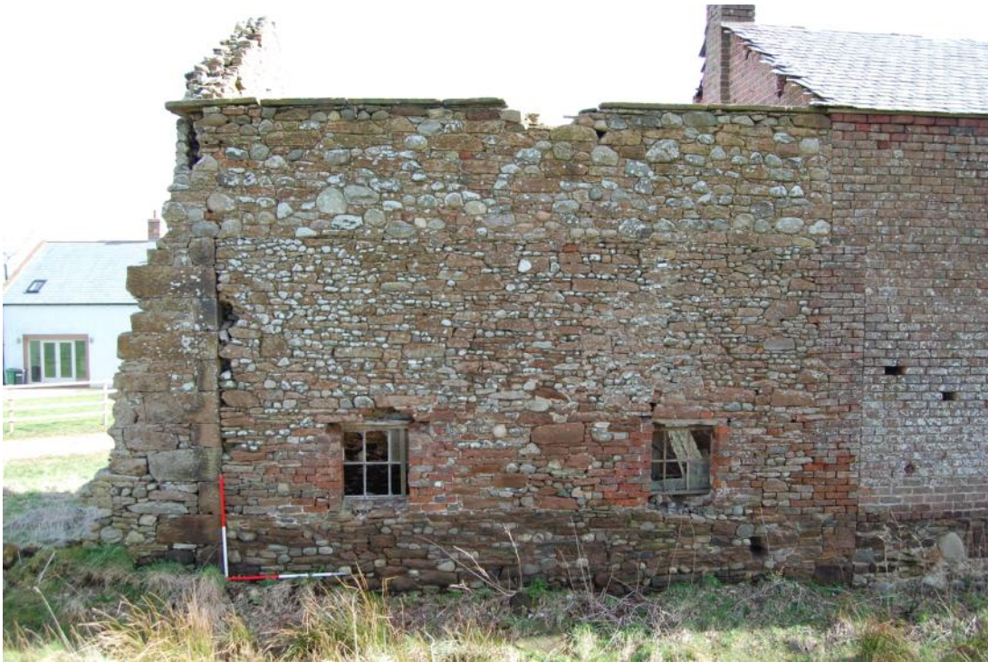
Plate 19: Western elevation to structure 5a, Unit 5
