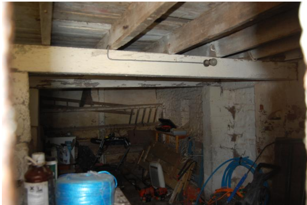
Plate 4: Interior of northern portion of barn Unit 4
