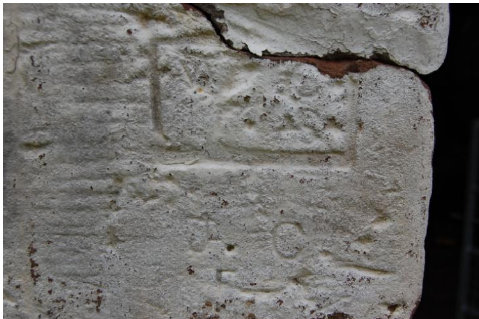
Plate 6: Graffiti on porch of barn of Unit 4
