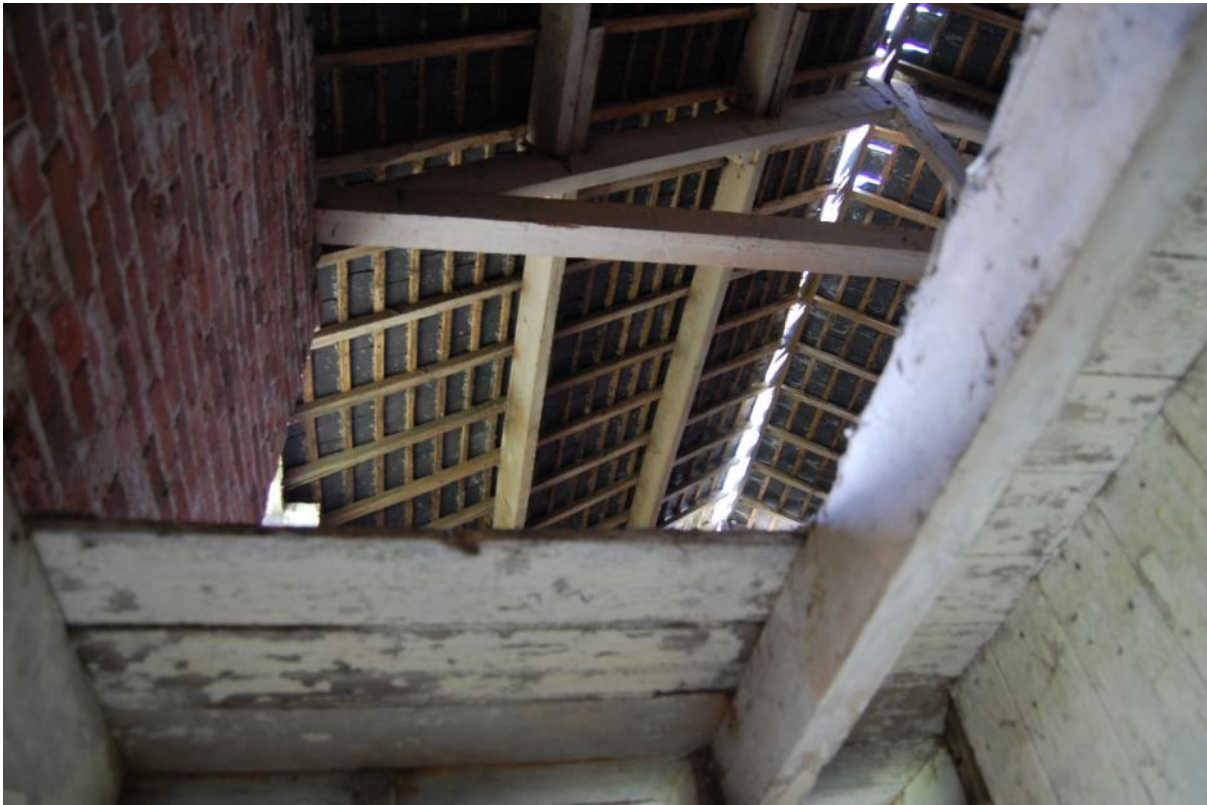
Plate 17: Interior of roof of structure 5b, Unit 5
