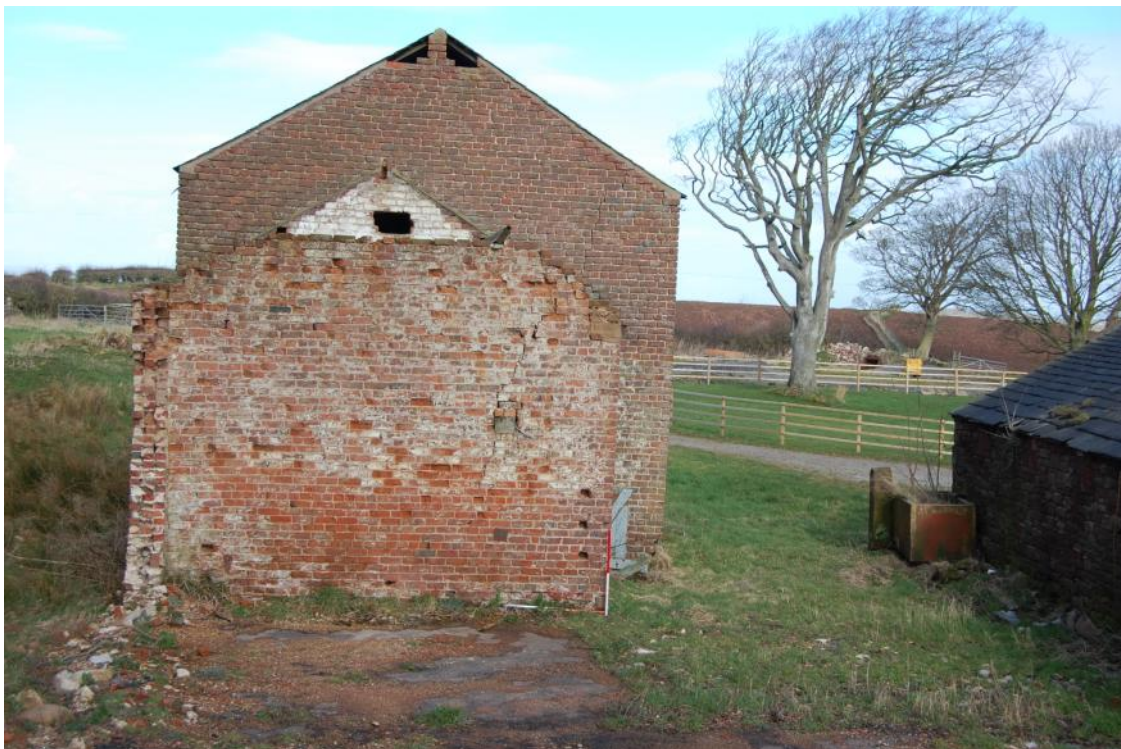
Plate 14: Foundations of building to the south of structure 5c, Unit 5
