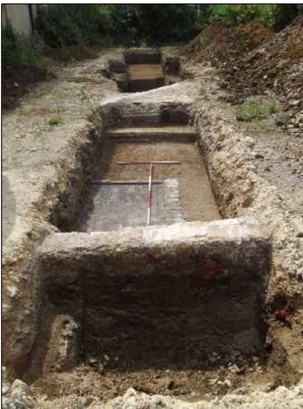
Plate 2: Trench 1; (facing southeast; 1m and 2m scales)
