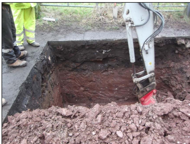
Plate 10: Natural revealed in Drill Pit 1, facing north
