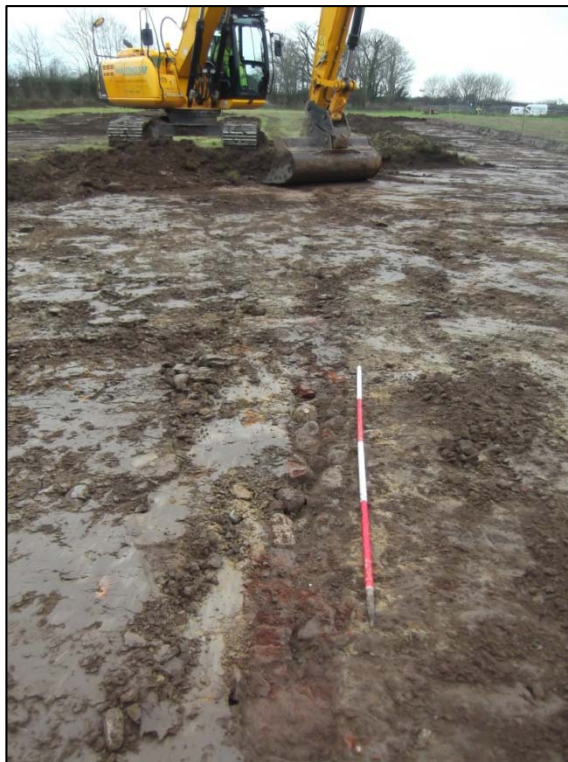
Plate 6: Second northernmost field drain, facing west-south-west
