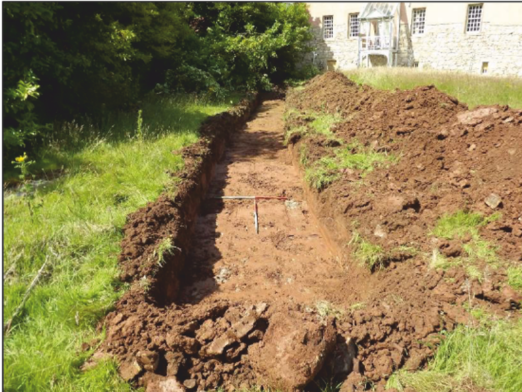
Plate 12: Trench 6, looking northeast
