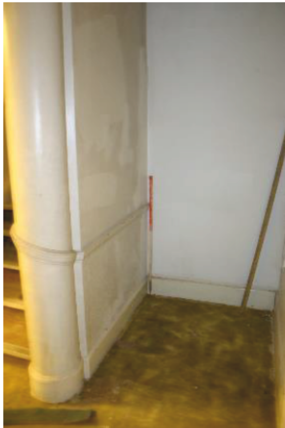
Plate 22: R 27, blocked up entrance to tunnel.
