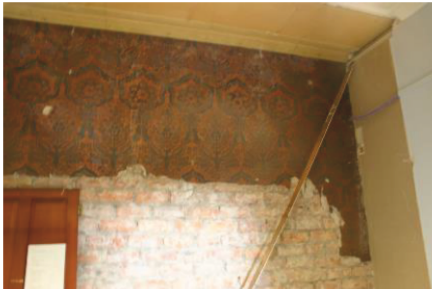
Plate 12: R 10, detail of wall covering.
