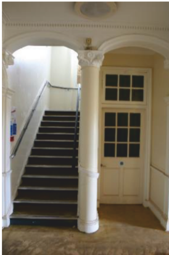
Plate 7: R 1, detail of staircase.
