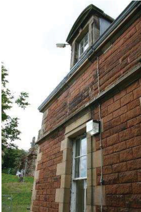
Plate 8: Detail East elevation, area of old staircase, are of old staircase
