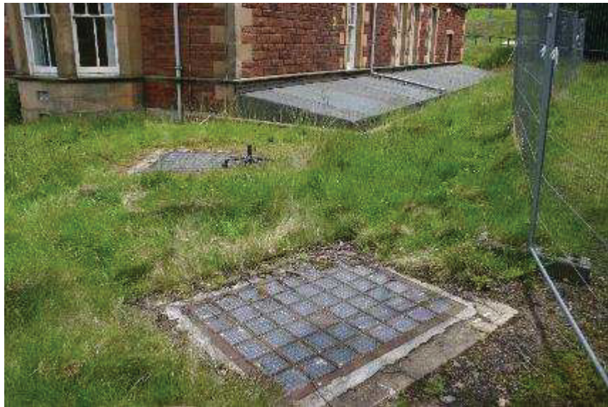
Plate 27: Skylights of tunnel
