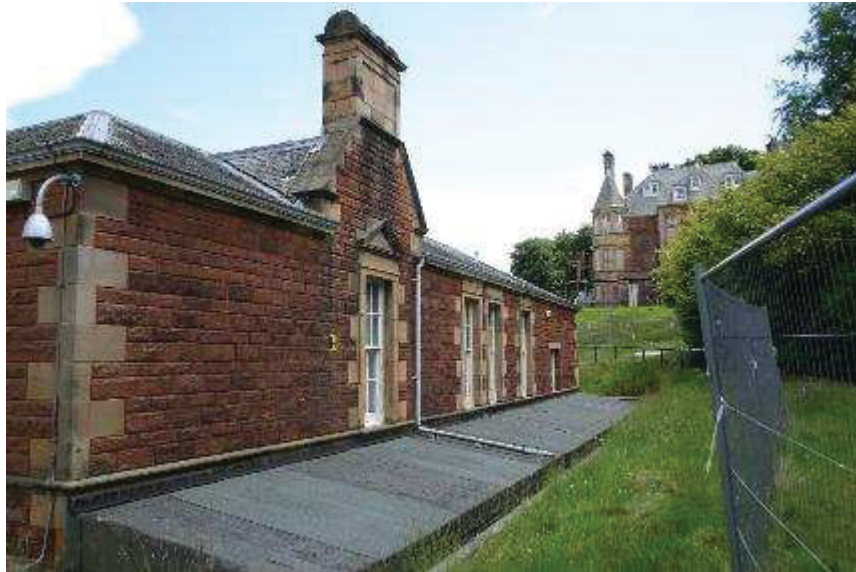
Plate 6: West Elevation, with tunnel
