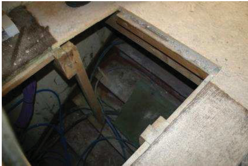
Plate 17: Detail stairs to tunnel
