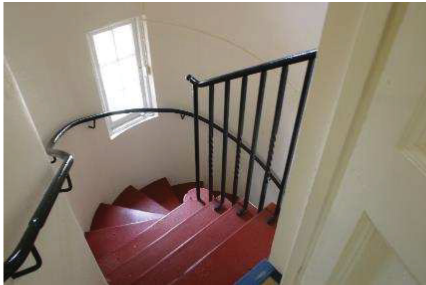
Plate 23: Detail newel staircase R7 to lower ground floor R 26
