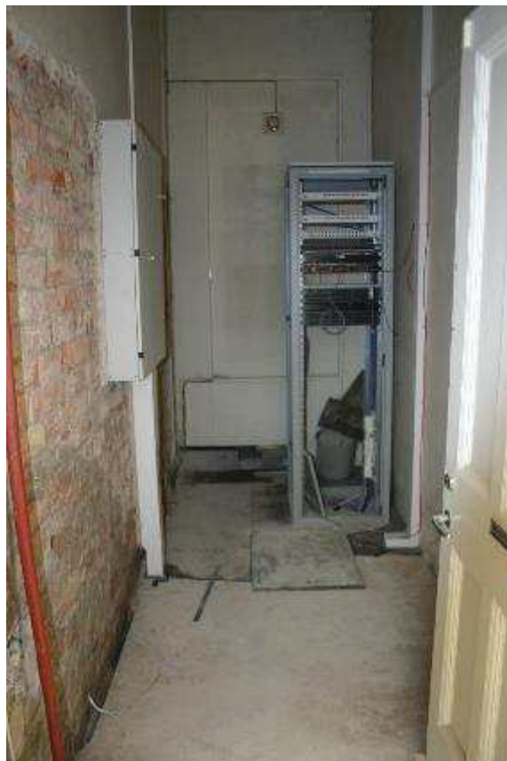
Plate 16: R 15, entrance to tunnel
