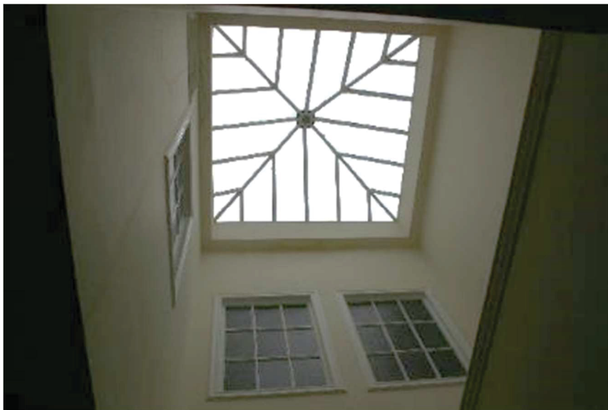
Plate 129: R 208, detail light well
