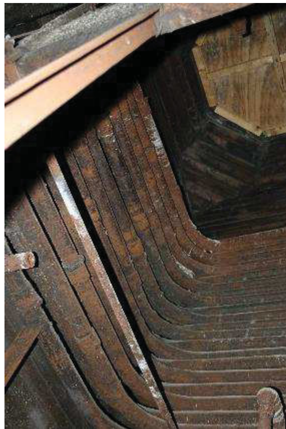
Plate 179: R 366, water or gas pipes in timber lined service shaft
