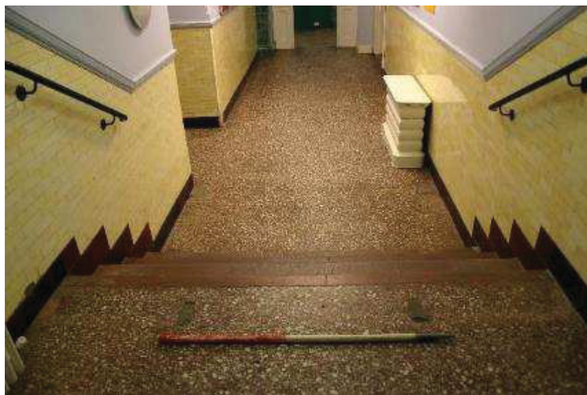
Plate 66: R 55, traces of handrail
