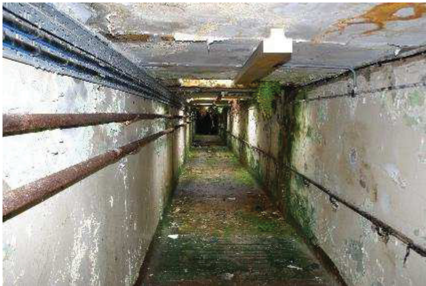
Plate 185: Tunnel between Bevan, East and New Craig
