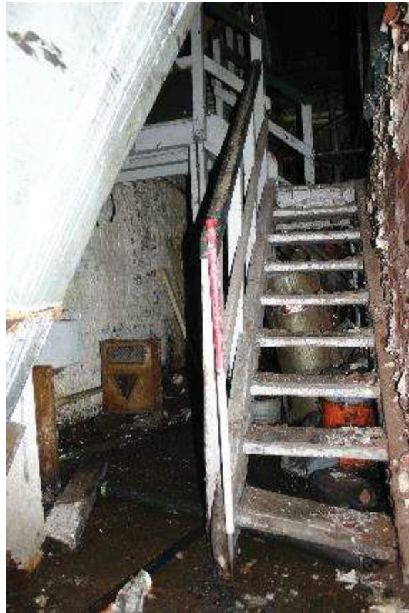
Plate 182: Engineers Pavilion, timber staircase
