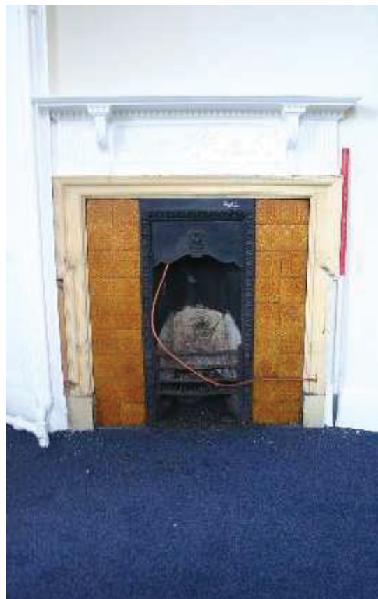
Plate 159: R 278, newly opened chimneypiece
