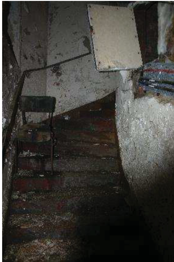
Plate 188: Entrance to Bevan House
