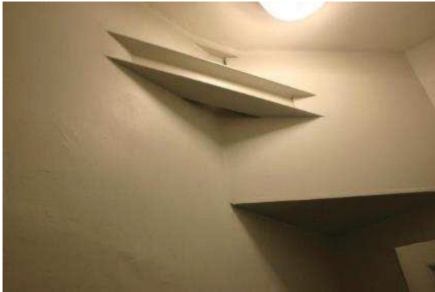
Plate 124: R 200, detail of steel beam
