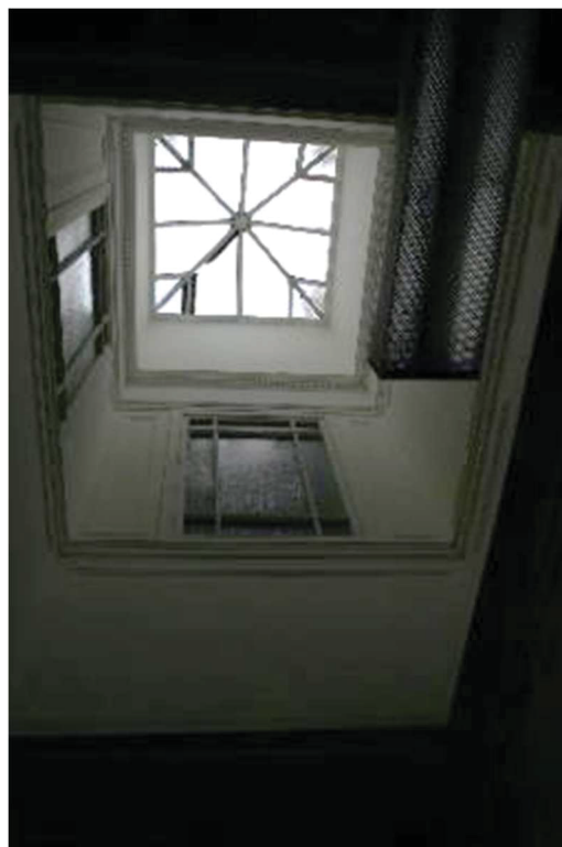
Plate 175: R 328, detail of light well
