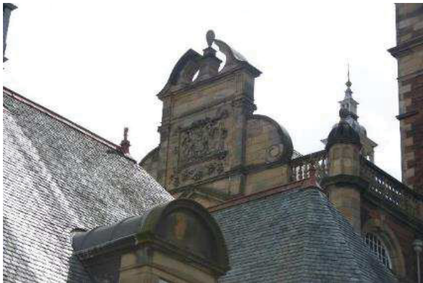
Plate 24: Detail of coat of arms north elevation Main Building
