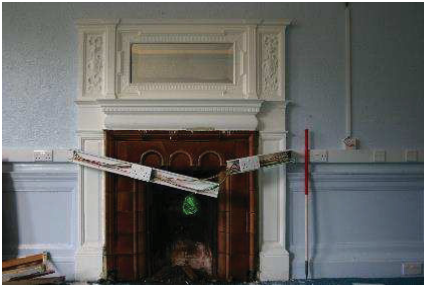
Plate 111: R 162, newly opened chimneypiece
