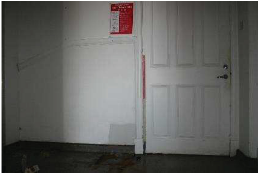
Plate 86: R 104, remains of staircase
