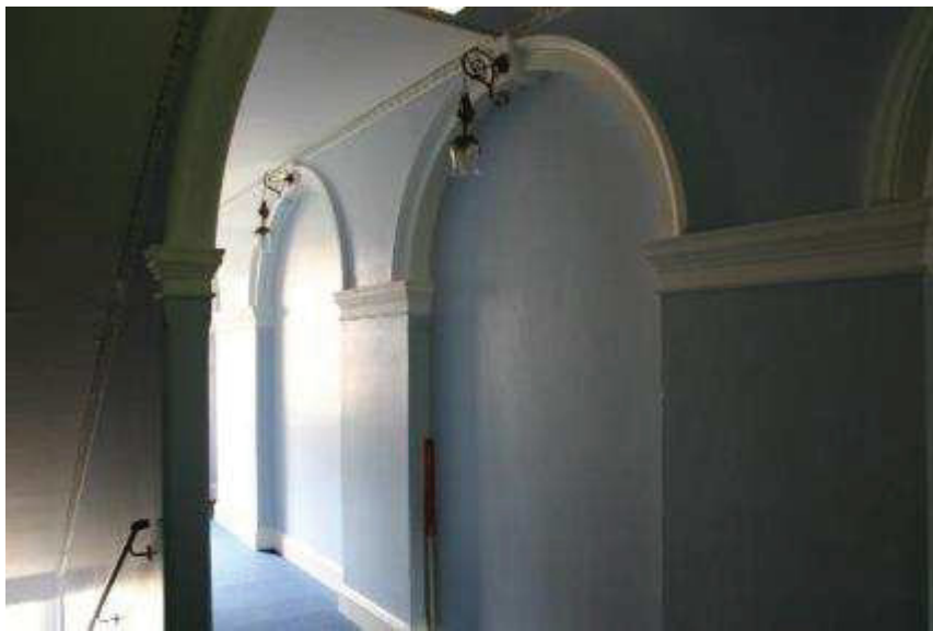
Plate 127: R 205, blocked gallery
