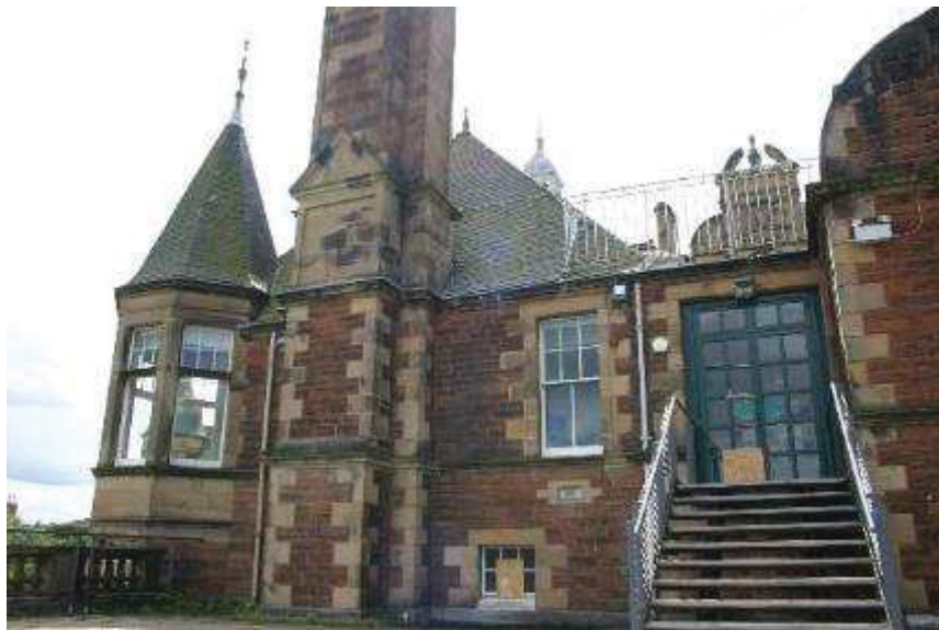
Plate 23: North elevation Main Building
