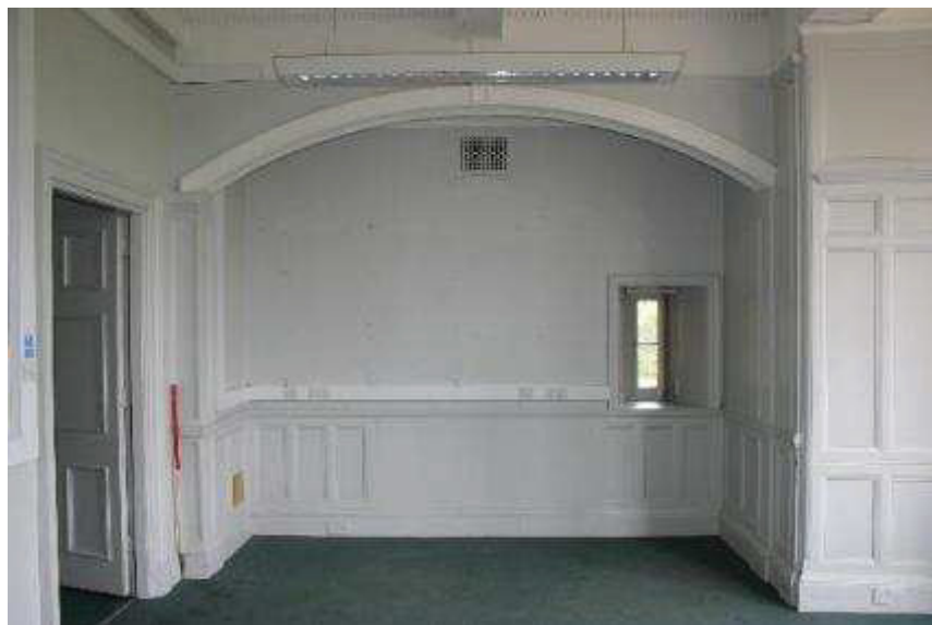
Plate 56: R 33, alcove with removed chimneypiece
