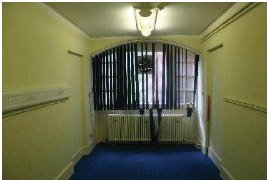
Plate 93: R 117, blocked doorway
