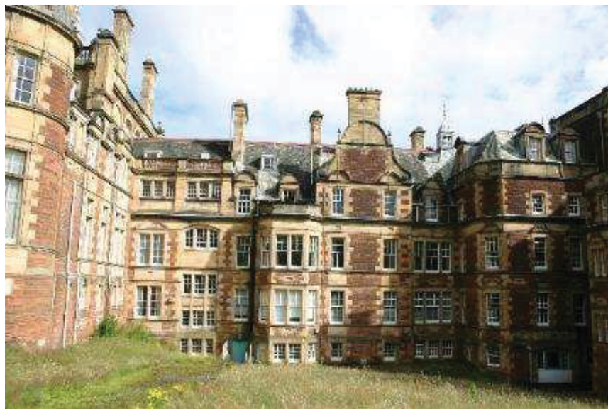
Plate 6: South elevation in the middle of the East Wing
