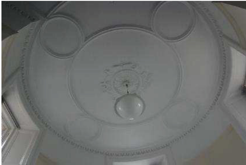
Plate 104: R 144, detail ceiling at circular bay
