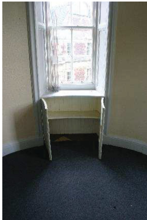
Plate 131: R 211, built in cupboard
