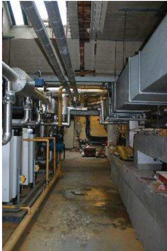
Plate 180: R 367, Boiler House
