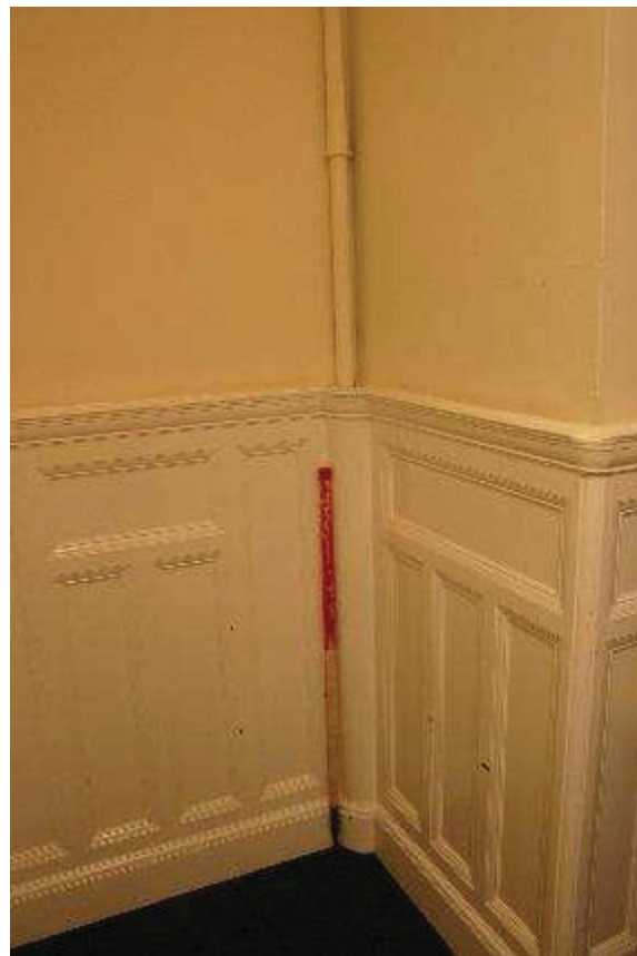
Plate 138: R 233, detail panelling (1 metre scale)
