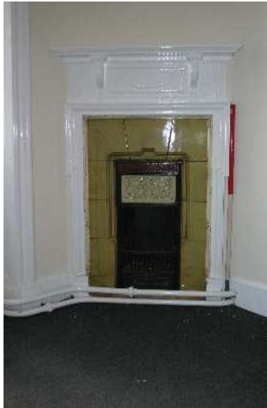
Plate 132: R 213, newly opened chimneypiece
