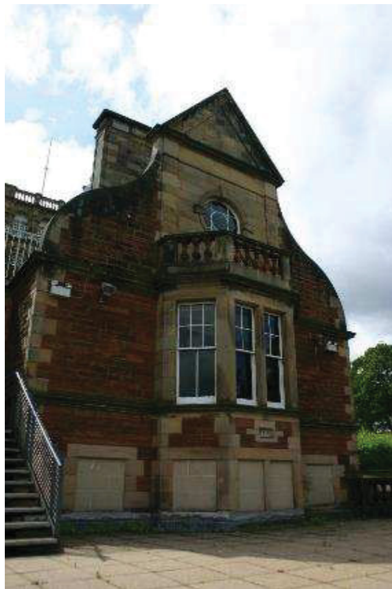
Plate 22: North elevation Main Building
