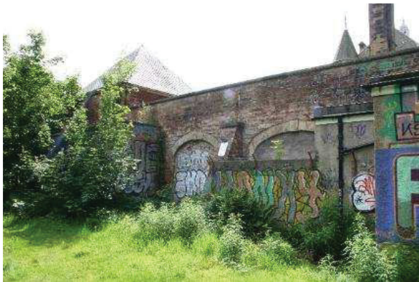
Plate 28: North elevation with modern extensions to Engineers Pavilion
