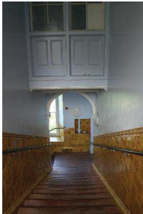
Plate 151: R 256, general view, detail: glazed corridor
