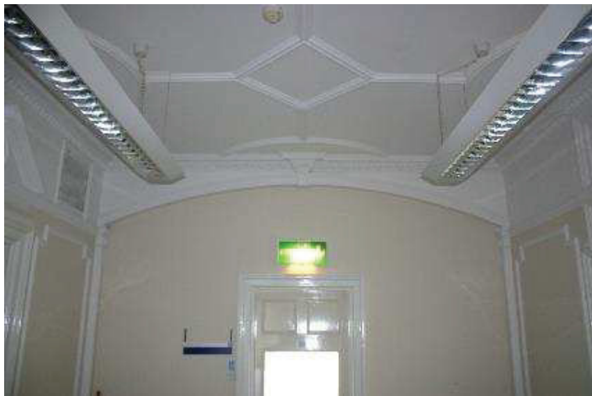
Plate 137: R 231, blocked arch
