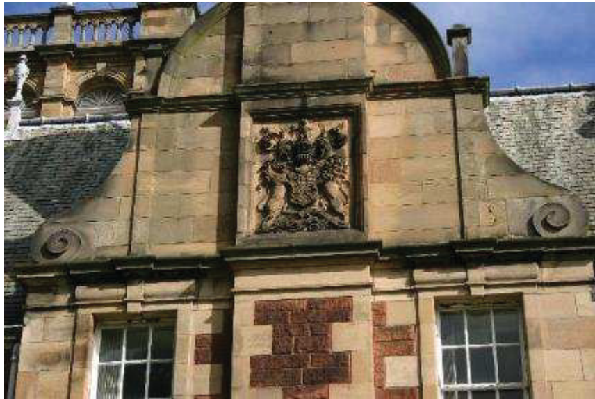
Plate 9: Detail from the south elevation of the Main Building
