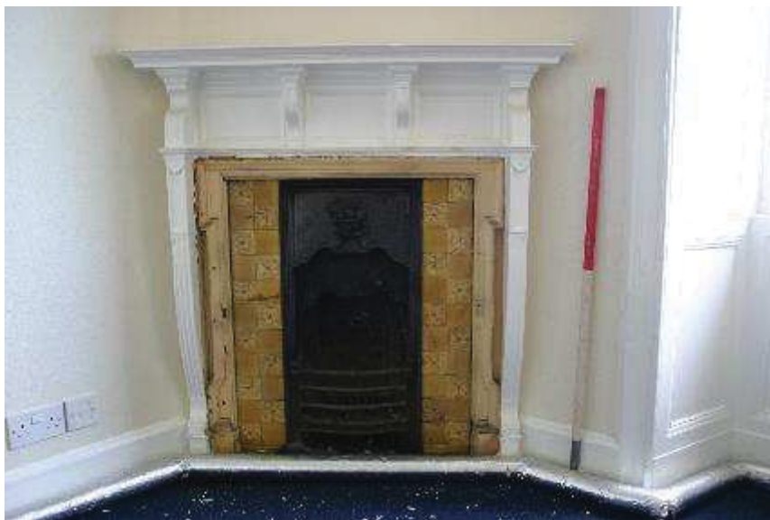
Plate 147: R 250, newly opened chimneypiece
