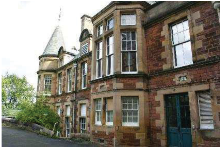
Plate 21: West elevation Main Building
