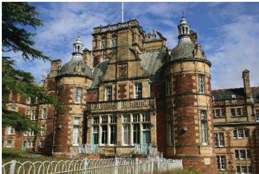
Plate 8: South elevation of the Main Building
