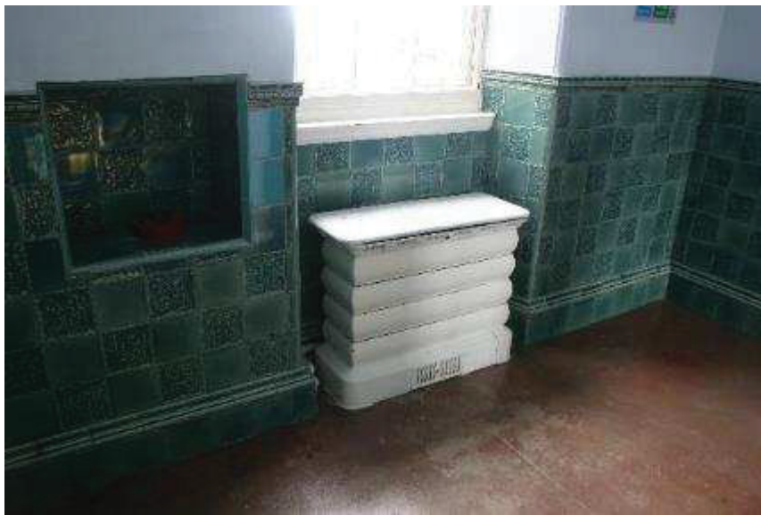
Plate 123: R 197, detail of Victorian radiator and cover
