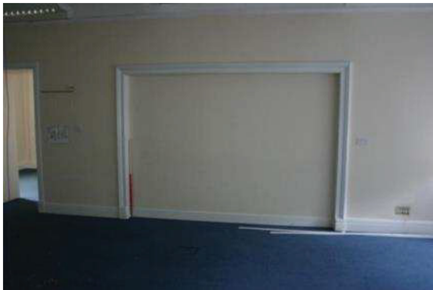
Plate 42: R 9, blocked double doorway
