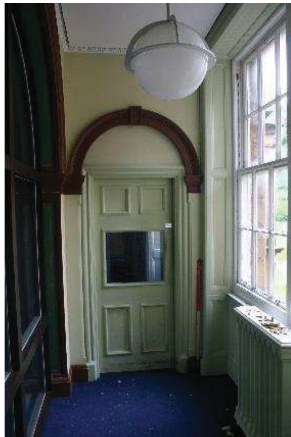
Plate 133: R 217, general view with Victorian radiator
