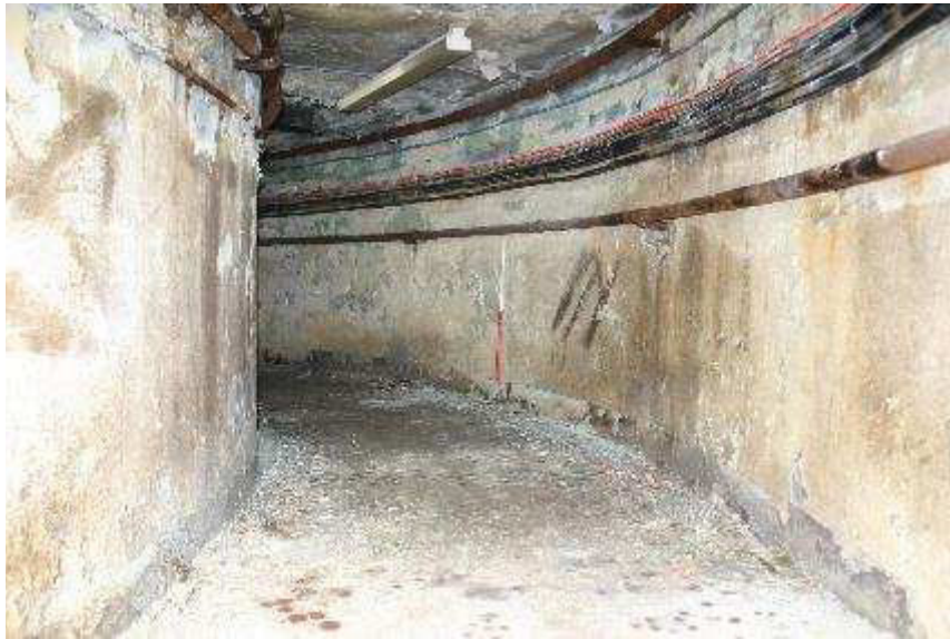
Plate 186: Tunnel between Bevan, East and New Craig
