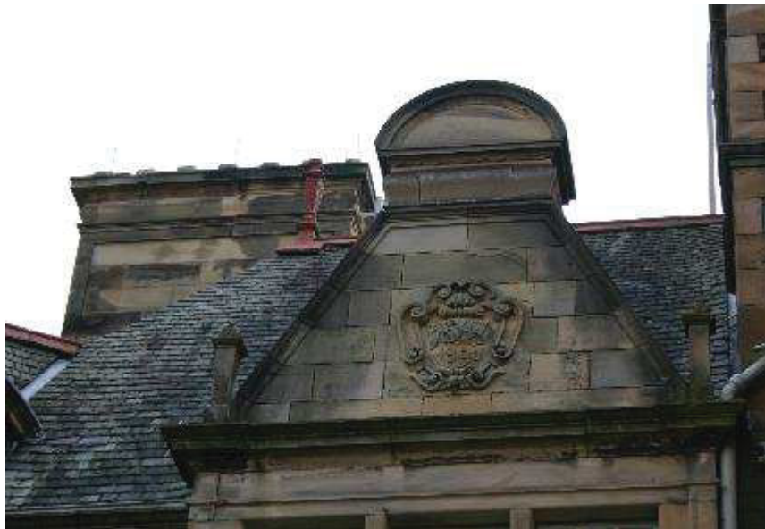
Plate 18: Detail south elevation West Wing
