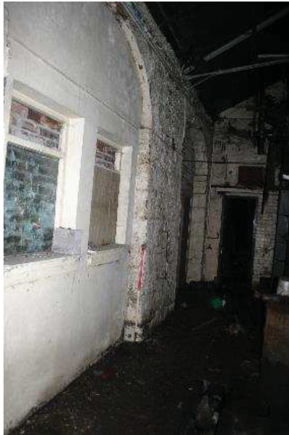
Plate 184: Engineers Pavilion, blocked arches
