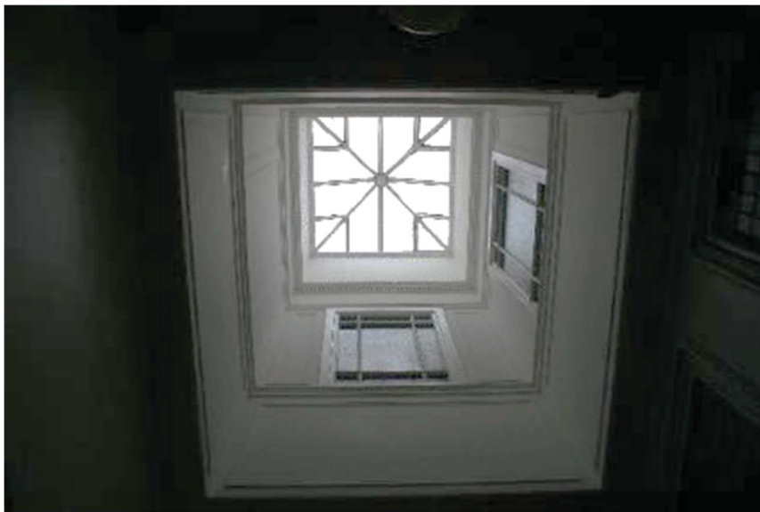
Plate 121: R 176, detail of light well
