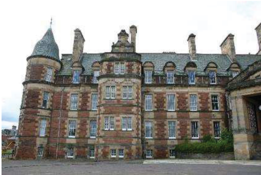
Plate 7: North elevation East Wing
