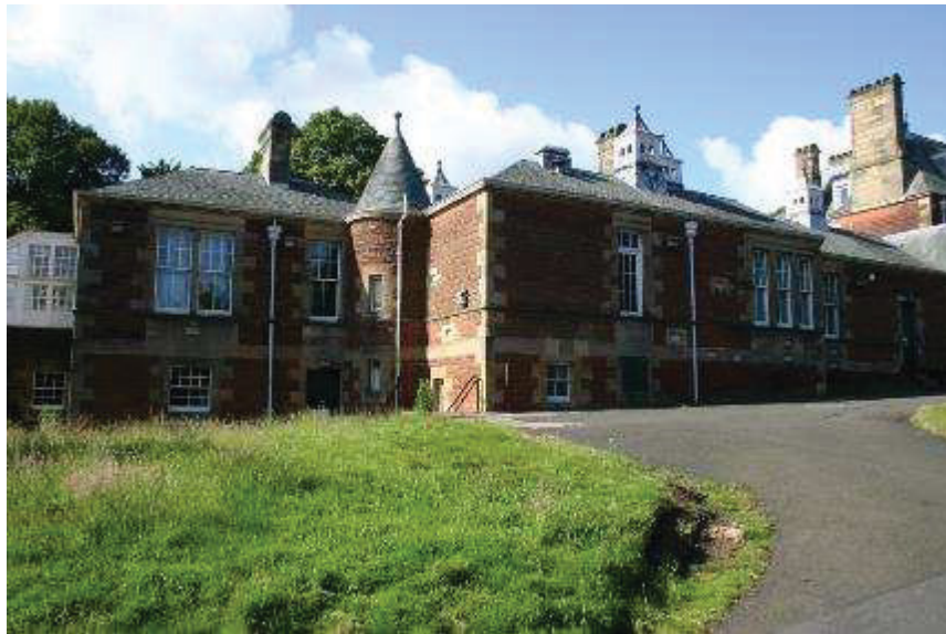
Plate 5: north elevation, east part
