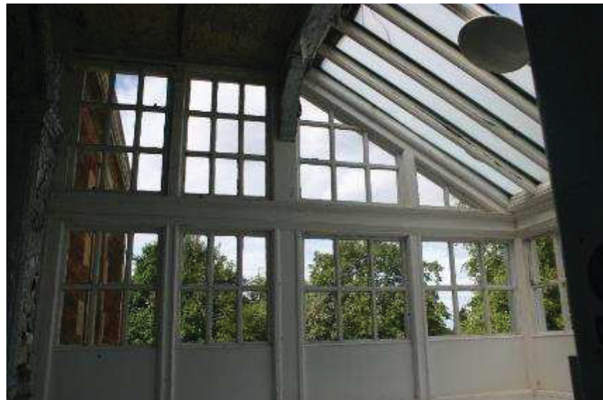
Plate 30: glazed timber conservatory R 36
