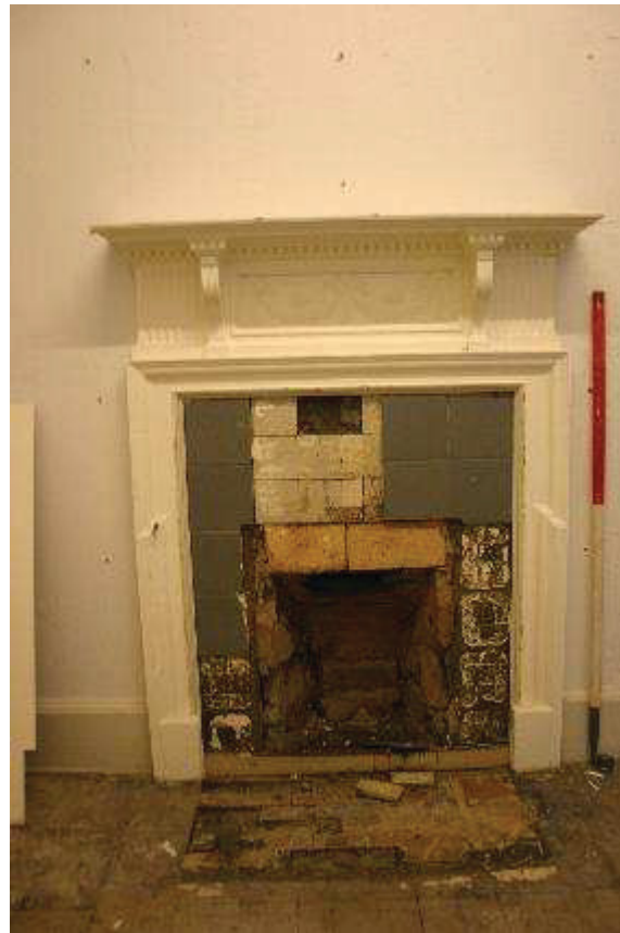
Plate 35: R 54, chimneypiece with several layers of tiles
