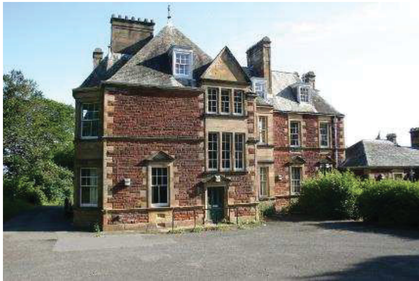
Plate 1: south elevation, west part
