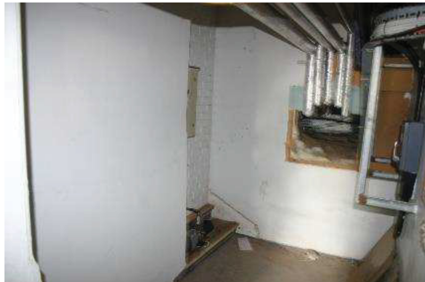
Plate 46: Blocked staircase to R 14 in R 76
