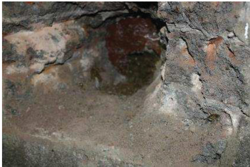
Plate 48: Blocked and filled tunnel entrance at Queens Craig
