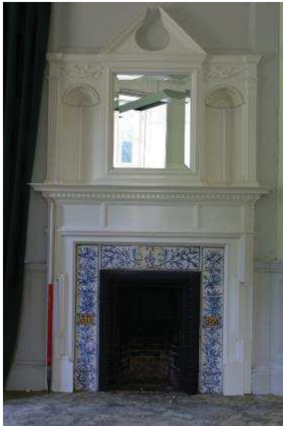
Plate 12: chimney piece with date A.D. 1894 in R 3
