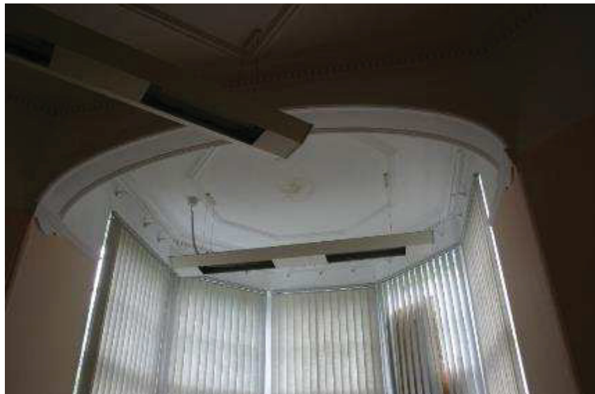
Plate 34: octagonal bay with three centred arch in R 42
