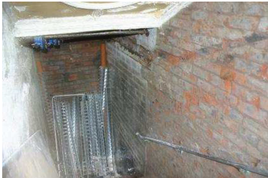
Plate 40: removed plaster and blocked tunnel entrance in R 64
