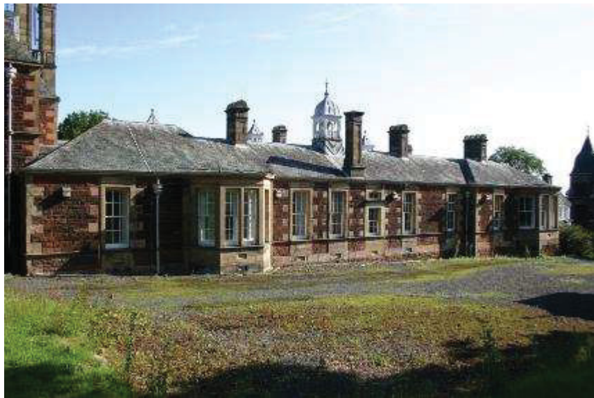
Plate 2: south elevation, east part
