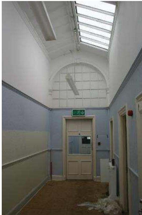
Plate 23: partition wall between 20 and 24, upper part possibly original, painted over
