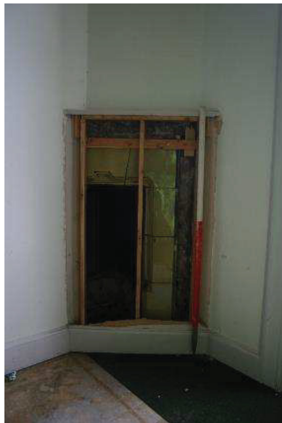
Plate 16: half built over, reopened chimneypiece in R 12
