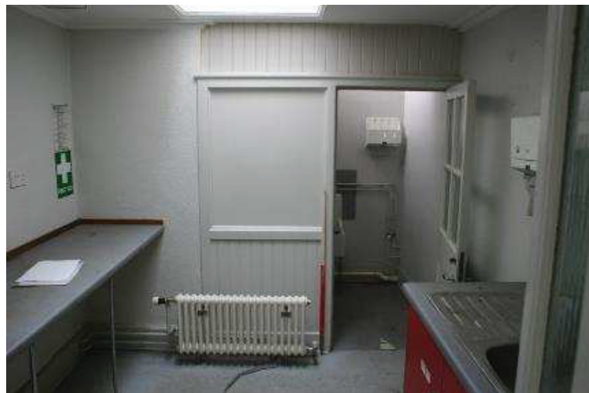
Plate 38: timber partition wall in R 59
