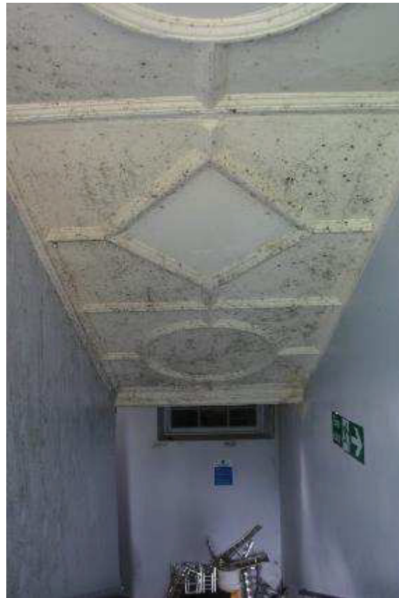
Plate 41: mould infestation in R 64
