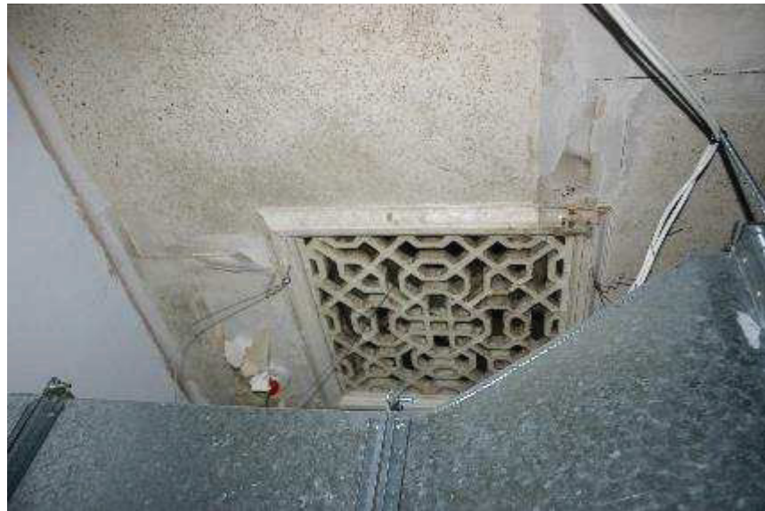
Plate 27: R 32, ceiling toilet room
