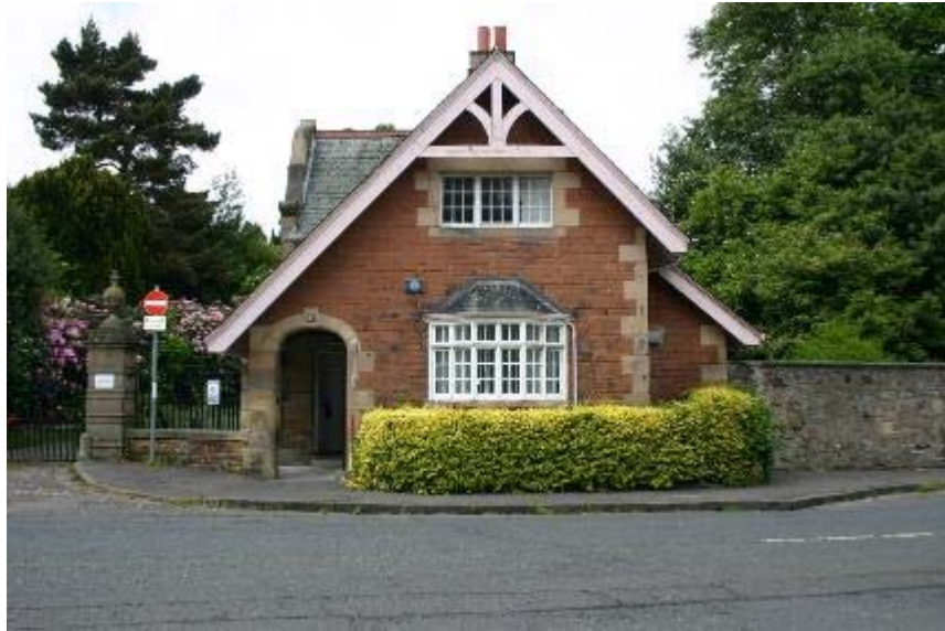
Plate 1: Front, east elevation.
