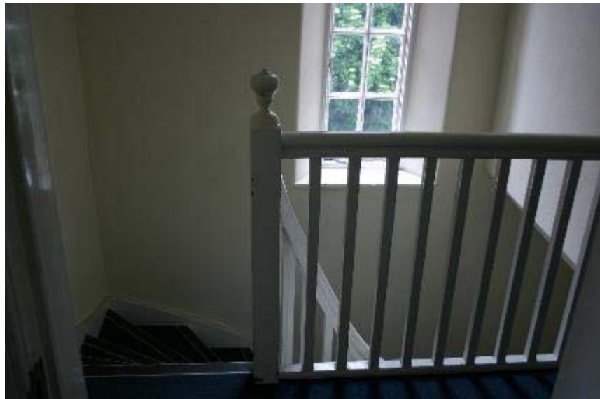
Plate 12: balustrade of timber staircase.
