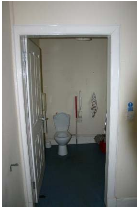
Plate 11: Toilet room, ground floor.
