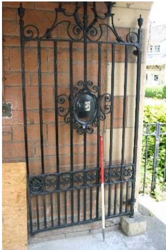
Plate 2: Detail, wrought iron pathway gate.
