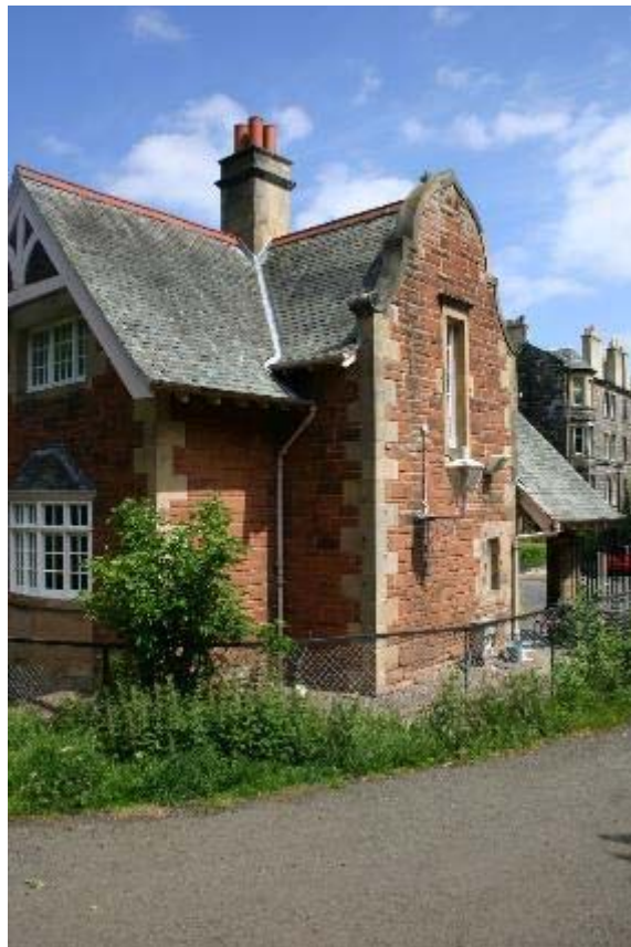
Plate 4: oblique south elevation.
