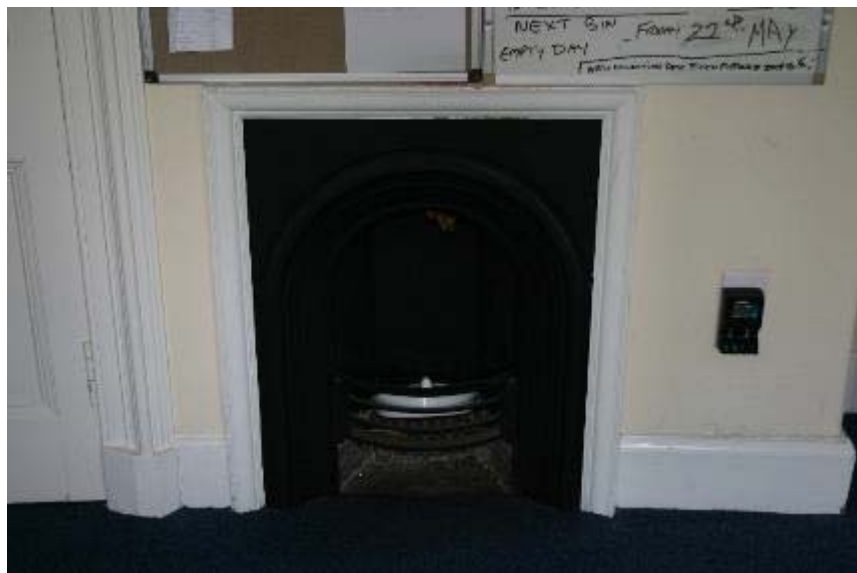
Plate 16: Cast iron fireplace R 5.
