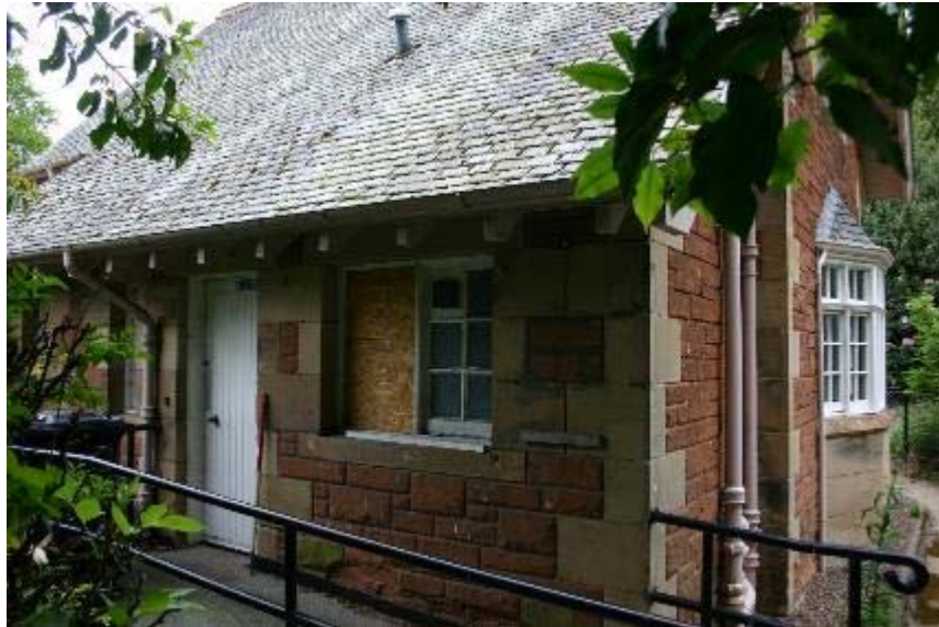
Plate 3: oblique north elevation.
